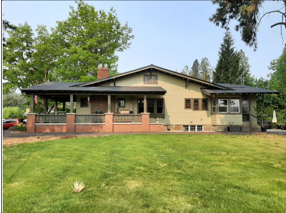
Photo 7 Looking west at the east elevation of the house in 2023
