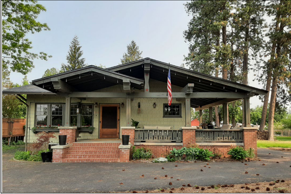
Photo 1 The south façade of the Arthur & Florence Davis House in 2023, looking north
