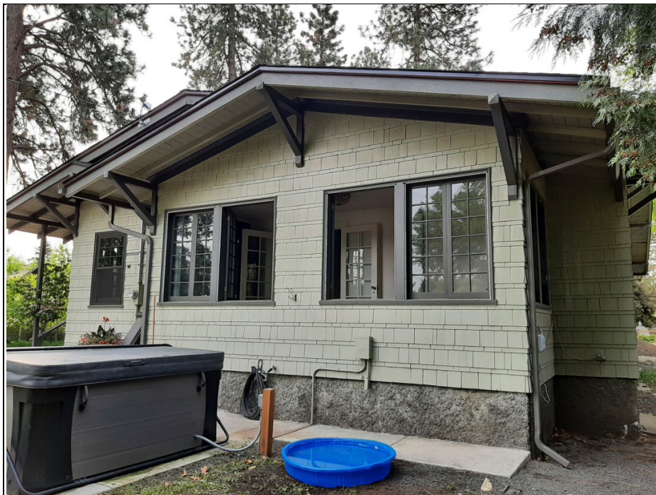
Photo 8 Looking at the north rear elevation of the house in 2023
