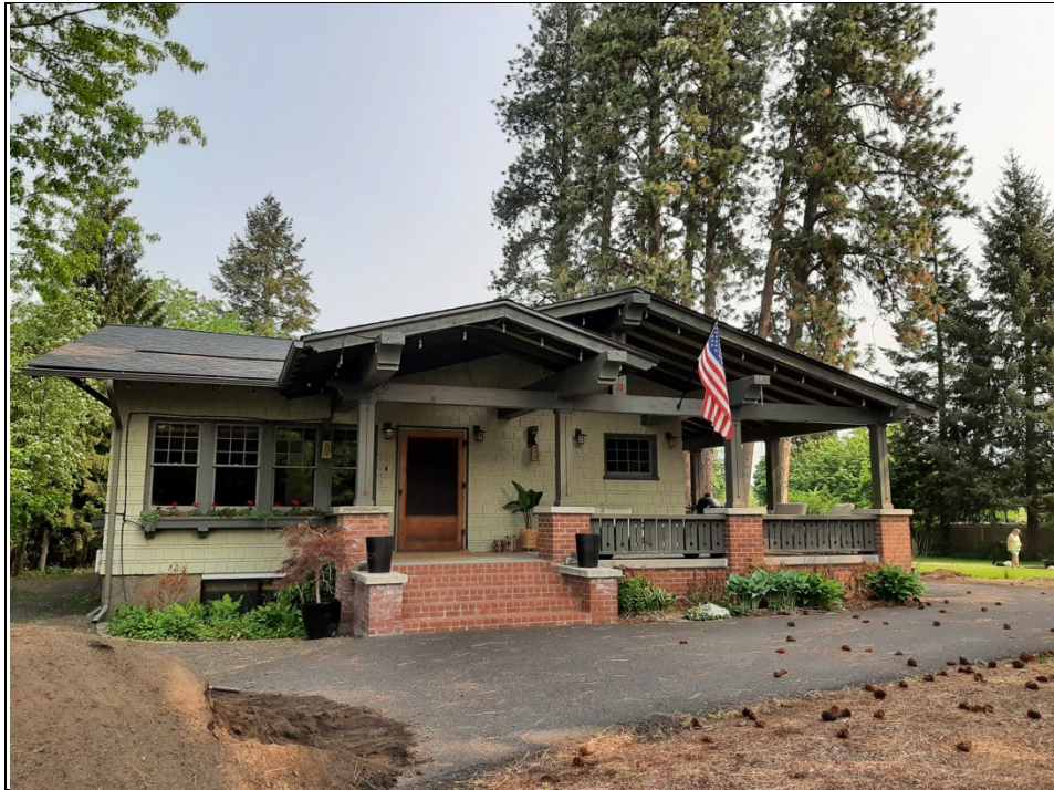
Photo 3 The south façade of the Davis House, looking north in 2023
