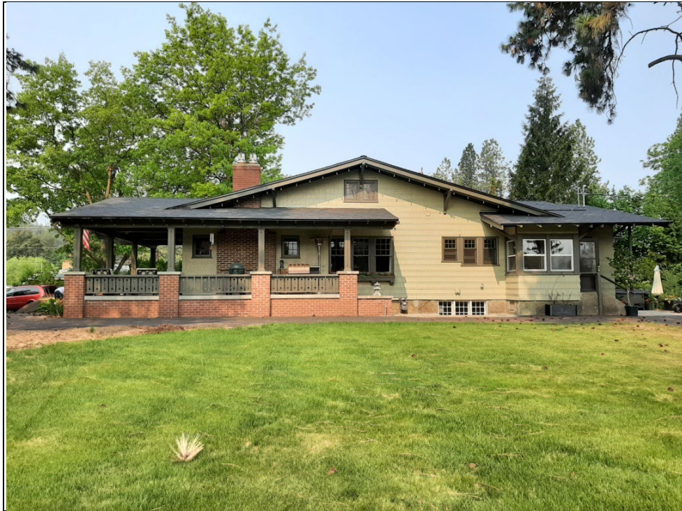
A 2023 photograph of the east elevation of the Davis House, looking west
