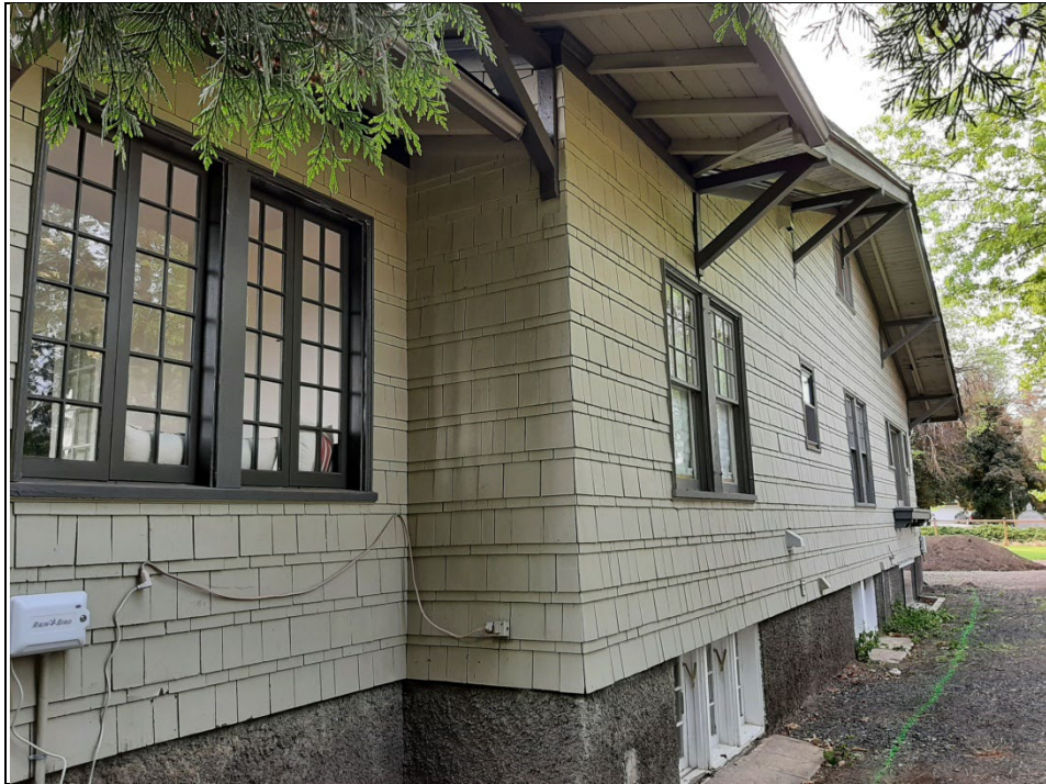
Photo 9 Looking south alongside the west elevation of the house in 2023
