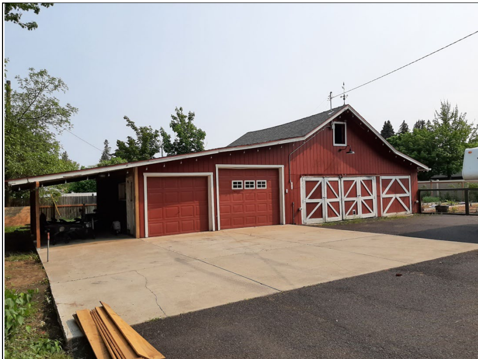
Photo 10 Looking north in 2023 at a barn that covers a carport, garage, shop, and storage
