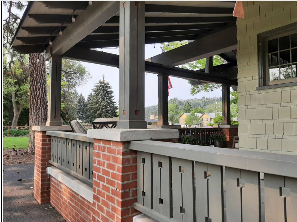
Photo 5 Looking south through the southeast corner of the front porch in 2023
