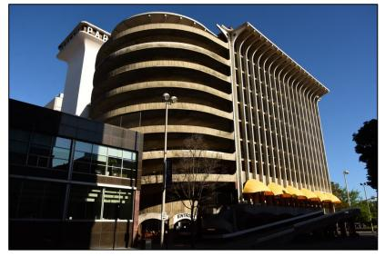
Poured in place, the ramp is finished with a raw, board-pressed concrete finish. Eight levels running between floors three and ten are displayed in eight arch segments as the final level joins the secondfloor exit level. On the west face, the ramp segments run between the eighth and second floors; the
