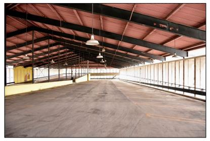
The open sides display the graceful arches of the cornice brackets in which 2-footdiameter round holes are centered within the spandrels of the arches. Elevated slightly above the cornice ledge are concrete bases upon which the steel I-beams of the roof structure are anchored. The lateral cross beams are supported by every fourth column, as are the smaller beams supporting the ends of the hipped roof
