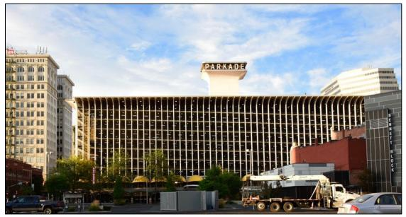
skywalk. Corresponding to the ground floor arched bays, the 52 concrete columns dividing the arched bays of the ground floor are aligned with every fourth column extending upwards from the second story level.
