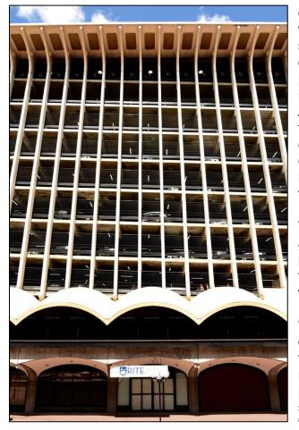
discerned on the south façade as well as the north façade. On the south façade, the edges of the floor decks, the guard rails—steel planks and steel cables, are visible in their upward slope to the west. As described above, the building is terminated with flared precast cavetto brackets supporting a concrete cornice ledge. The hipped roof is set back and only visible from a distance.
