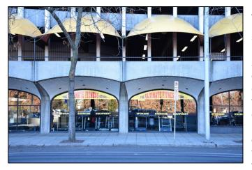
All the bays are configured identically with a vertical 24-inch square concrete column with a bush hammered finish, spaced about 17'-10" on center. The bay opening is 16 feet between columns and 50 feet from grade to top or arch. The square columns extend from sidewalk grade to the point at which the elliptical arches of the window bays intersect the vertical faces of the columns. At that point, the columns narrow and
