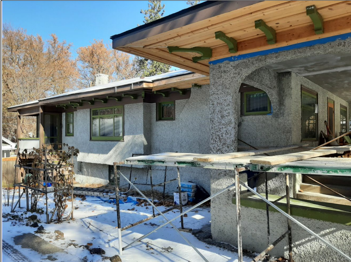
Looking east at the west elevation of the house in 2023
