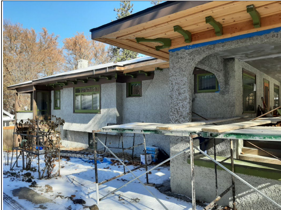
Photo 5 The west elevation of the Ritter House in 2023, looking east
