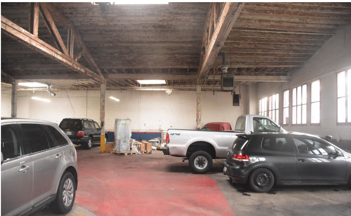
20. Garage, looking east along south wall
