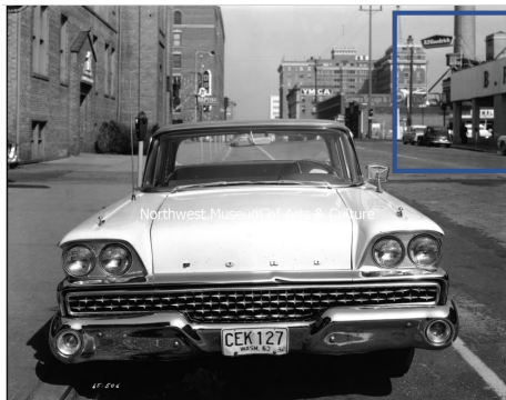
L87-1.506-65 NW MAC JEF Research Archives Libby Collection – 1965 photo showing the porte cochere corner of the Ahrens & Ahrens Building
