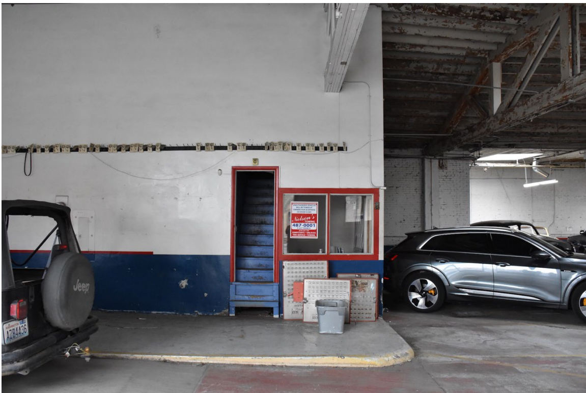
18. Garage office and stairs to mezzanine storage room, looking east
