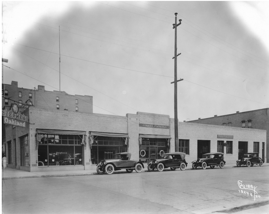
11. Ahrens & Ahrens in 1920 - west facade, looking southeast _ L87-1.18244-20
