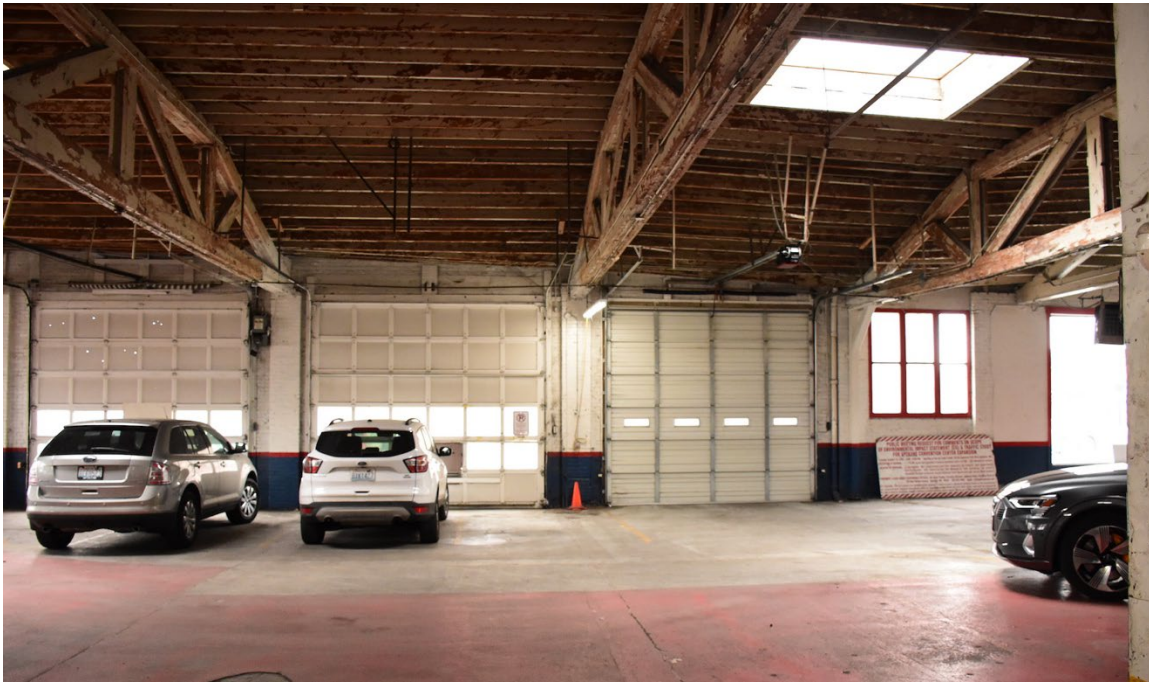
21. Garage, looking west toward west wall door bays
