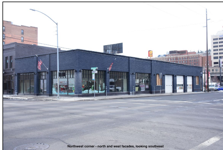
Northwest corner - north and west facades, looking southeast
