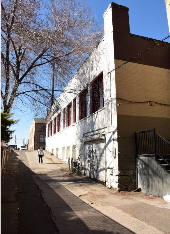
The rear southeast corner of the building where it extends behind the neighboring building to the east.
