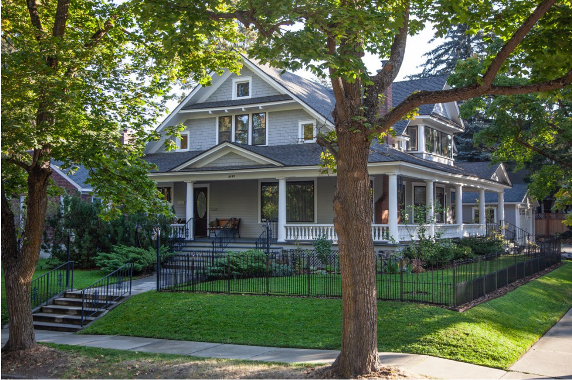
Photograph 1, October 2022: West and South façade.
