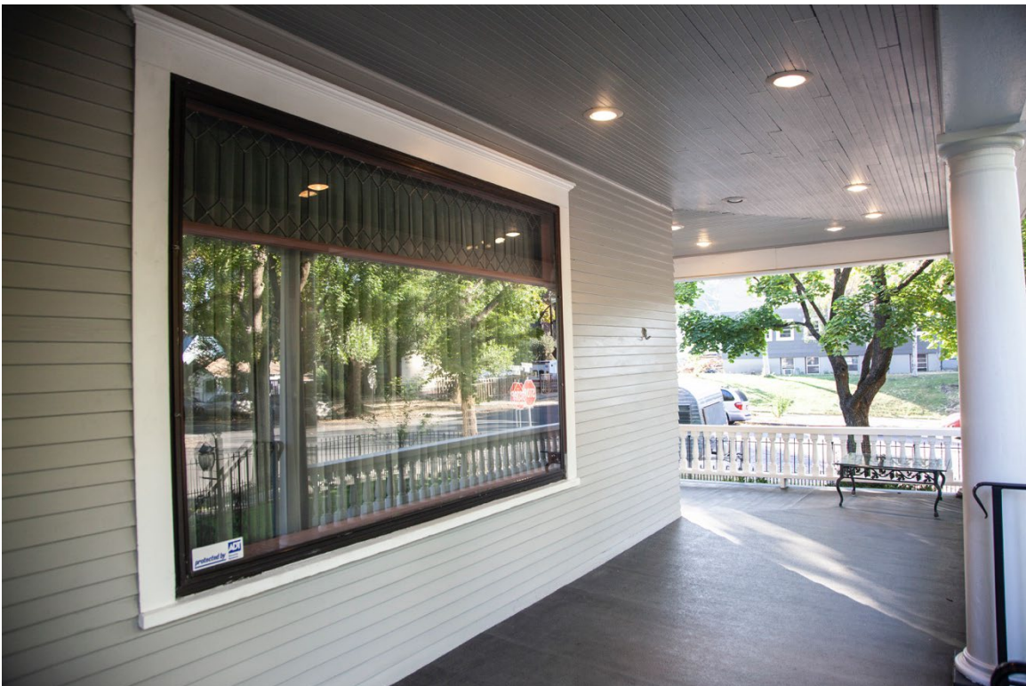
Photograph 8, October 2022: The large, fixed diamond-glass upper lights window on west, primary façade.
