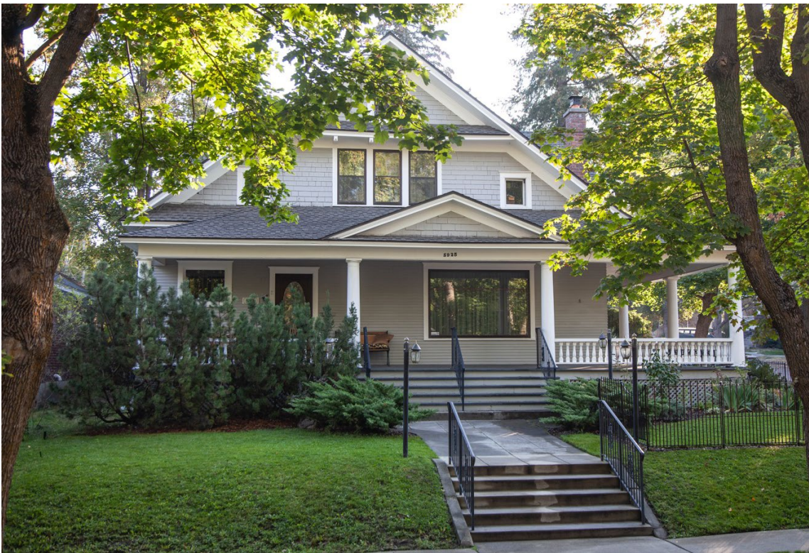
Photograph 2, October 2022: West, primary façade.
