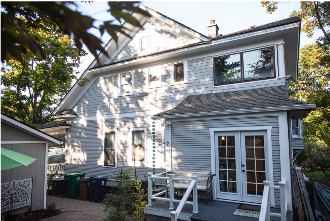
Photograph 6, October 2022: The back yard, east façade.
