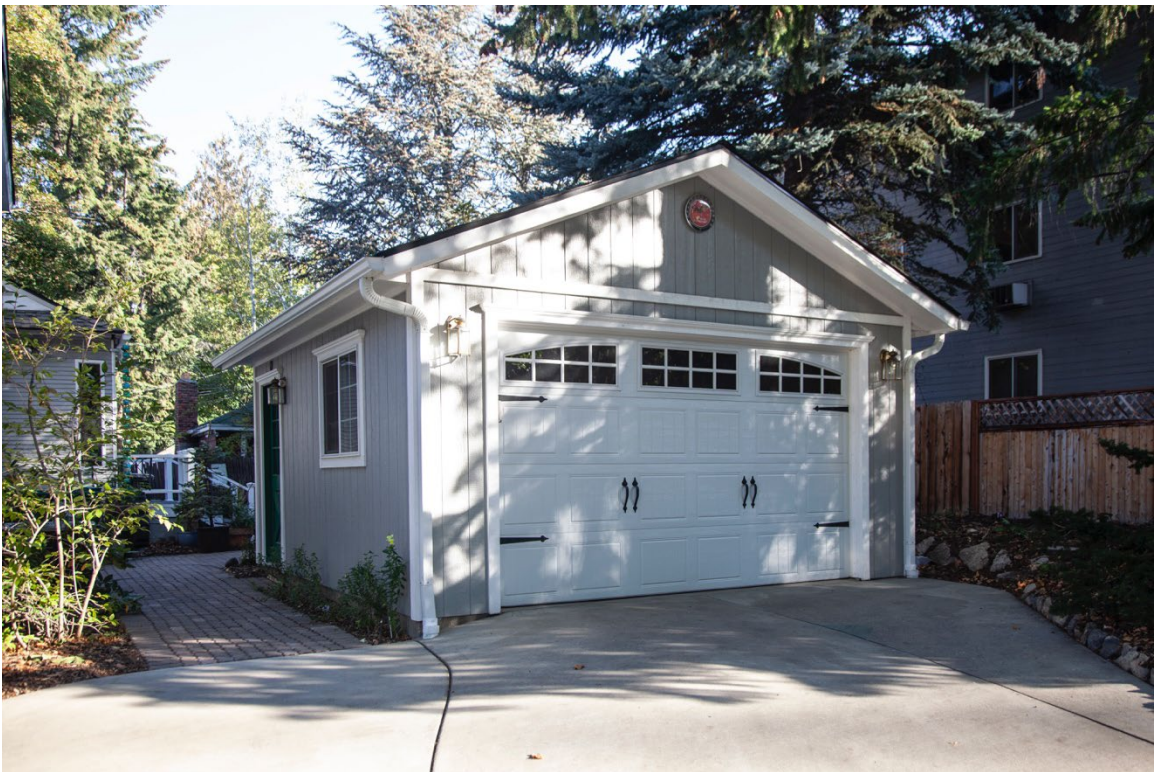
Photograph 4, October 2022: Garage, facing south.
