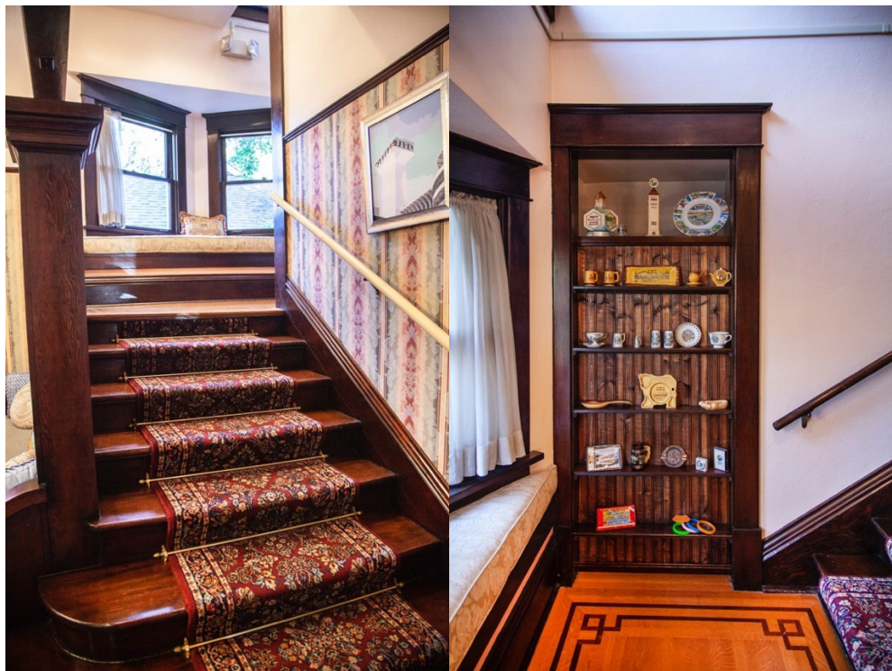
Photograph 12/13, October 2022: The staircase leading up to the landing, and the closed off doorway that connected the stairway to the kitchen.
