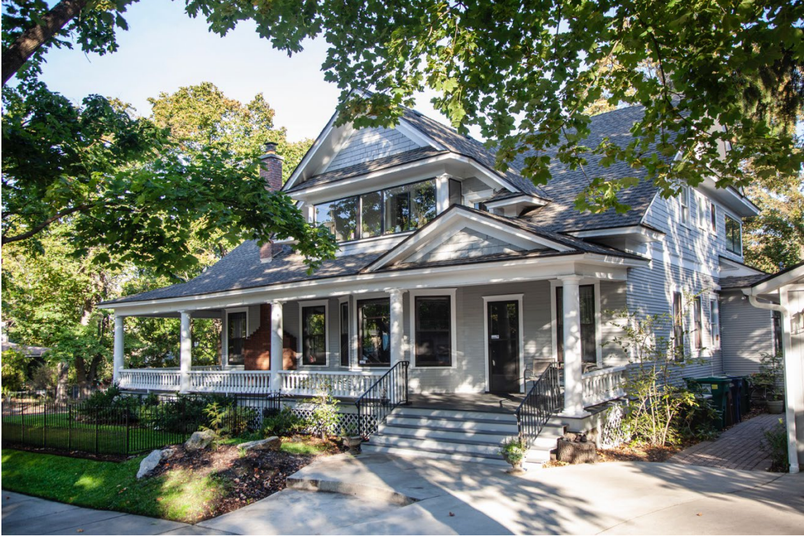
Photograph 3, October 2022: South façade.
