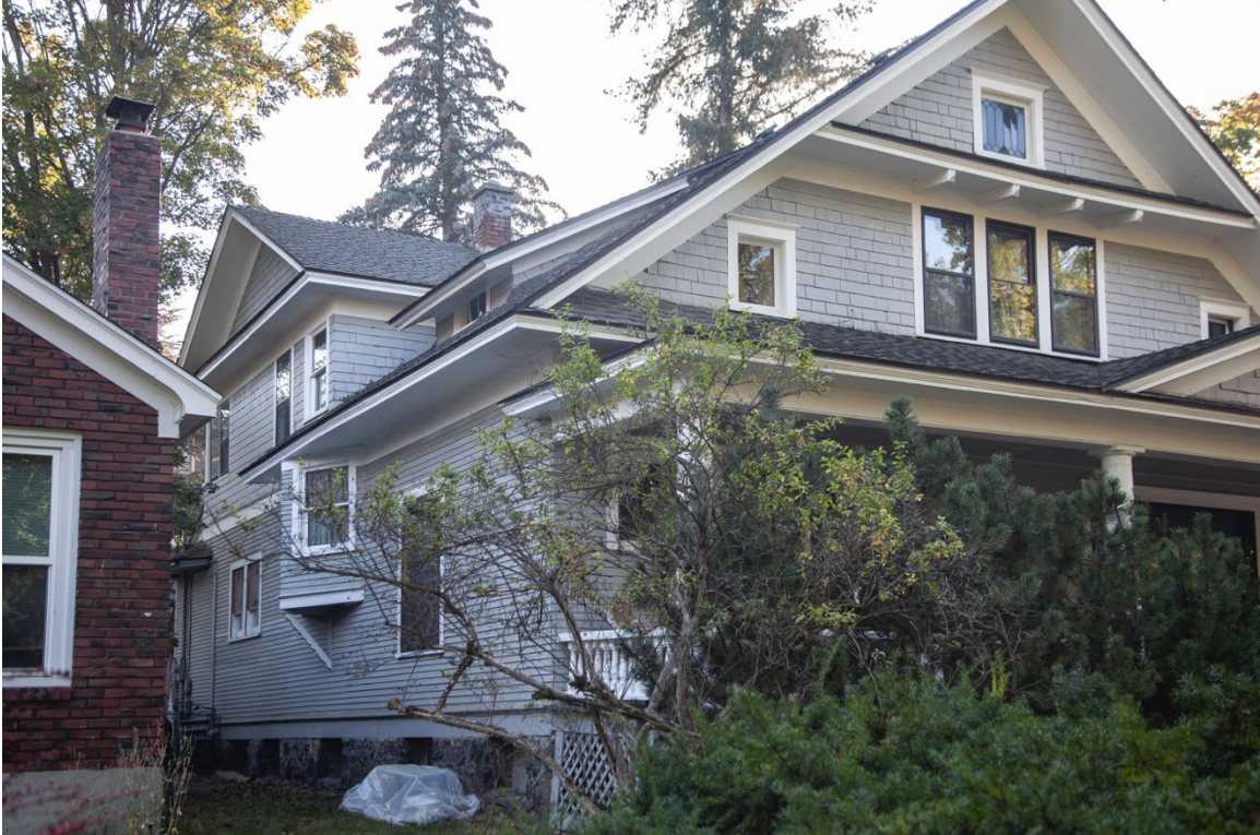
Photograph 5, October 2022: North and west façade.
