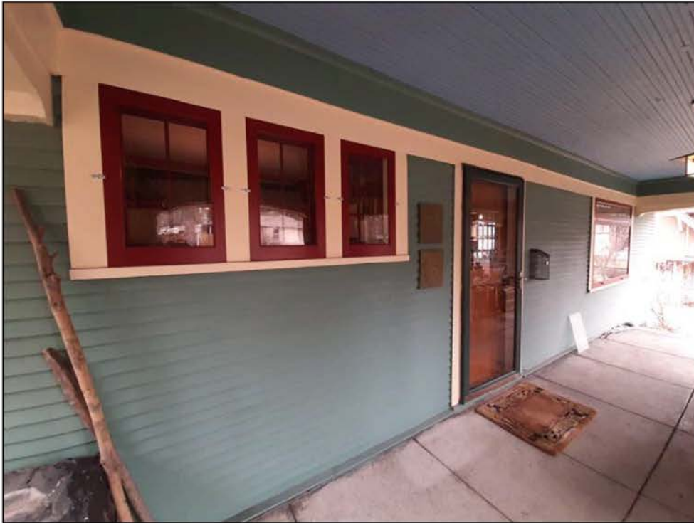
Photo 9—Covered front porch at east façade in 2021, looking northwest
