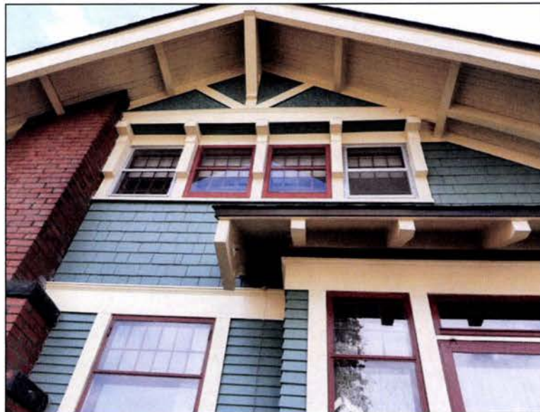
North elevation detail of the Eastman-Heritage House
