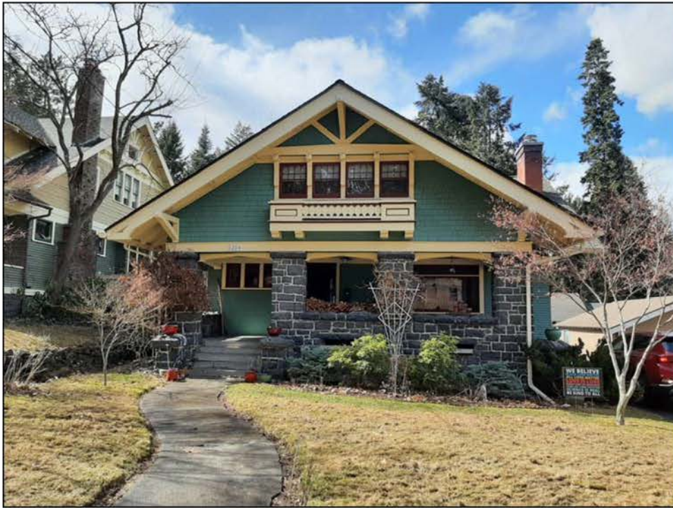
Photo 1—East façade of property in 2021, looking west
