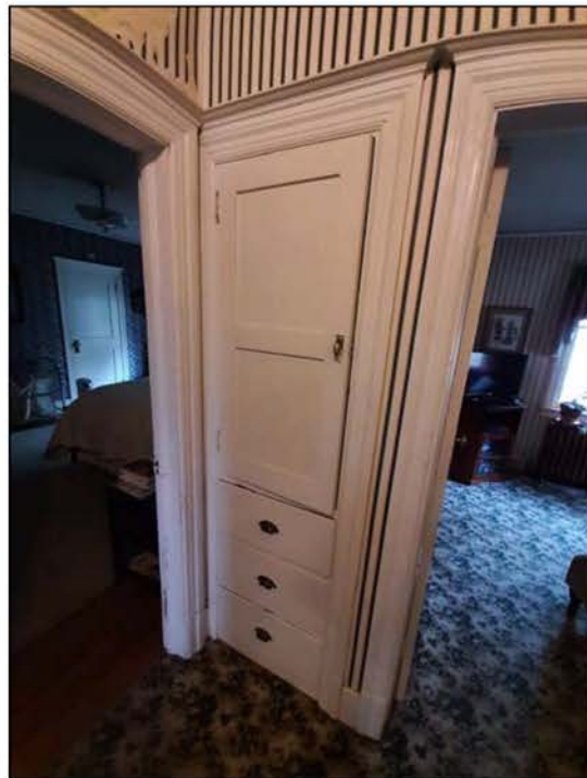
Photo 20—Built-in linen closet in first-floor hall in 2021
