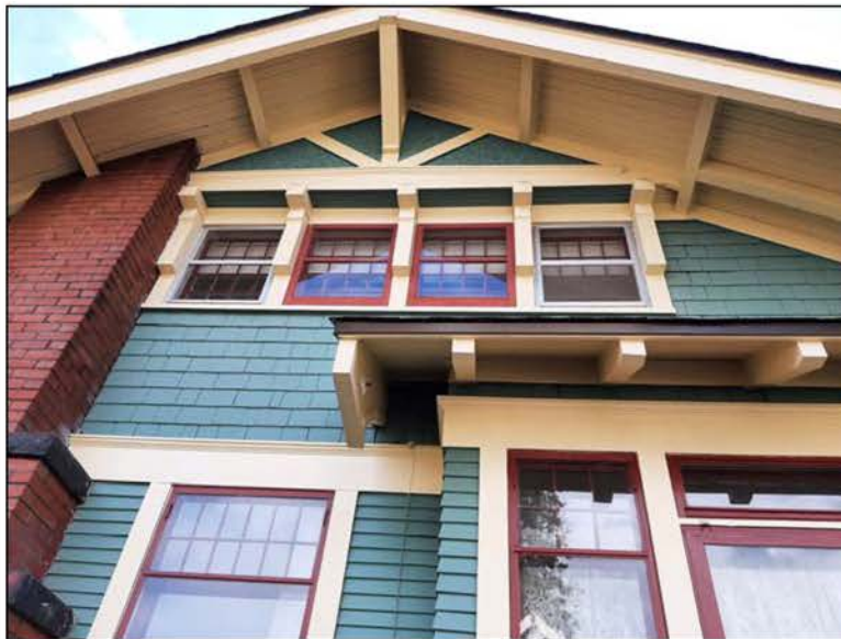
North elevation detail of the Eastman-Heritage House
