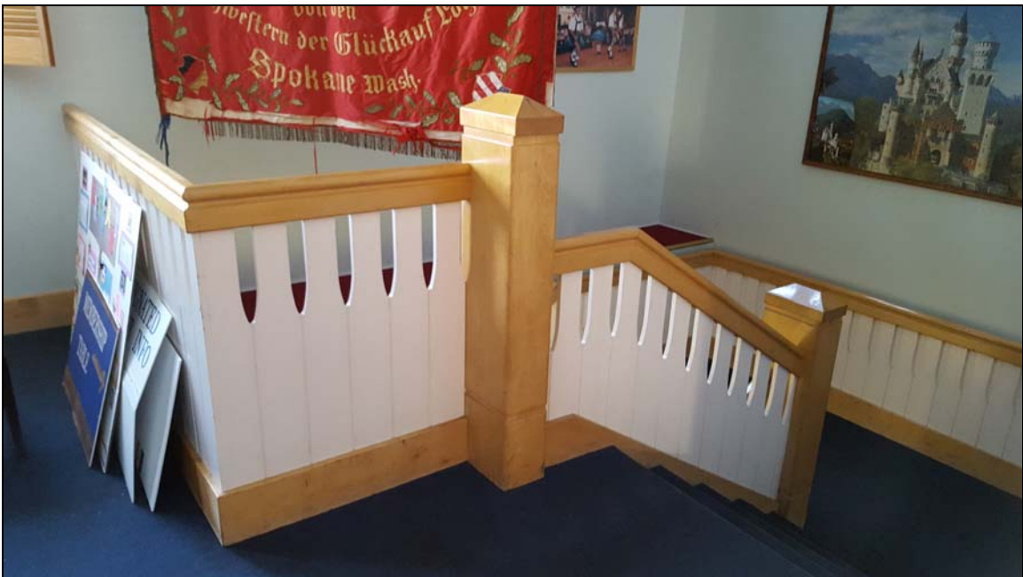
Photo 14 Looking at the front stairs on the second floor in 2018
