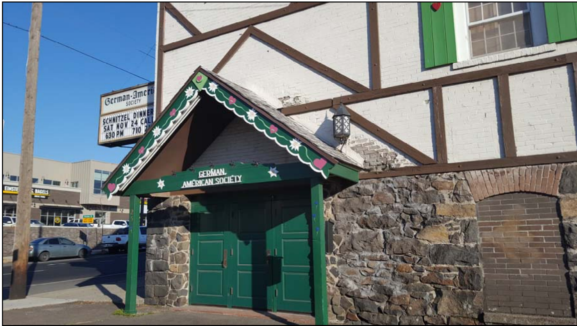
Photo 3 The front entrance to the building on the north end of the west face.
