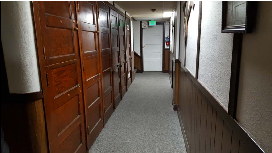
Photo 10 The basement north-south hallway, looking south in 2018.
