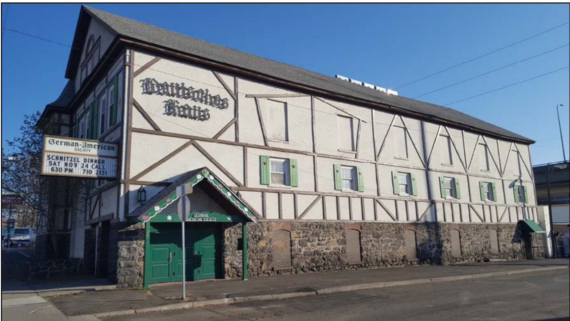
Photos 1 and 2 Views of the north façade and west face of the building in 2018
