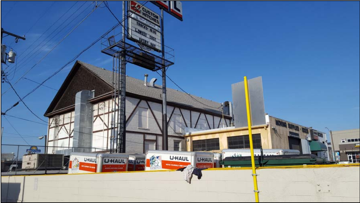
Photo 5 The southeast corner of the building, looking northwest in 2018.
