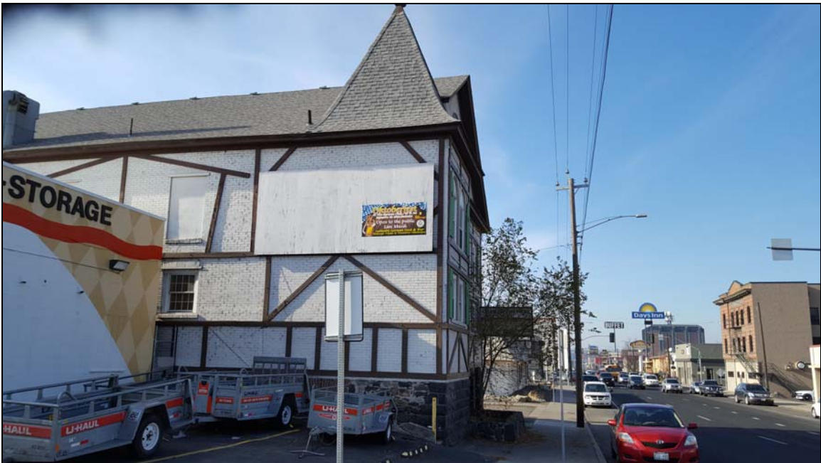
Photo 6 The east face of the building at the building's northeast corner, looking west in 2018.
