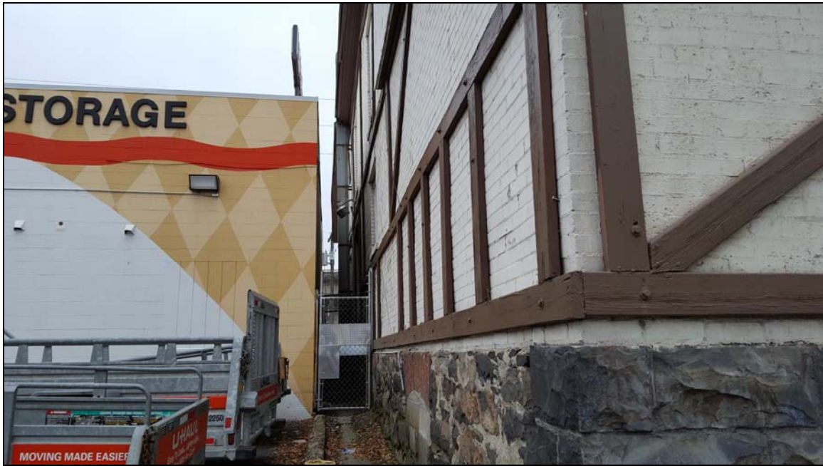
Photo 7 Looking south between two buildings from the northeast corner of the building along the east face in 2018.
