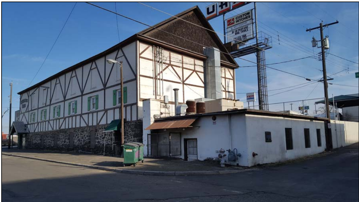
Photo 4 A view of the south face (gabled end) and west face of the building, looking northeast in 2018.
