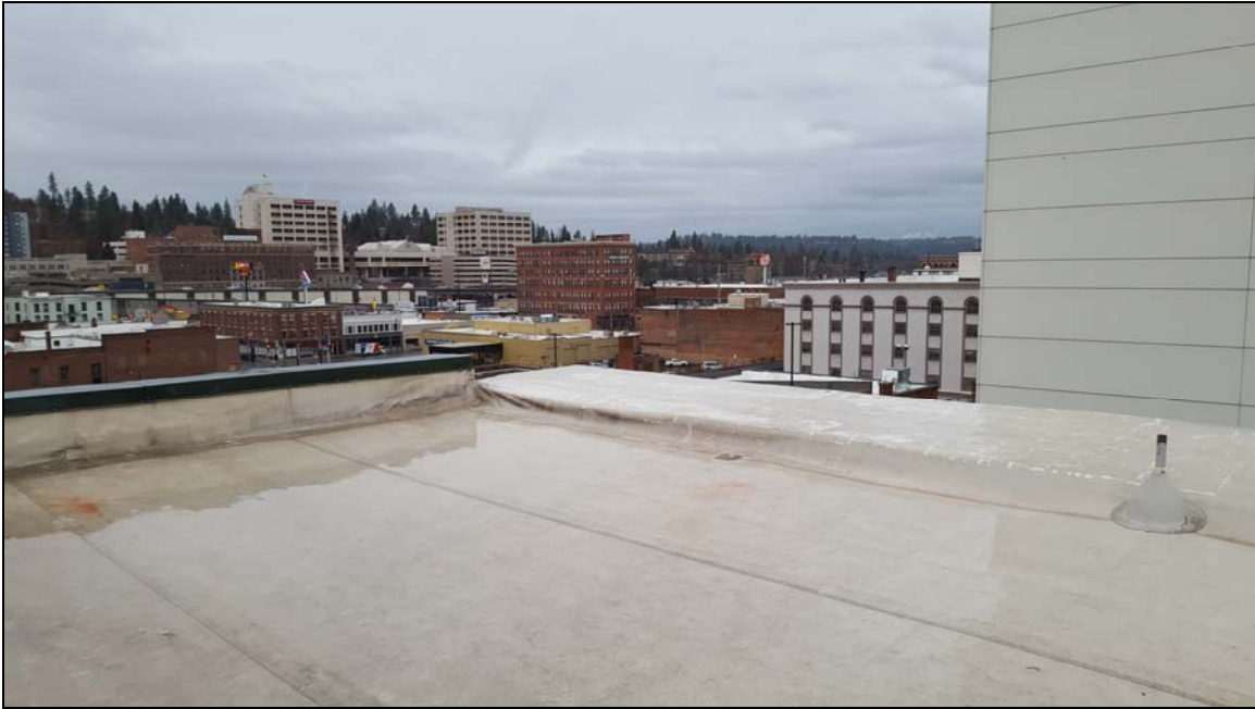
Roof of Columbia Building, looking southwest in 2019
