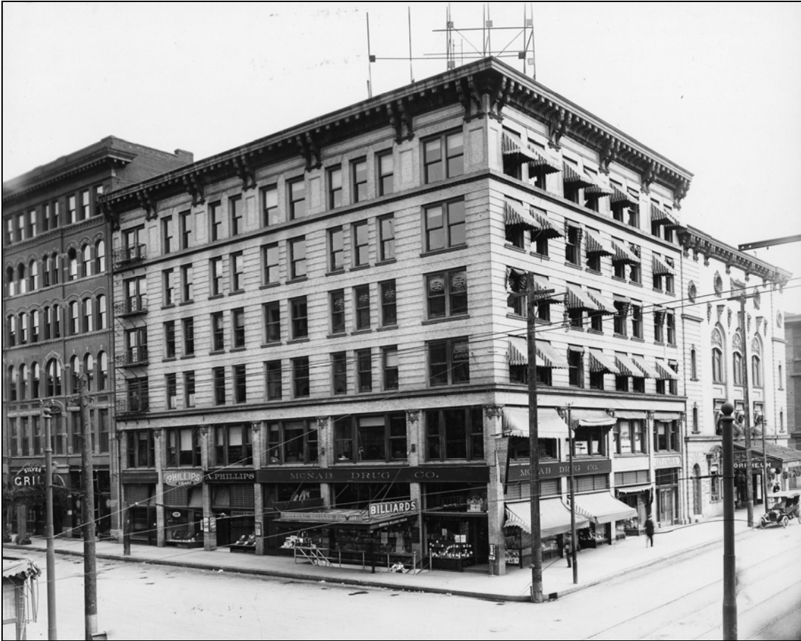
The Columbia Building in circa 1915, looking southeast at the building from First Avenue & Howard Street.
