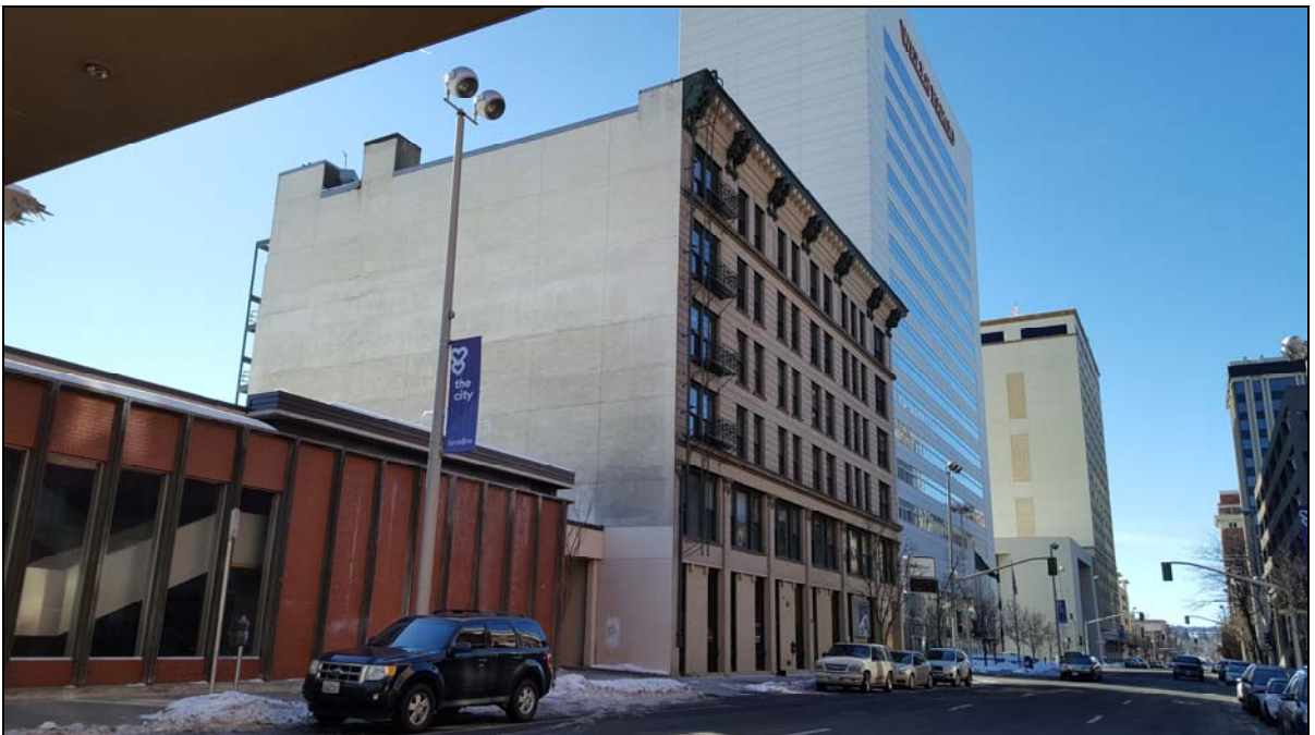
East face of Columbia Building in 2019, looking west
