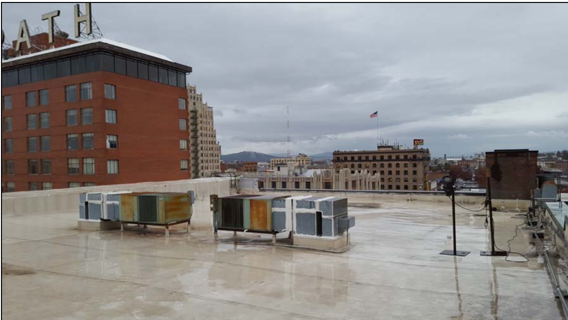
Roof of Columbia Building, looking east in 2019
