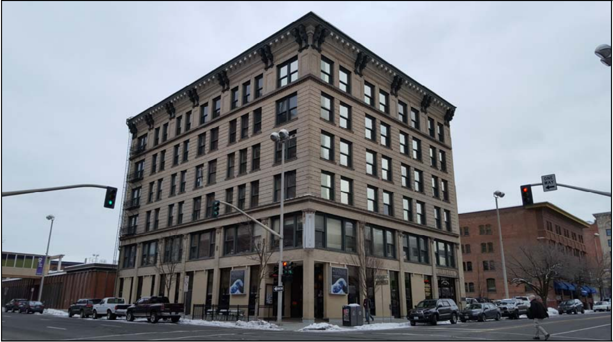
Columbia Building in 2019, northwest corner façade, looking southeast
