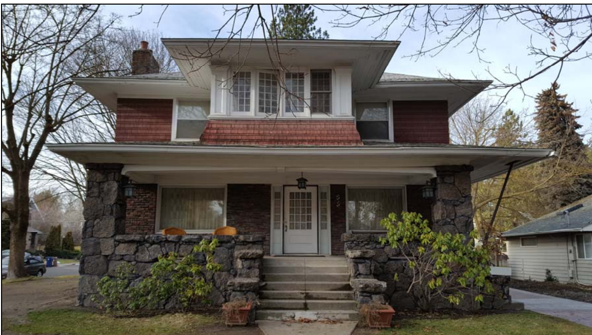
East façade of the Toevs House in 2019
