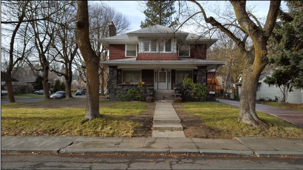
East façade of the Toevs House in 2019
