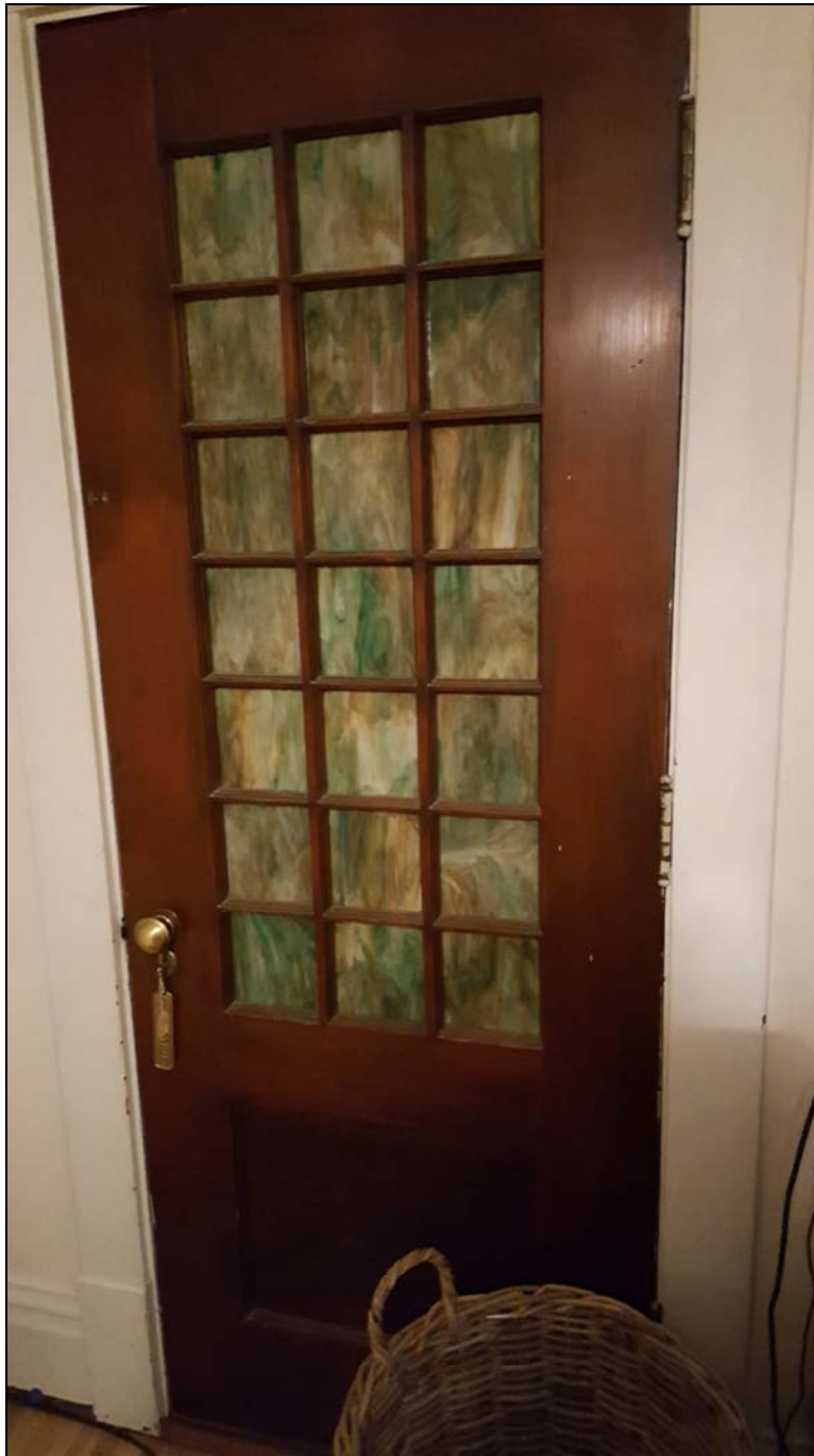
Stained-glass in door in southwest bedroom on the second floor; looking west in 2019 at the door, which opens to a sleeping porch in the southwest corner of the house.
