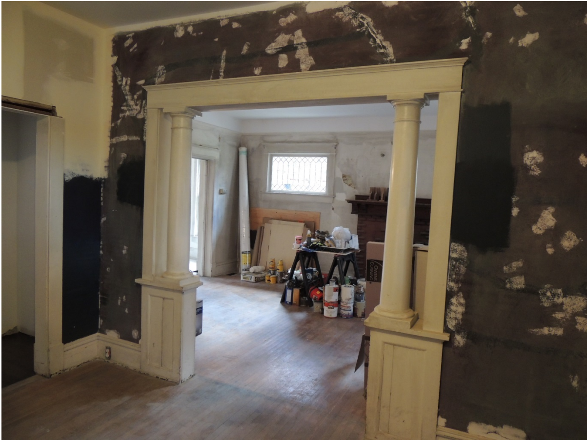
View from the library/parlor into the living room (north looking south)
