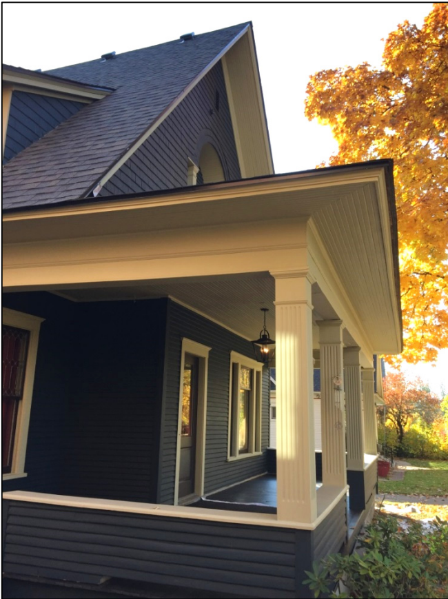
Front porch, west elevation
