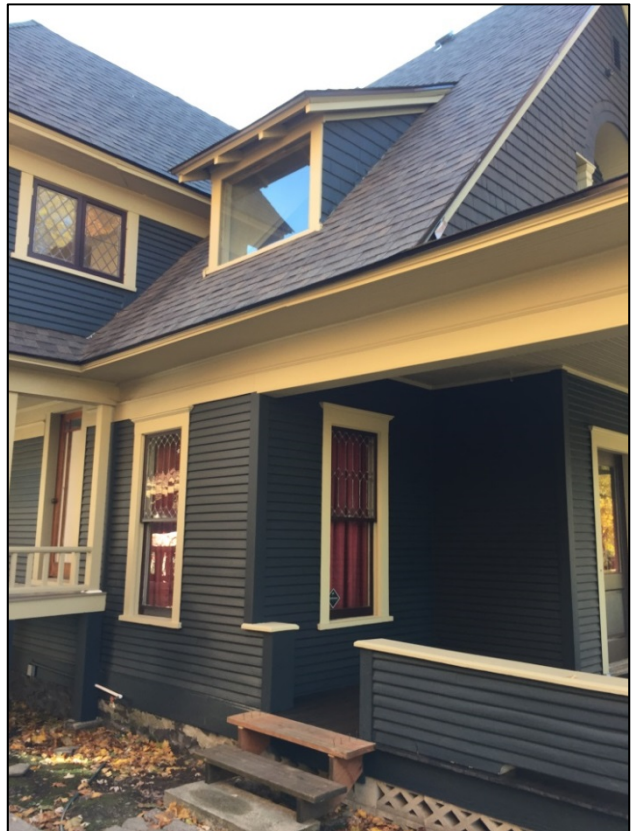
North elevation showing dormer and cross gable
