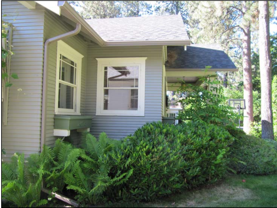
South side view of front porch in 2017
