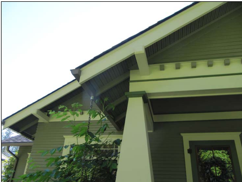
East façade front entry porch in 2017
