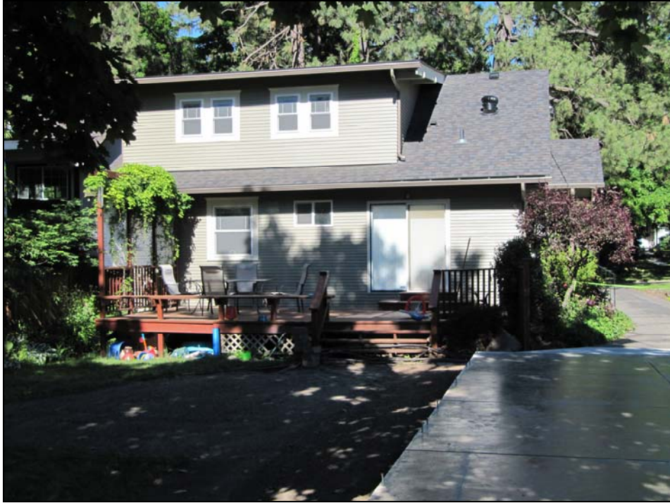
West rear of house in 2017, looking east
