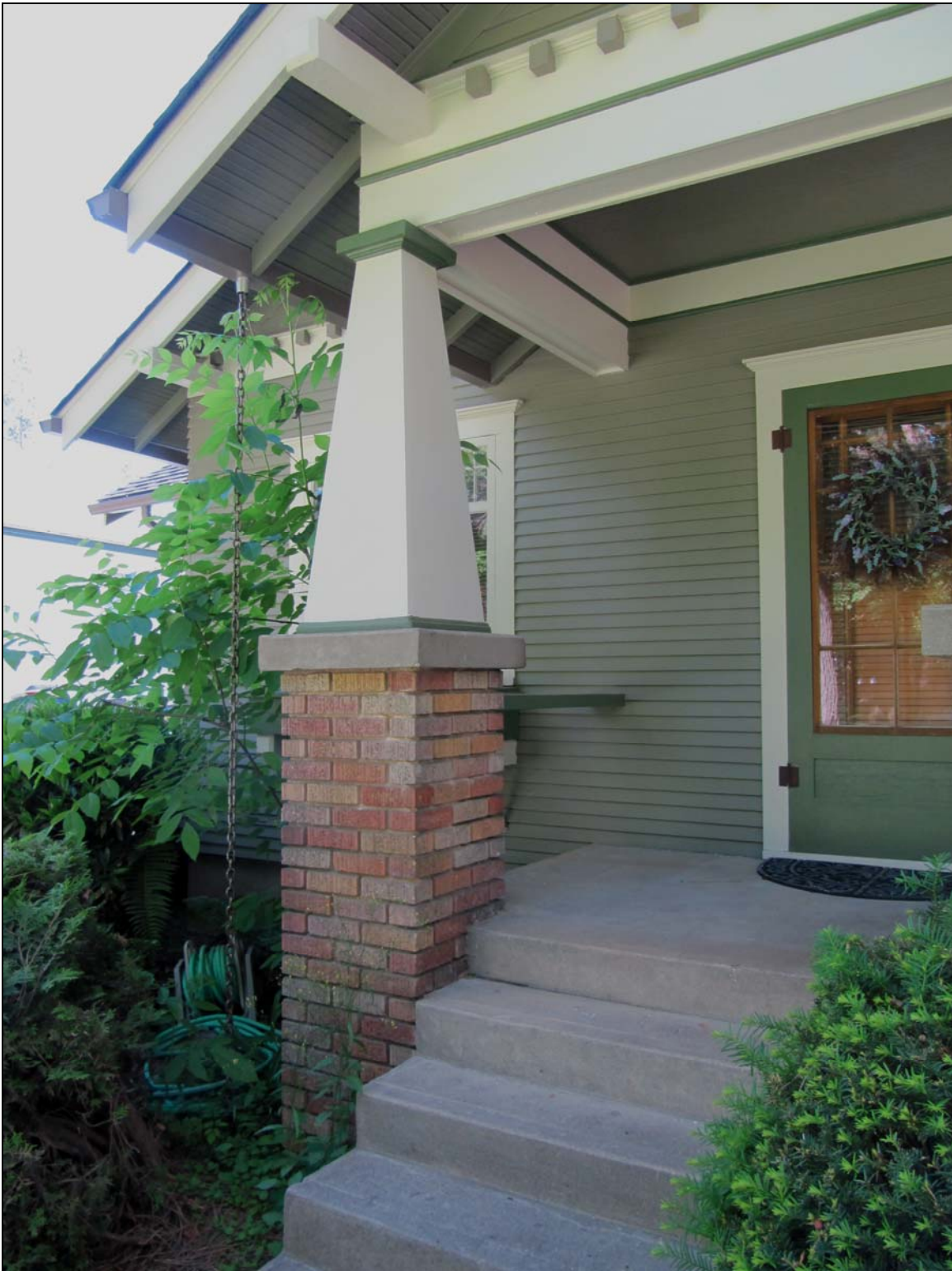
East façade front entry porch in 2017
