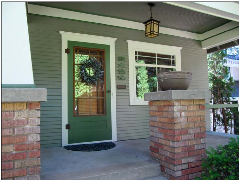
East façade front entry porch in 2017
