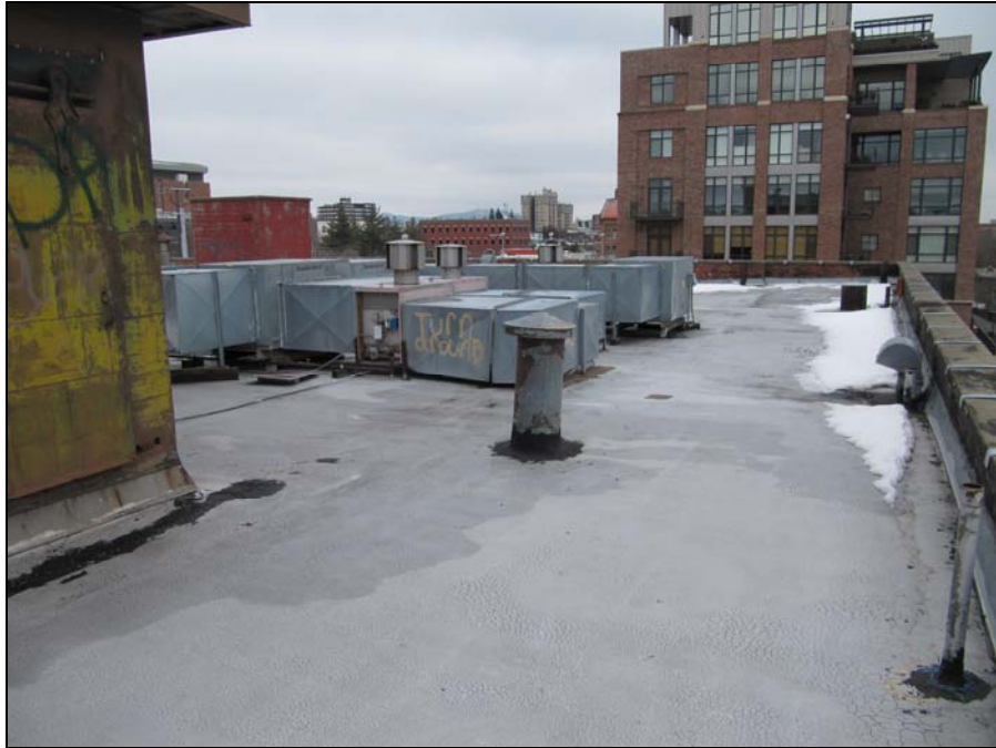
Roof in 2017, looking east at southeast corner of roof
