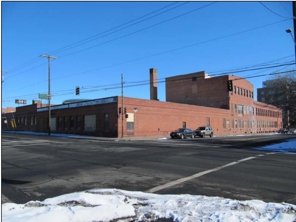
South façade and southwest corner of building in 2017
