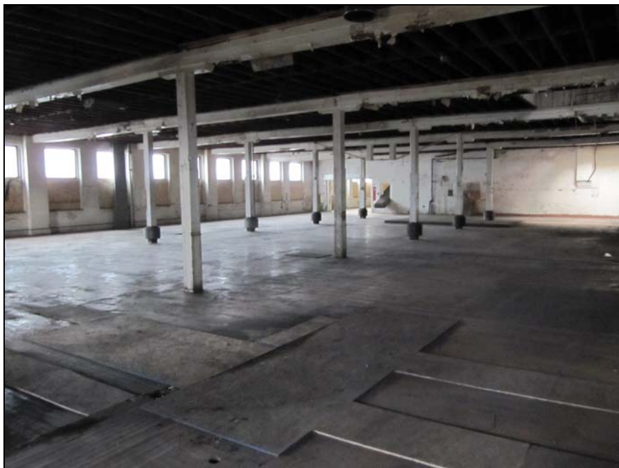
Second floor, looking southwest in 2017
