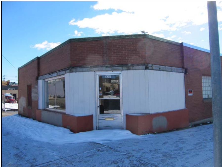
Rear northwest corner of attached garage/loading dock wing in 2017
