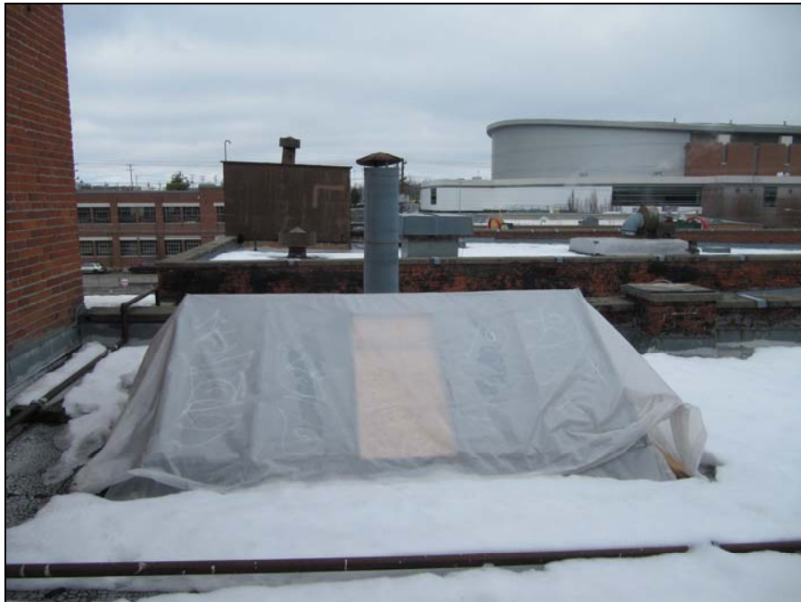
Roof, looking east in 2017
