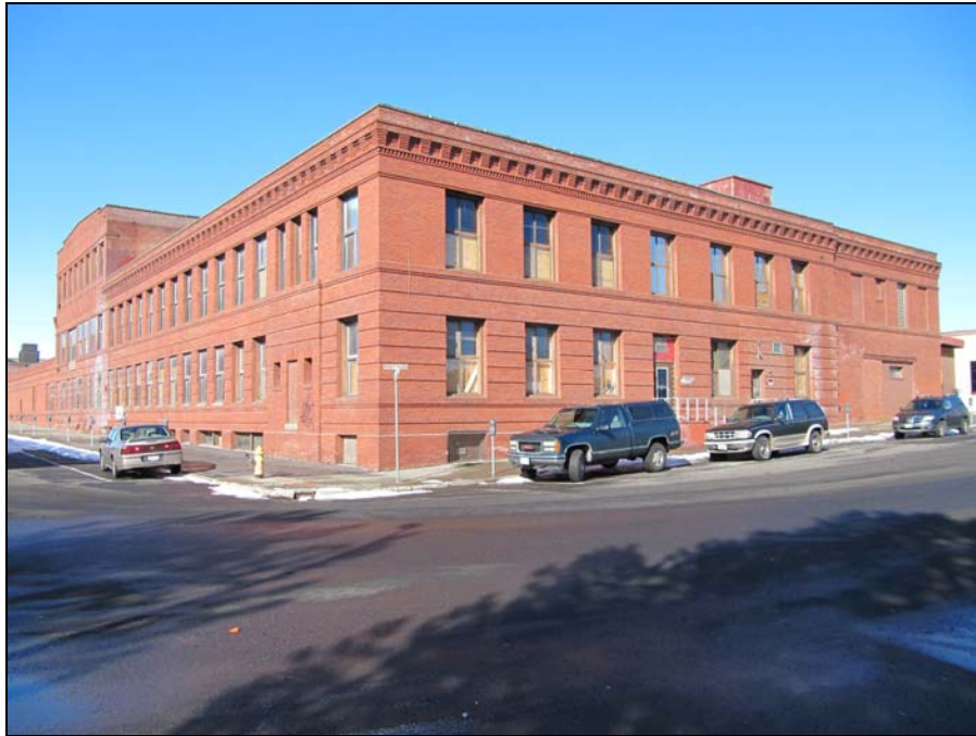
Southeast corner façade of building in 2017
