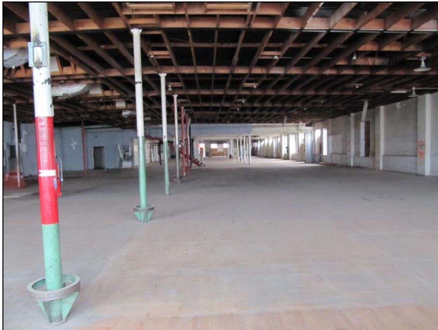
First floor in 2017, looking east
