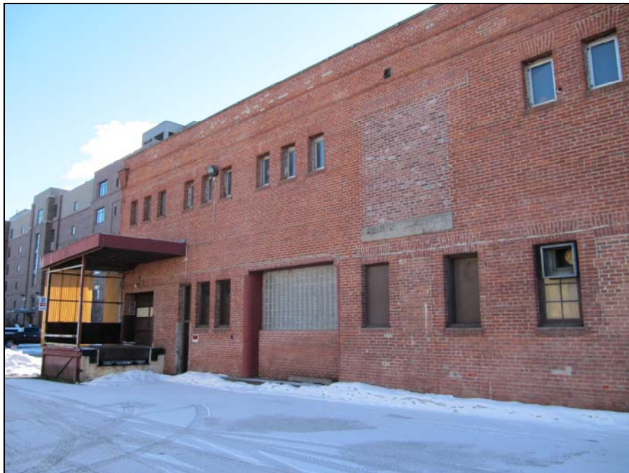
Rear north face of building in 2017
