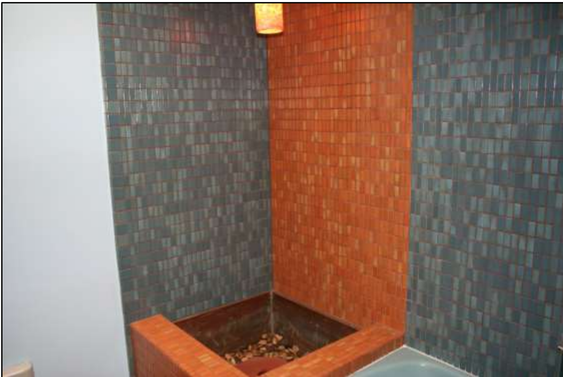
WH-39 Main family bathroom, planter detail, view to the north.
