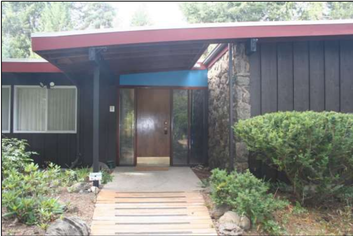
WH-1 Northeast (front) entry, view to the southwest.
