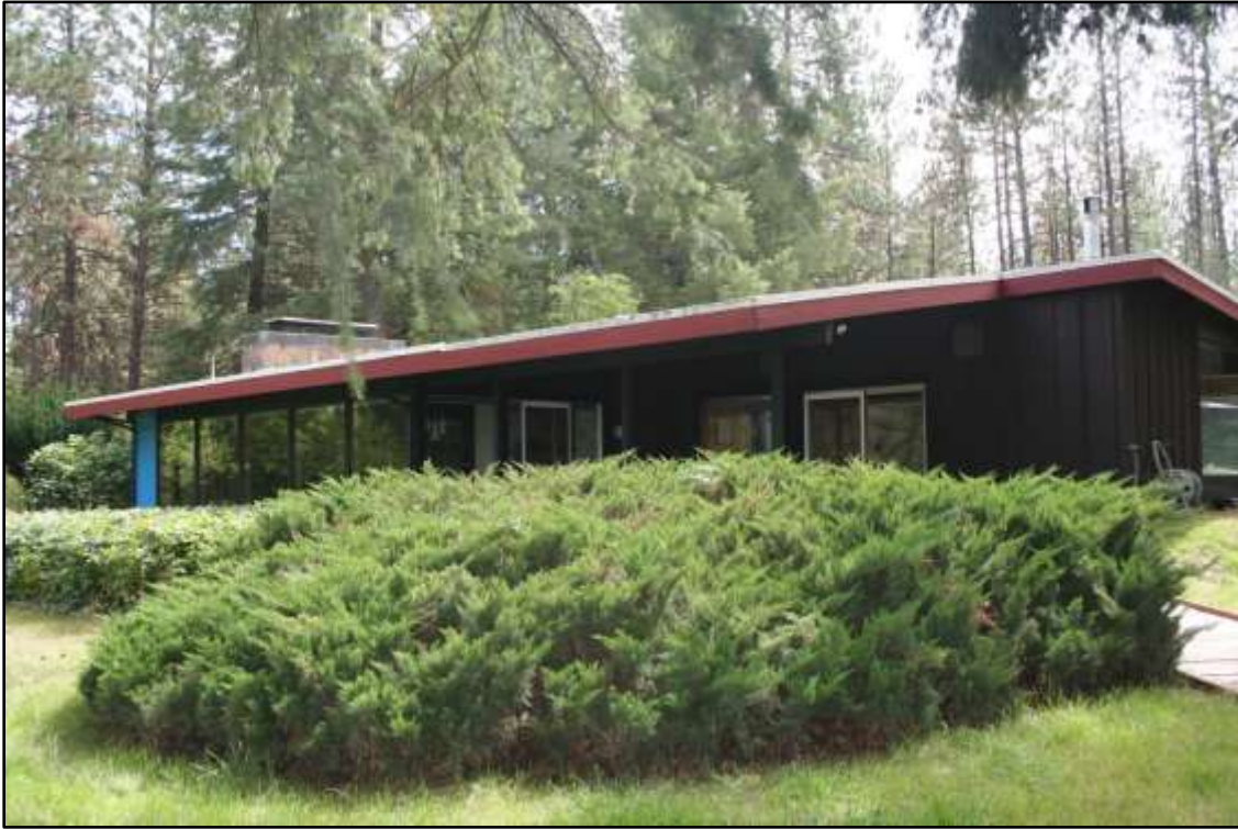
WH-15 Northwest and southwest elevations, view to the east.
