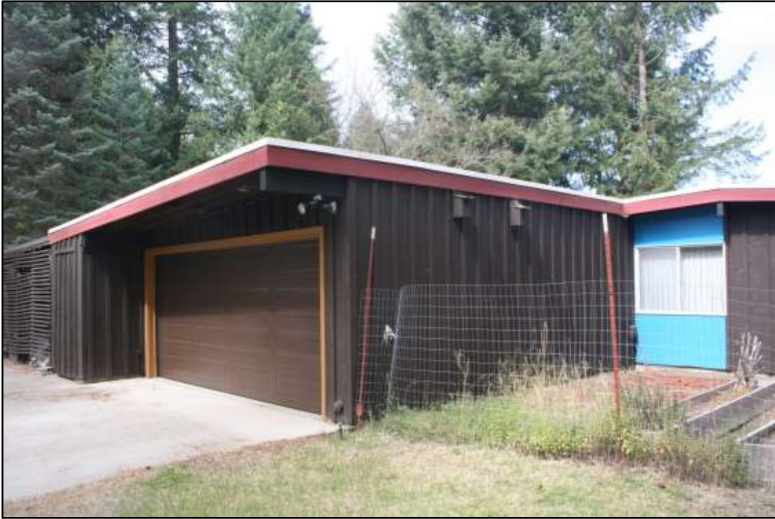
WH-7 Southeast and northeast elevations, garage door, view to the north.
