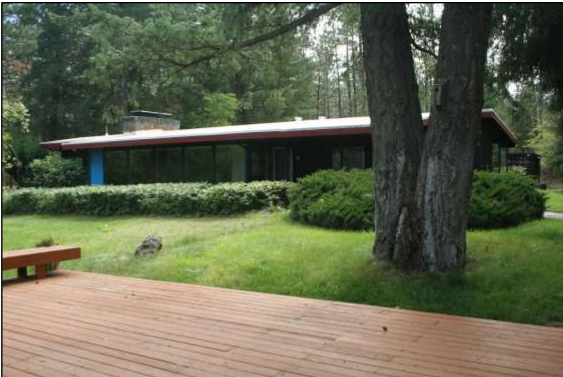
WH-12 Northwest elevation, view to the east.
