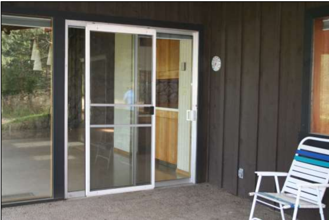
WH-16 Back patio entry detail, view to the east.
