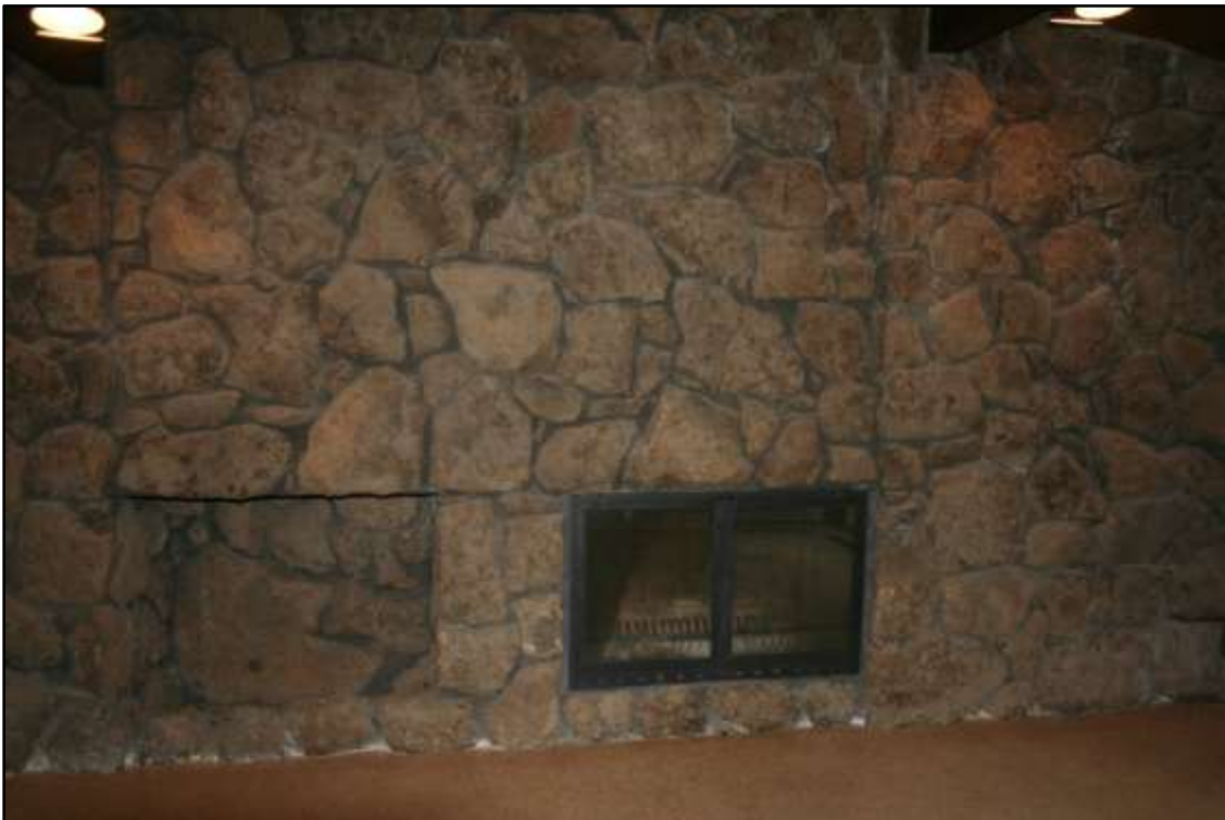
WH-20 Rock wall and hearth in the office/den, view to the southwest.
