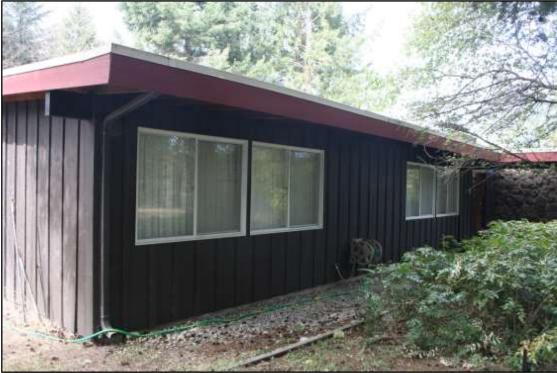
WH-5 Northeast elevation, view to the north.
