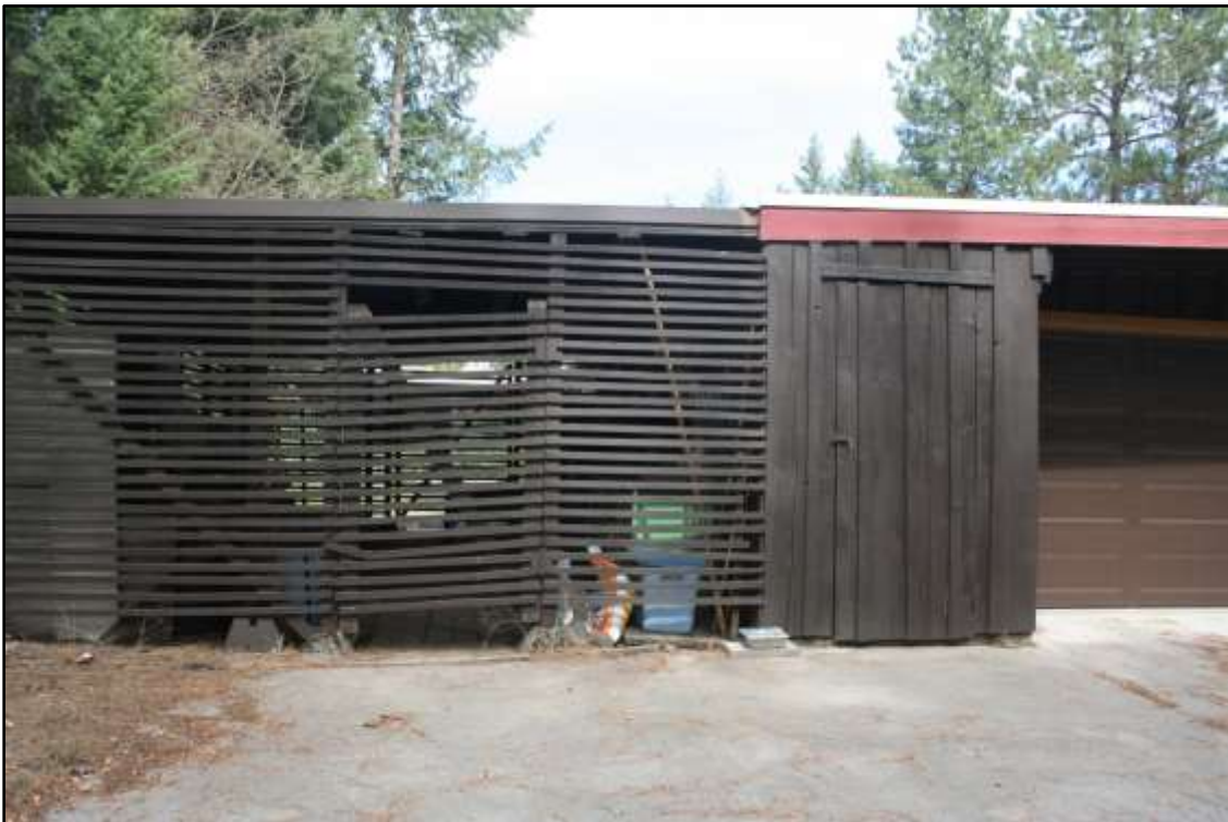
WH-8 Southeast elevation, attached garden shed, view to the northwest.
