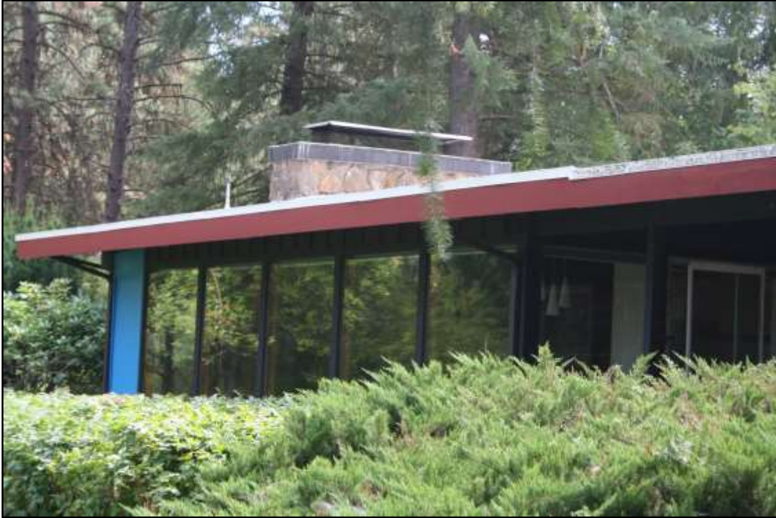
WH-13 Northwest elevation, chimney, view to the east.
