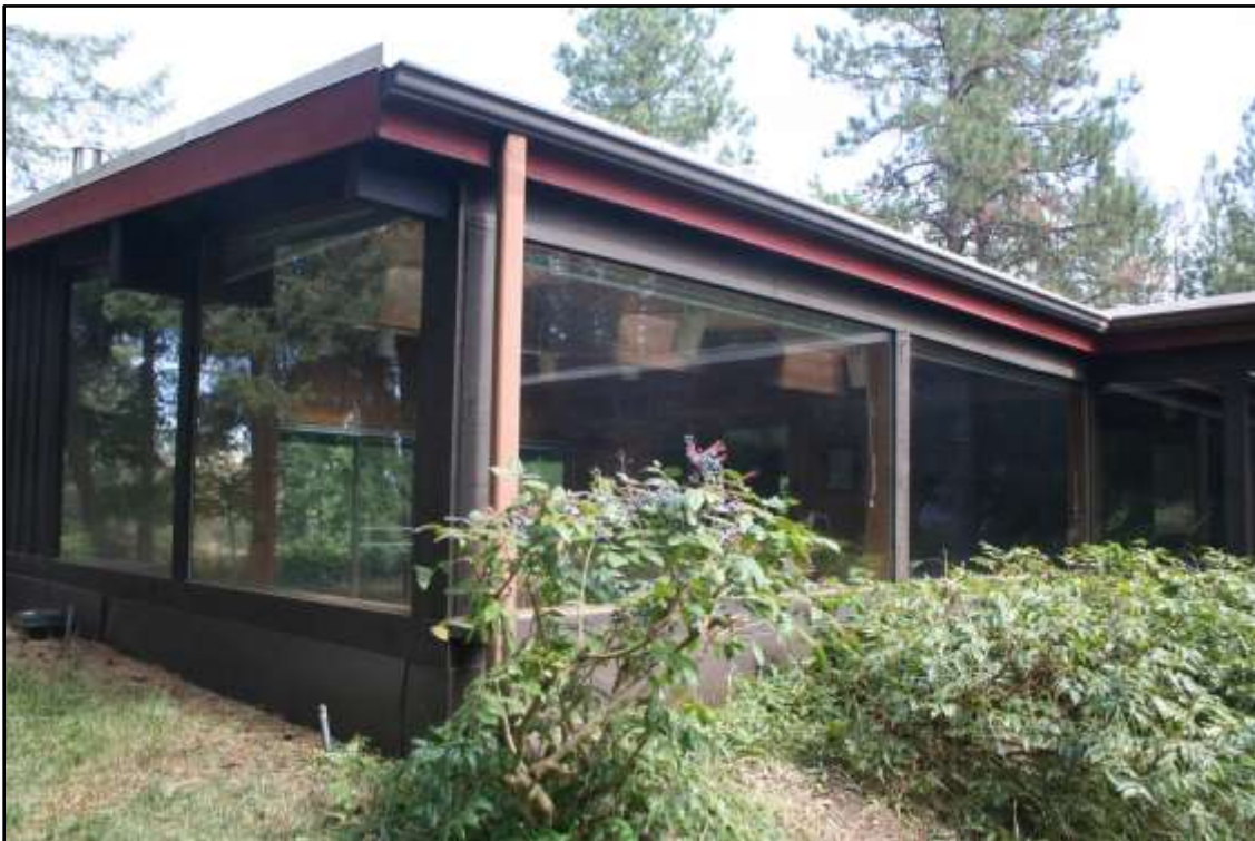
WH-10 Southeast and northeast elevation, view to the north.
