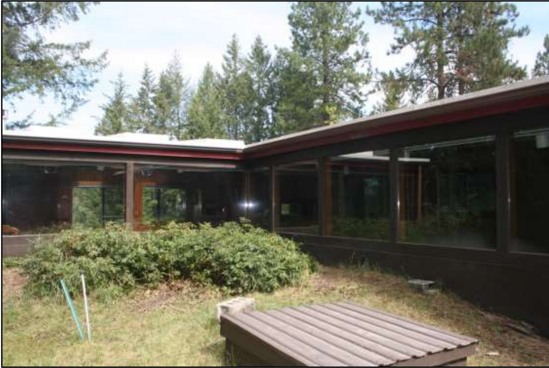
WH-9 Southeast and southwest elevations, view to the north.
