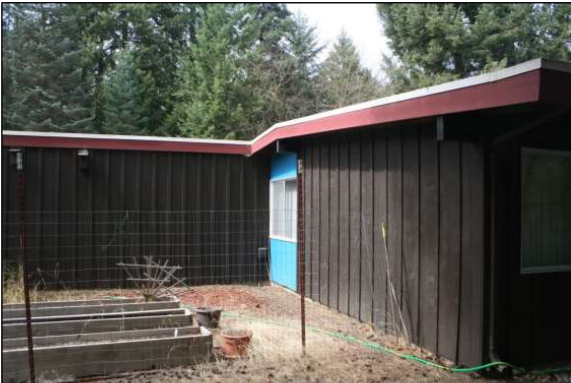
WH-6 Southeast elevation, garage wall, view to the north.
