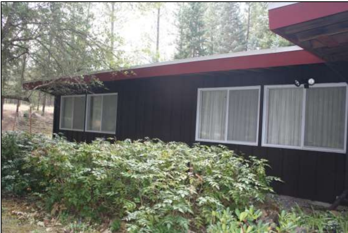
WH-4 Northeast elevation, left side, view to the south.
