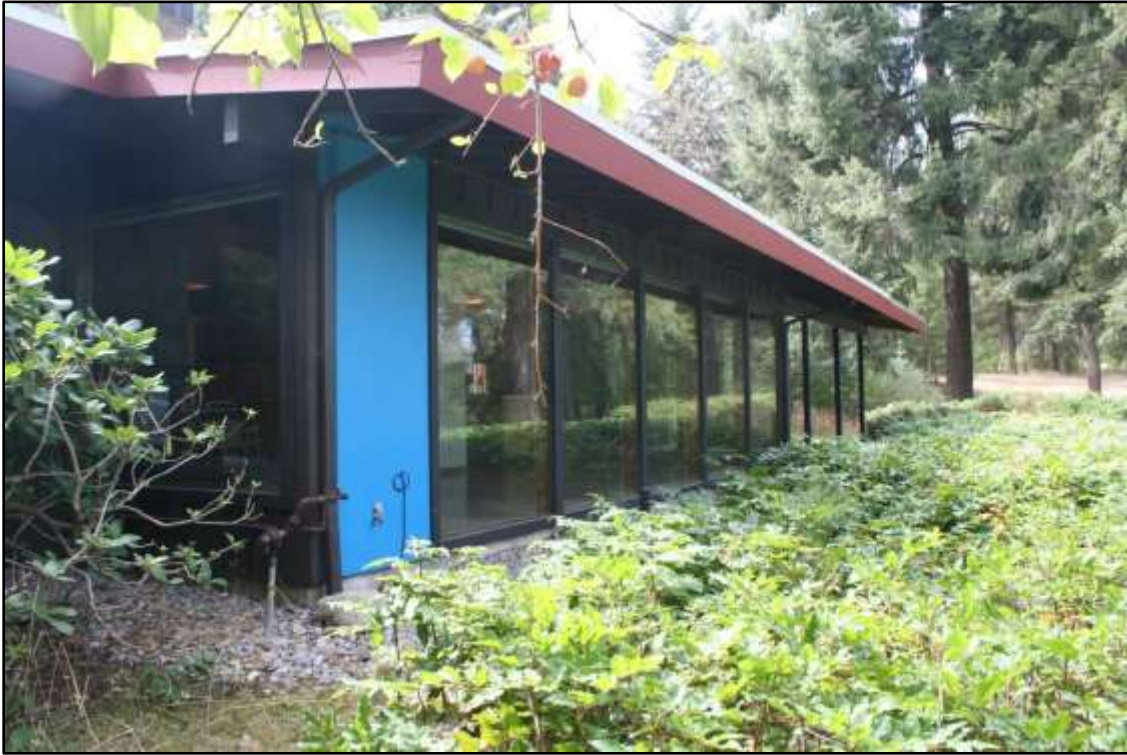
WH-17 Northwest elevation, view to the south.
