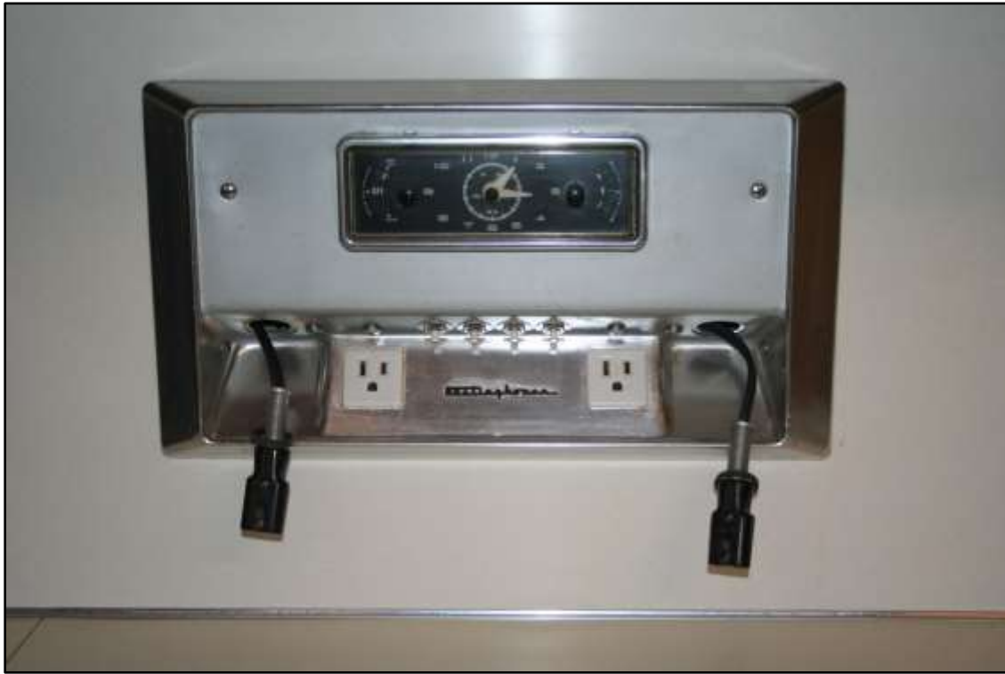
WH-32 Kitchen, Westinghouse timer and extension cord outlet, view to the northwest.
