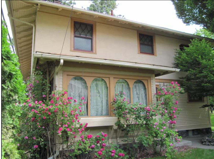
South rear face of house in 2015
