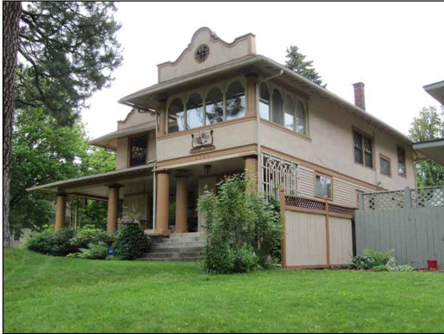
Northwest façade corner in 2015
