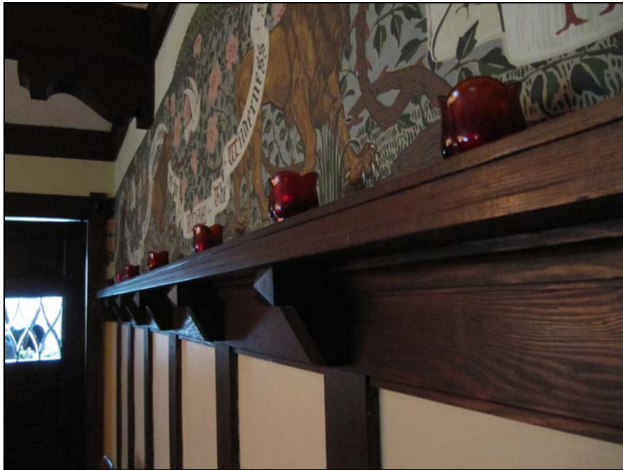
Ceiling brackets and plate rail in dining room in 2015
