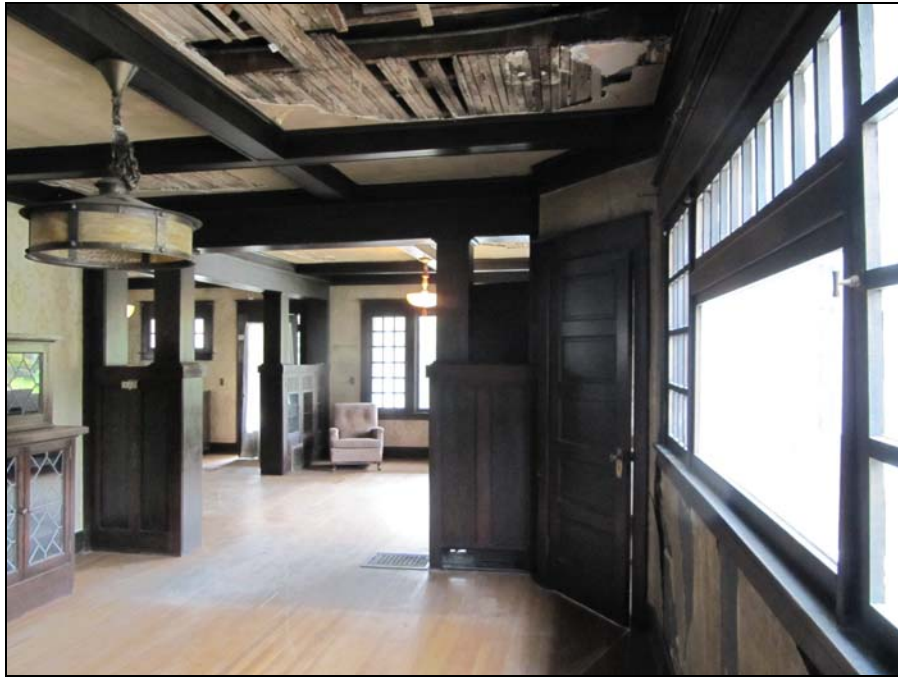
Dining room, living room, and front entrance, looking west in 2015
