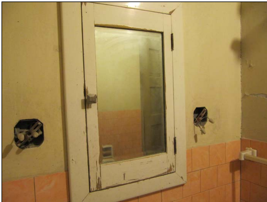
Built-in medicine cabinet above sink in 2 nd floor bathroom, looking west in 2015
