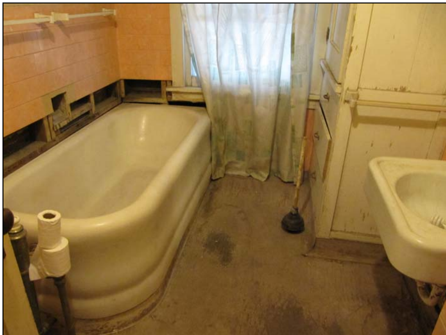
Circa 1910 bathtub on 2 nd floor, looking south in 2015
