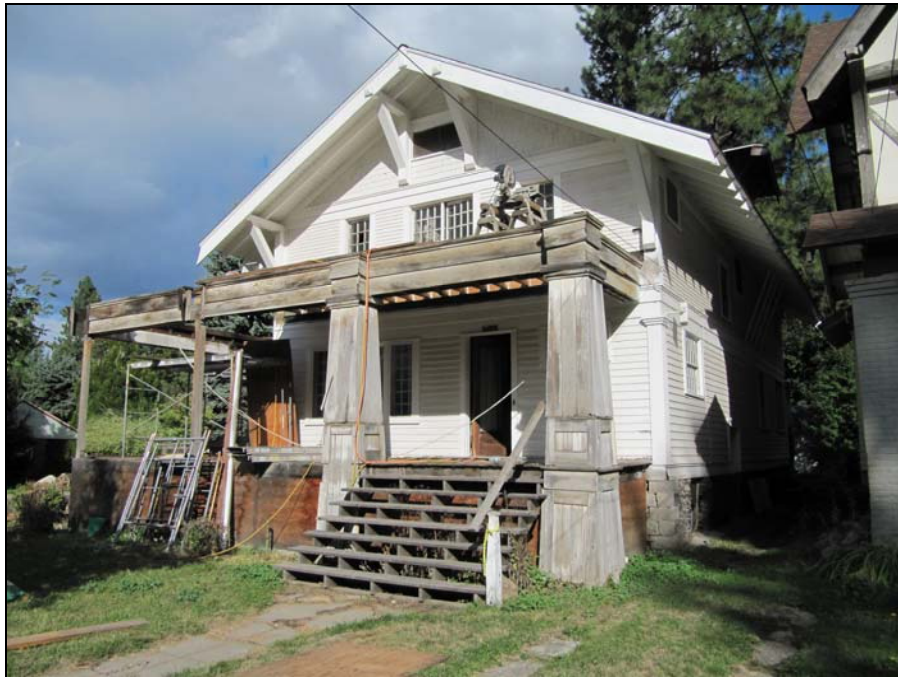
West façade in 2015
