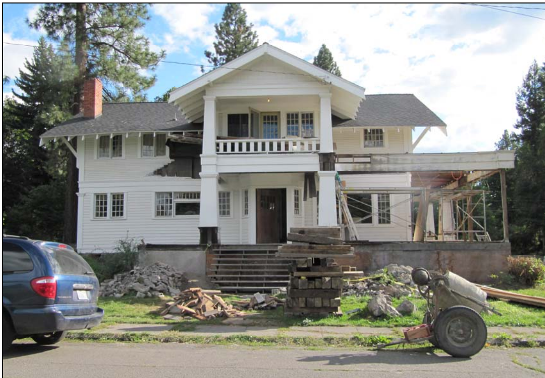
North façade in 2015
