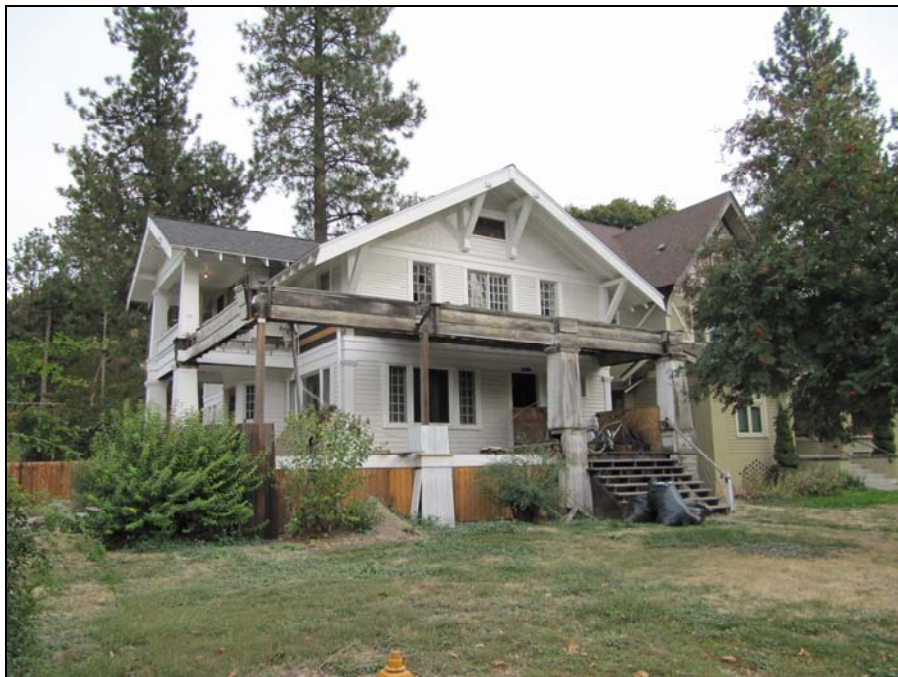
West façade in 2015
