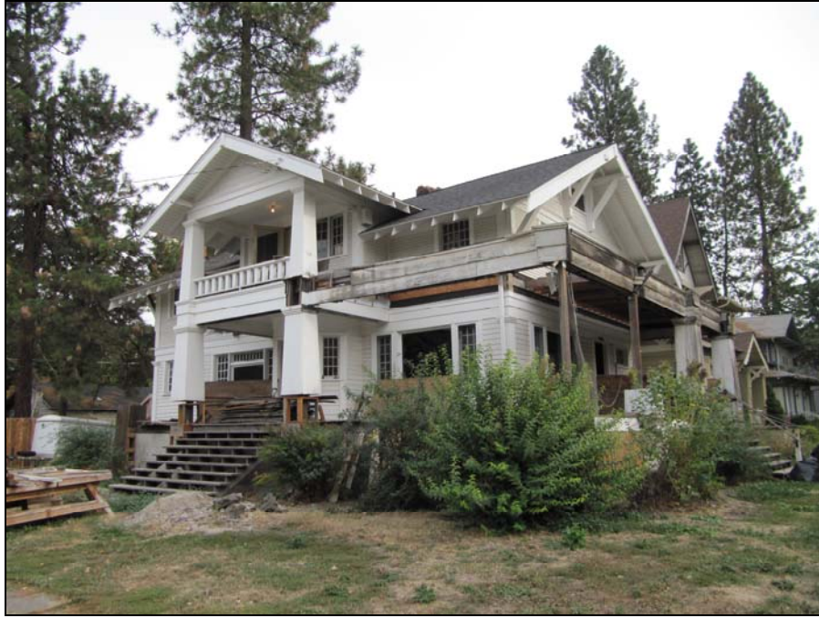
Northwest façade corner in 2015
