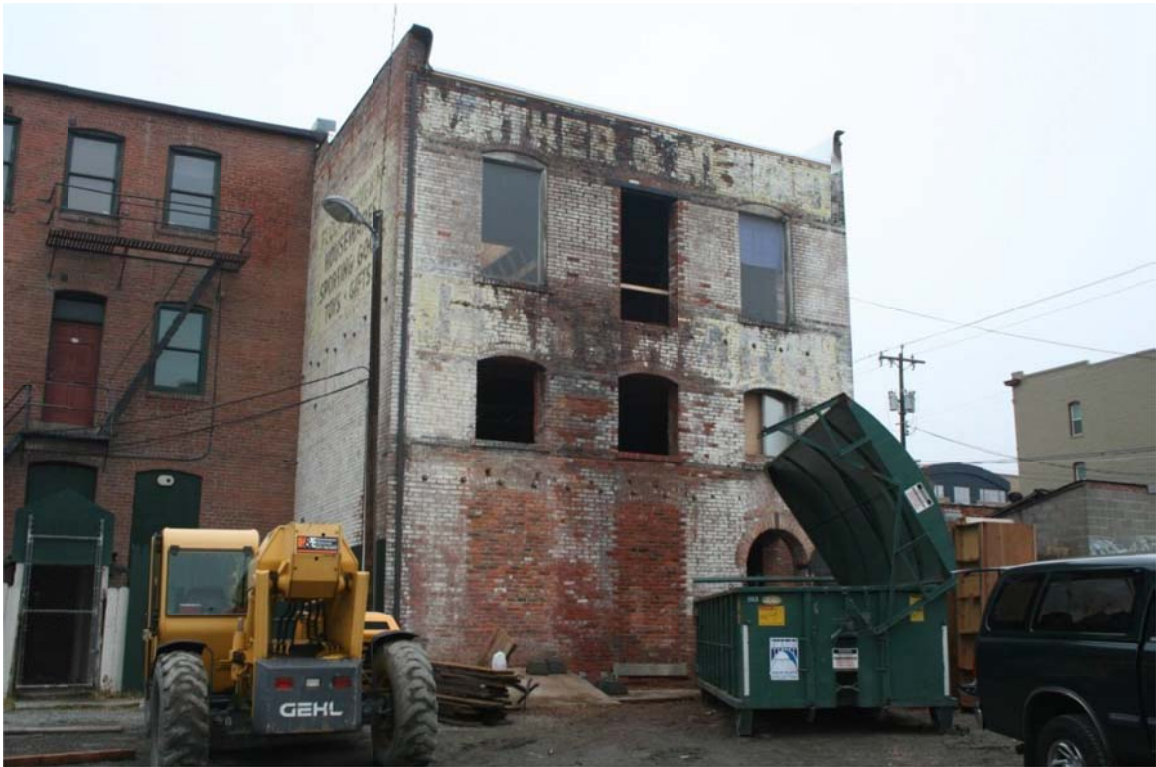
VNH-7 East (rear) and south facades, view to the northwest.
