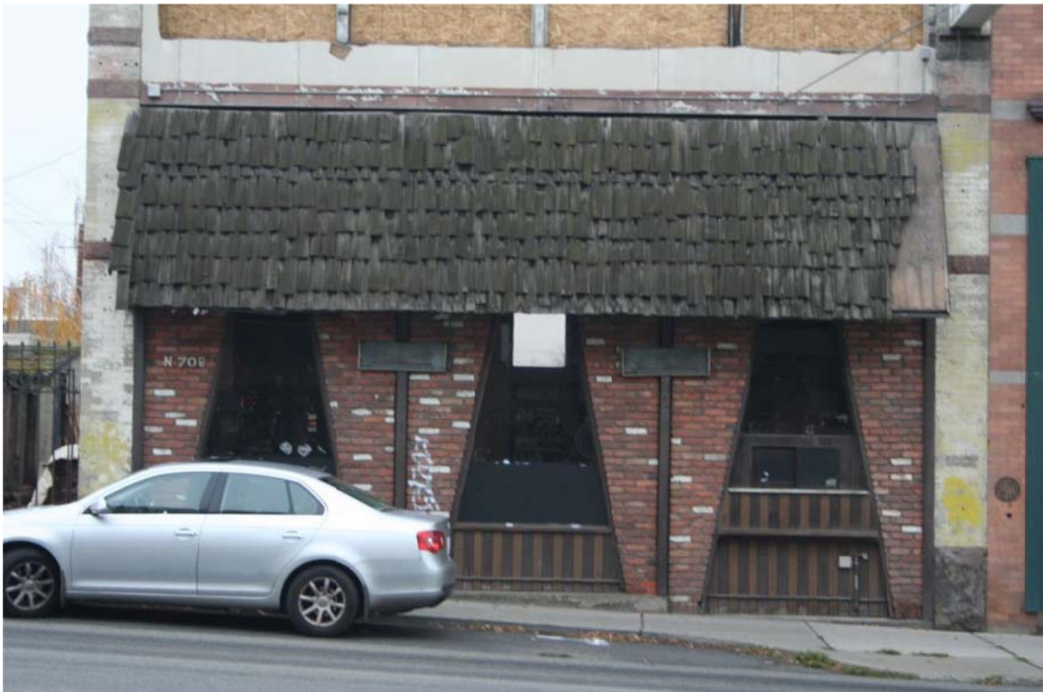
VNH-6 West (front) façade, lower level, view to the east.
