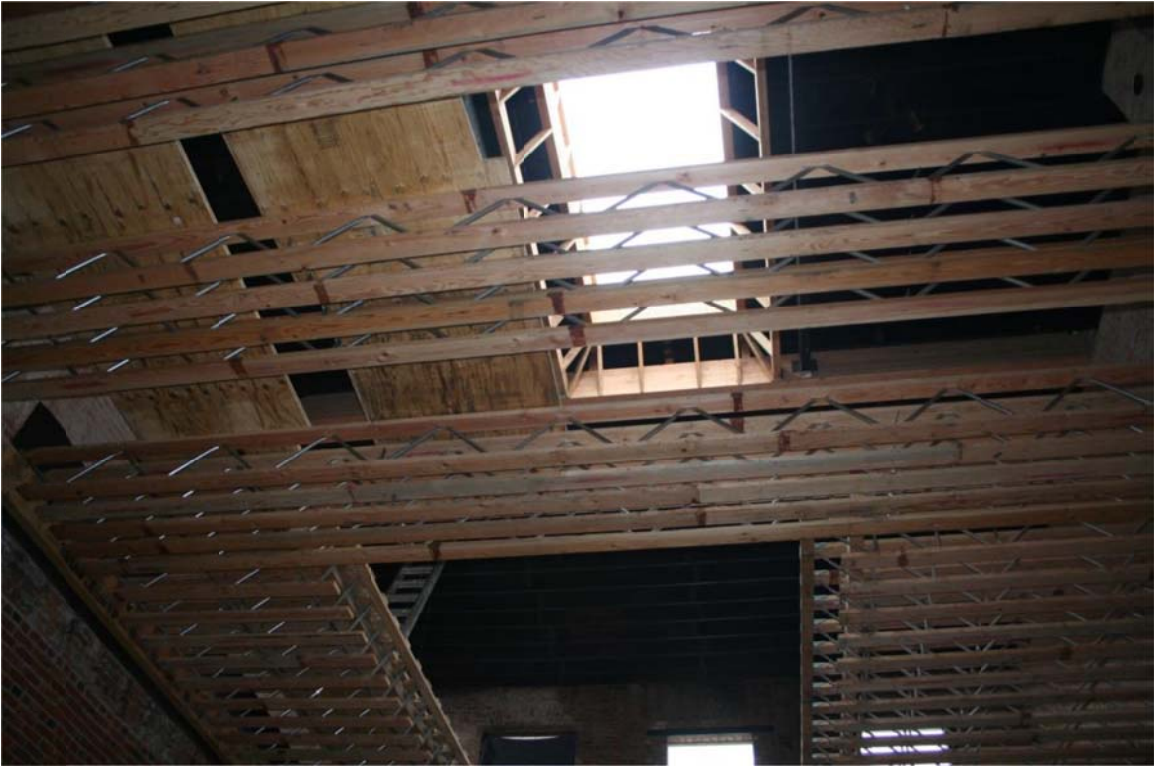
VNH-11 Floor joists, new, view to the east.
