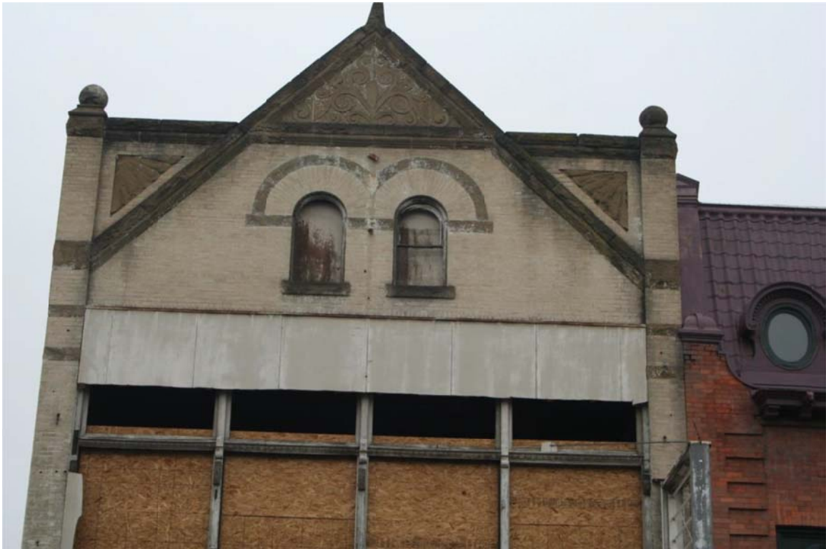
VNH-5 West (front) façade, upper level, view to the east.
