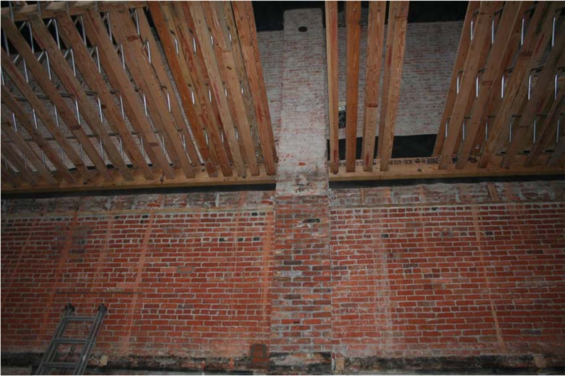
VNH-13 Interior, chimney pilaster, view to the south.
