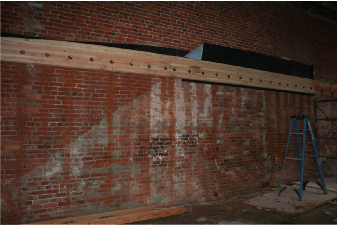
VNH-14 Imprint left by stair removal, view to the northeast.
