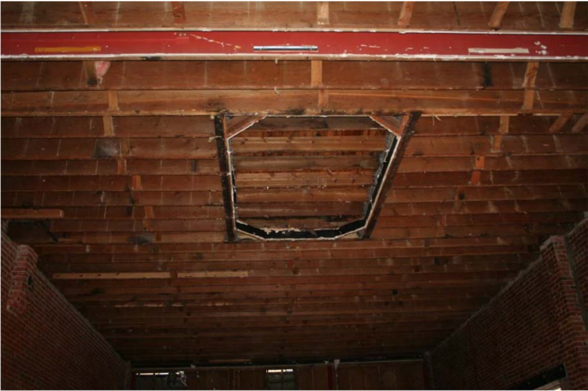
VNH-10 Floor joists, old, view to the west.
