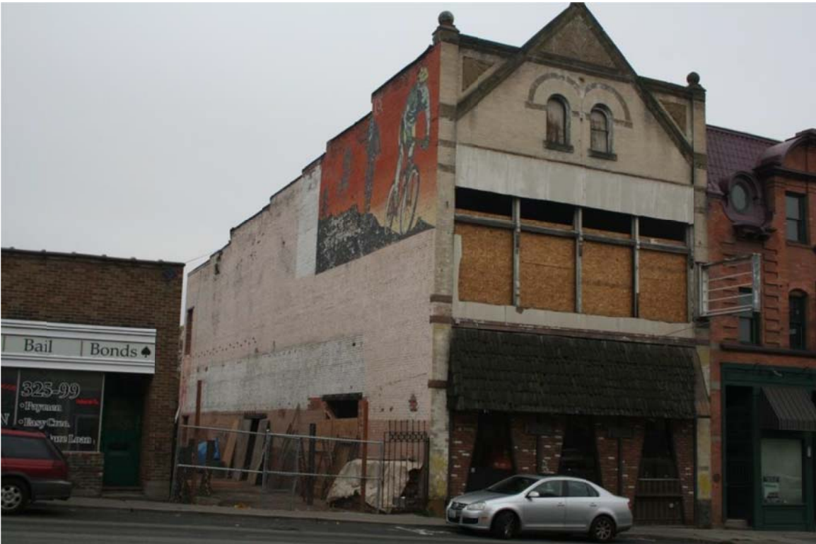
VNH-4 West (front) façade, view to the southeast.
