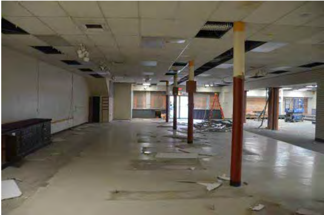
Photo 3 - Looking North Toward Main Entry Showing Bay #s 409, 411, 415
