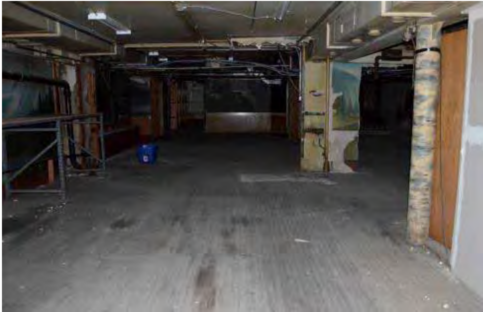
Photo 1 - Looking North at Basement of Dutch's (Durkin's/Ulrich's)
