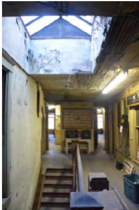
Photo 4 - Looking North on 3rd Floor Stairwell and Skylight
