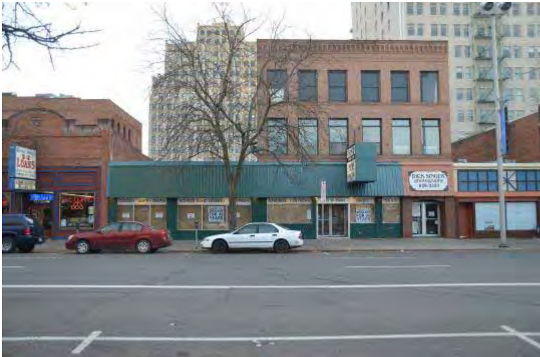
Photo 4 – Looking South at Front Façade of Dutch's (Jimmie Durkin's Building on West Side)
