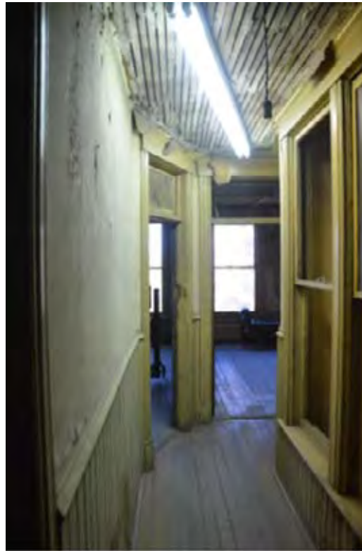
Photo 5 - Looking North at Hallway to Hotel Rooms at North End
