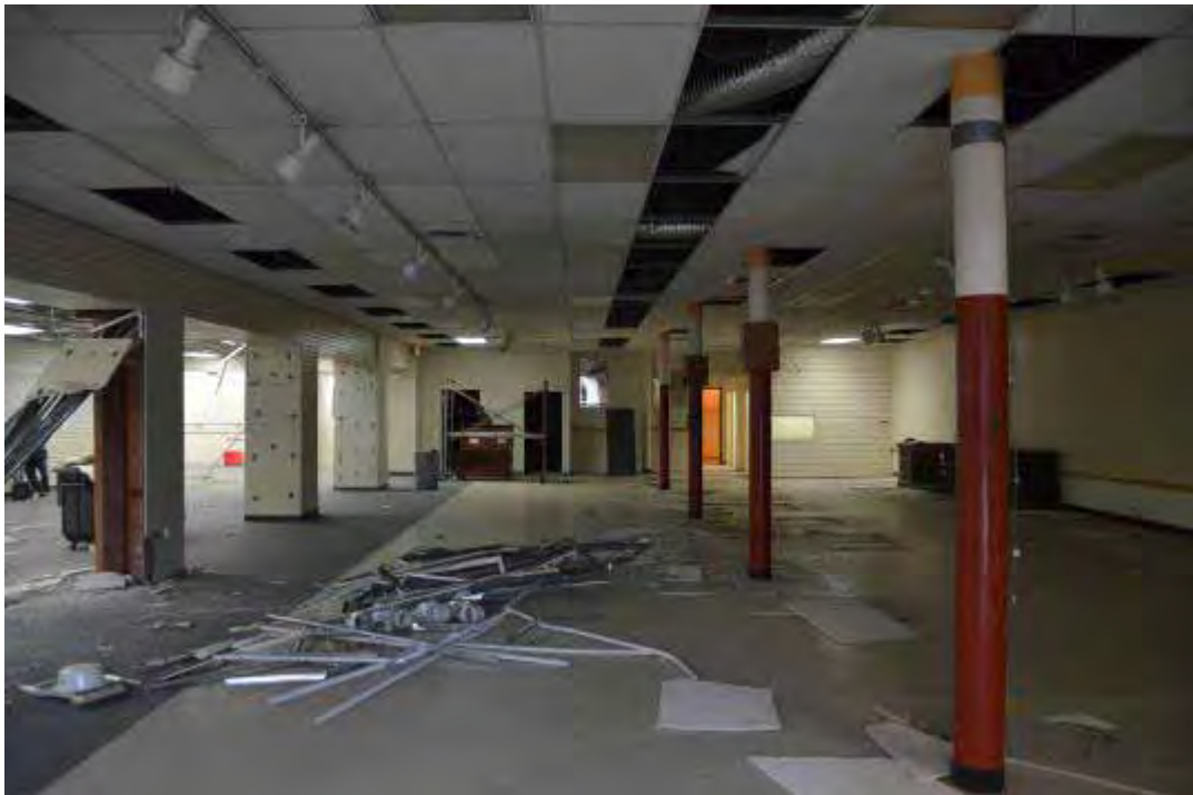
Photo 4 - Looking South from Main Entry (#415 - #s 411 & 409 to East)
