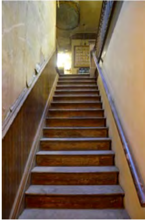
Photo 3 - Looking South up Stairs from 2nd to 3rd Floor
