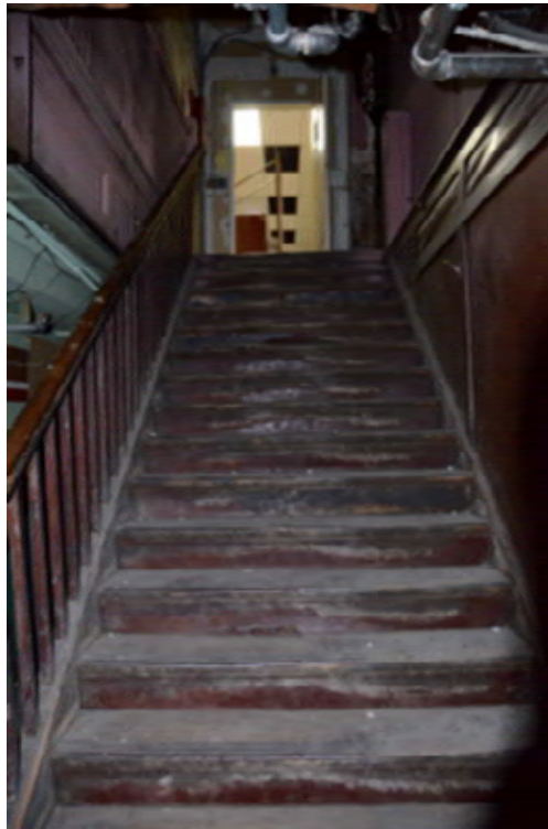
Photo 2 – Looking North Up Stairs from Basement to 1 st Floor
