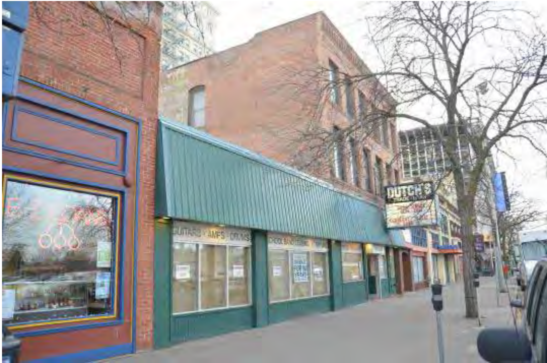
Photo 3 – Looking West at NE Corner of Dutch's
