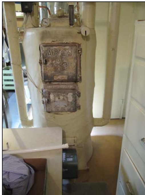
Original boiler in basement in 2015
