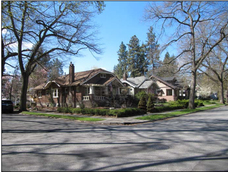
Looking at northeast corner of house from intersection of 27 th Avenue and Division Street in 2015
