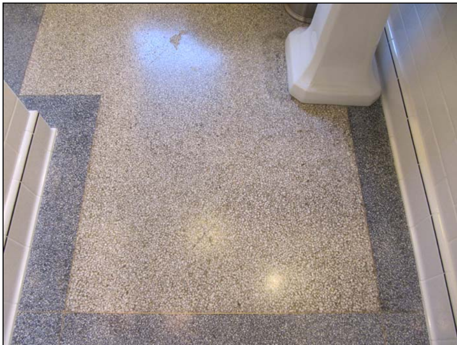
Bathroom with original terrazzo floor in 2015
