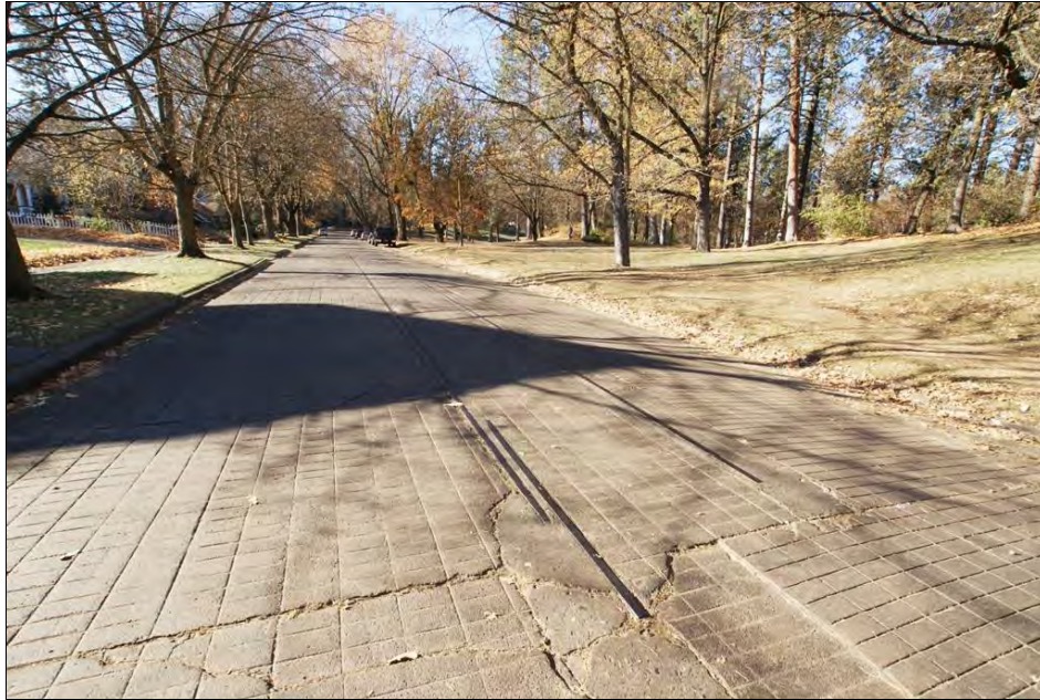
Photo 17. WA_SpokaneCounty_ManitoParkAndBoulevard_0017. Trolley Tracks, view west.
