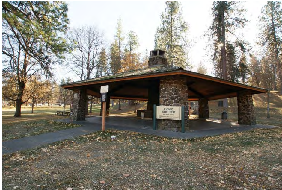
Photo 12. WA_SpokaneCounty_ManitoParkAndBoulevard_0012. Rotary Club Picnic Shelter, view southeast.
