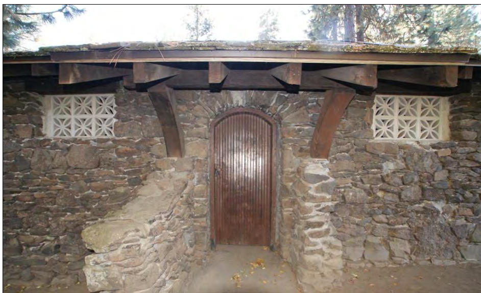
Photo 26. WA_SpokaneCounty_ManitoParkAndBoulevard_0026. Detail of entrance to storage shed, with original door, view south.
