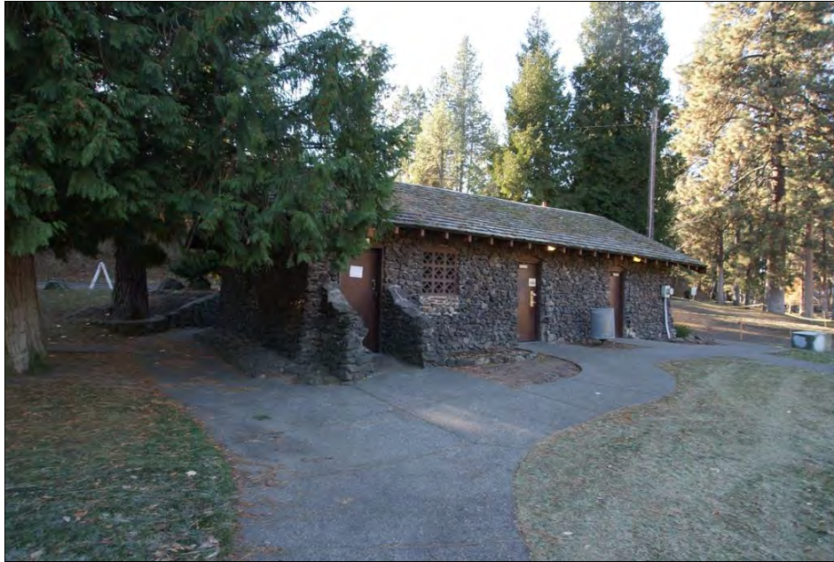
Photo 15. WA_SpokaneCounty_ManitoParkAndBoulevard_0015. Restroom No. 1, view southwest.
