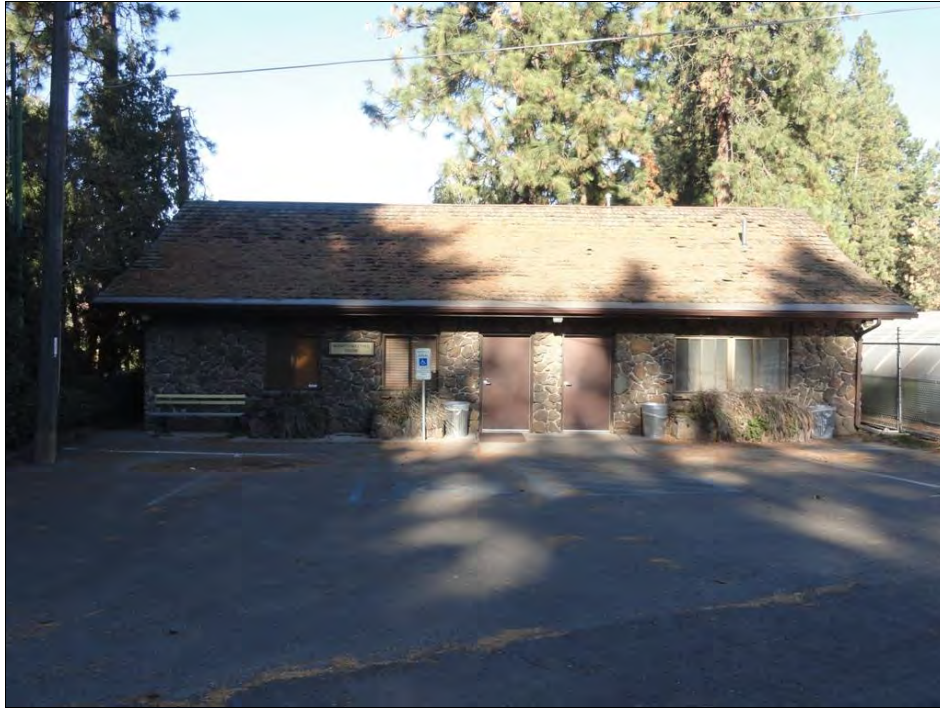
Photo 21. WA_SpokaneCounty_ManitoParkAndBoulevard_0021. Manito Meeting Room, view north.
