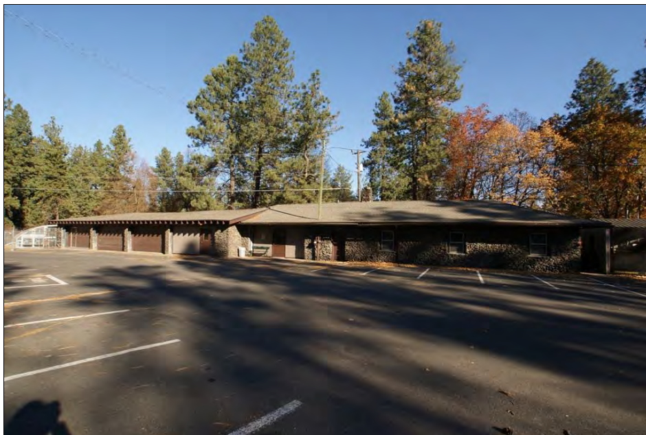
Photo 22. WA_SpokaneCounty_ManitoParkAndBoulevard_0022. Garage No. 1, view northeast.
