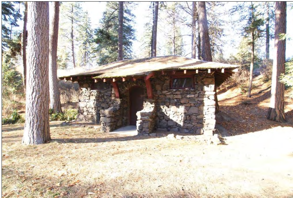
Photo 20. WA_SpokaneCounty_ManitoParkAndBoulevard_0020. Ancillary Building, view west.
