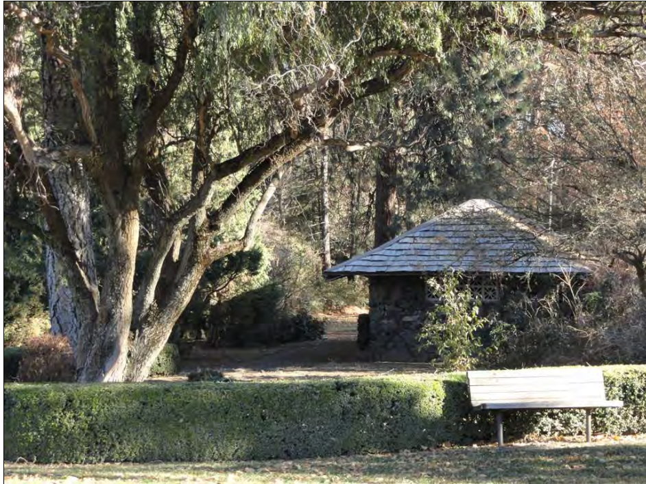
Photo 25. WA_SpokaneCounty_ManitoParkAndBoulevard_0025. Storage Shed, view east.
