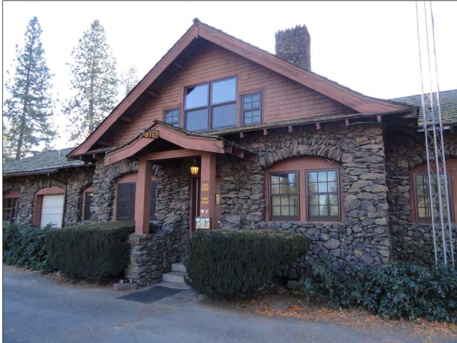
Photo 5. WA_SpokaneCounty_ManitoParkAndBoulevard_0005. Detail of Administrative Offices, view south.
