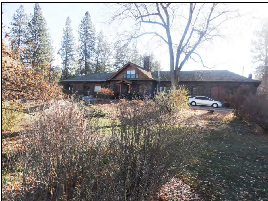
Photo 4. WA_SpokaneCounty_ManitoParkAndBoulevard_0004. Administrative Offices and Joel E. Ferris Perennial Gardens, view southeast.
