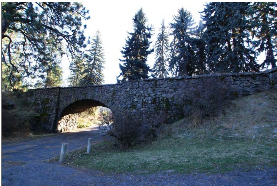
Photo 28. WA_SpokaneCounty_ManitoParkAndBoulevard_0028. Loop Road Bridge, view southwest.
