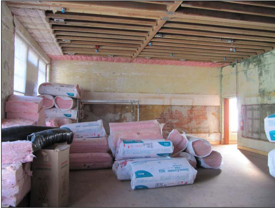
Looking east in north classroom on first floor in 2015
