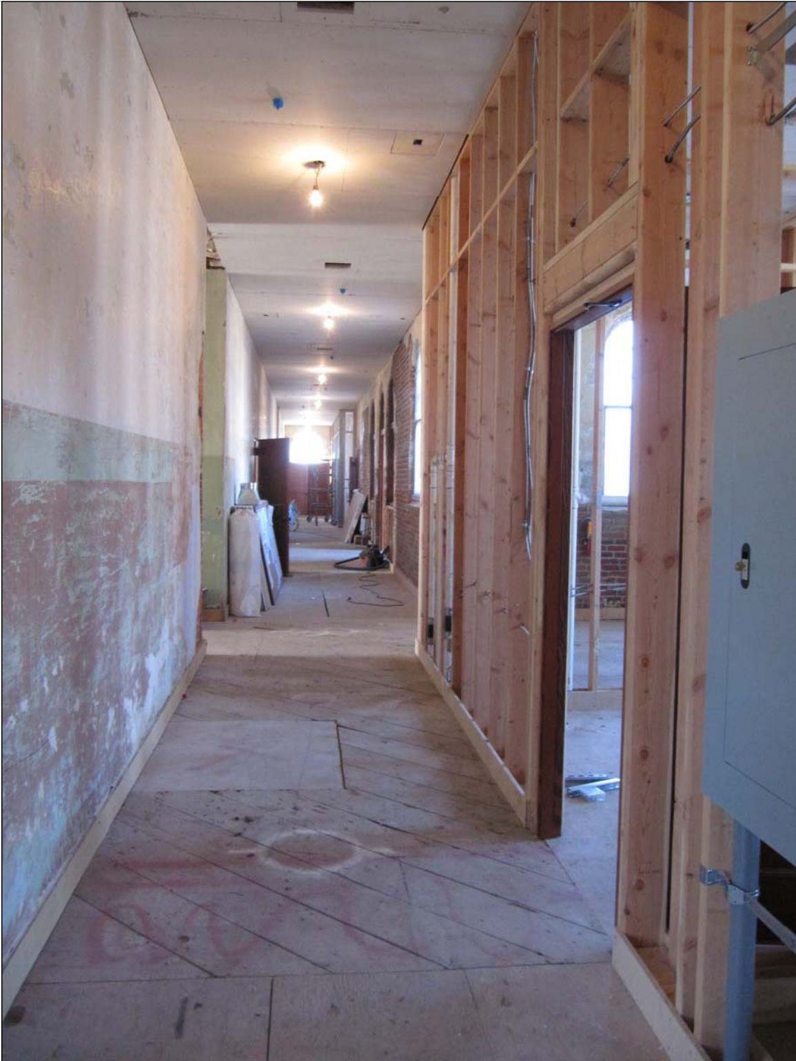
Looking south down center hallway on first floor in 2015
