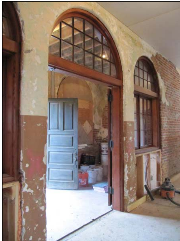
First floor, looking northwest into front vestibule and front door in 2015
