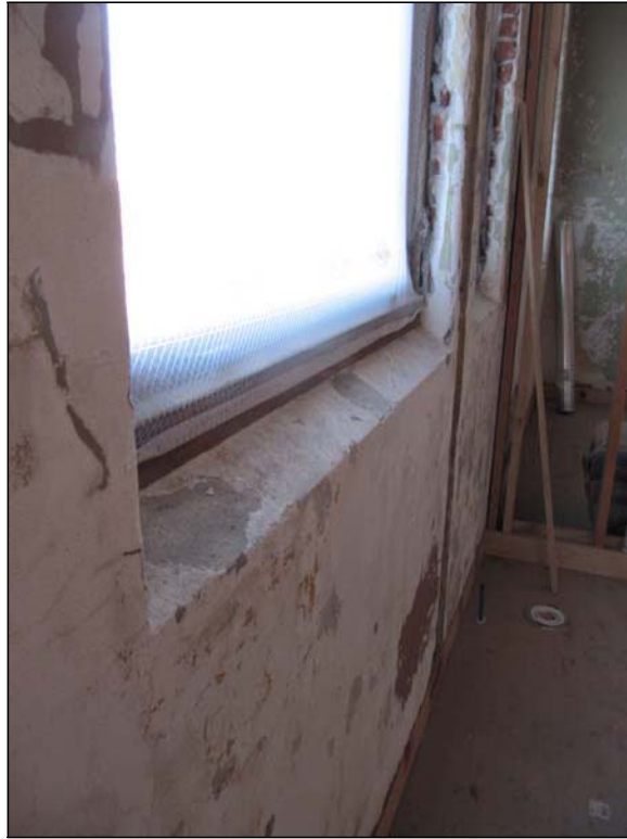
Window sill detail in 2015
