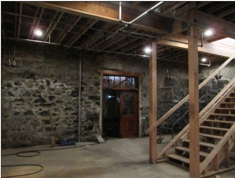
Basement, looking east in 2015
