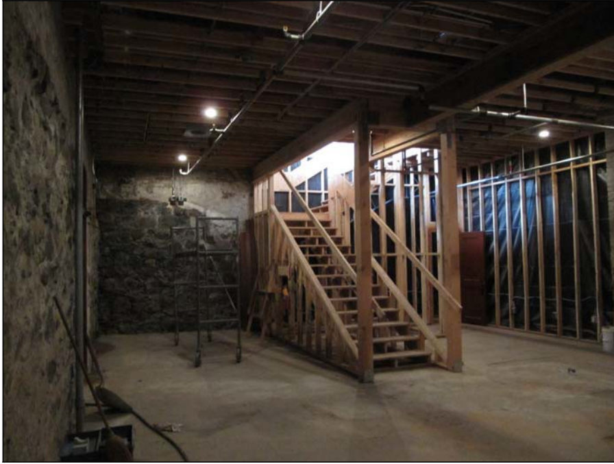
Basement, looking southwest in 2015
