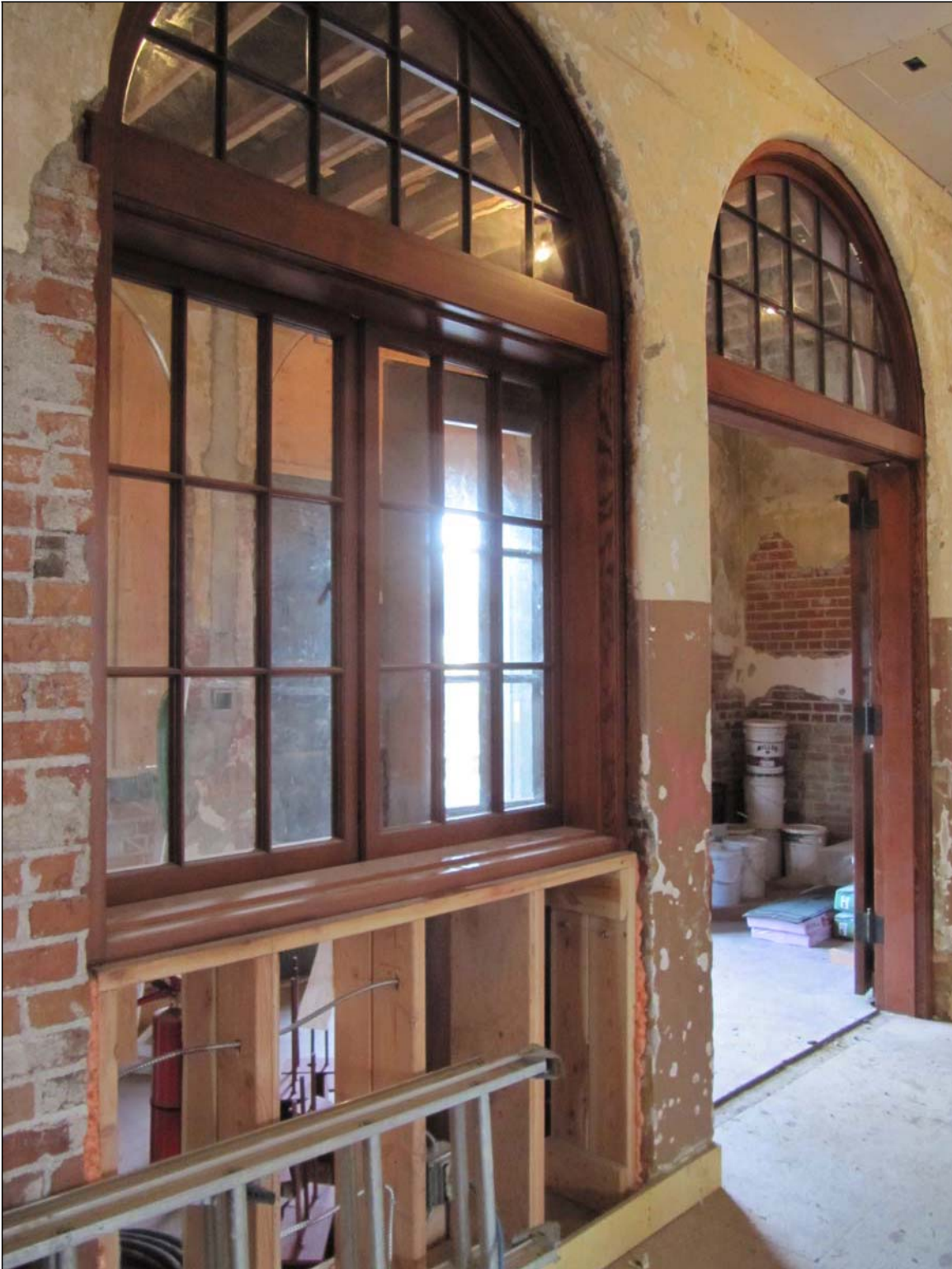
First floor, looking northwest in 2015 into front vestibule
