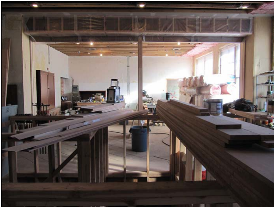
Looking north in center classroom on first floor in 2015
