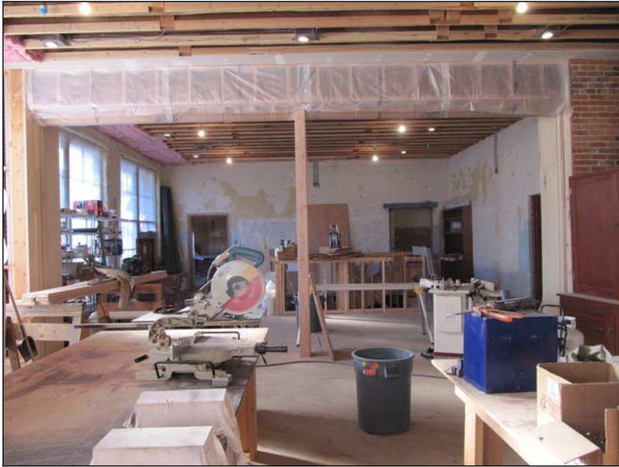
Looking south in center classroom on first floor in 2015
