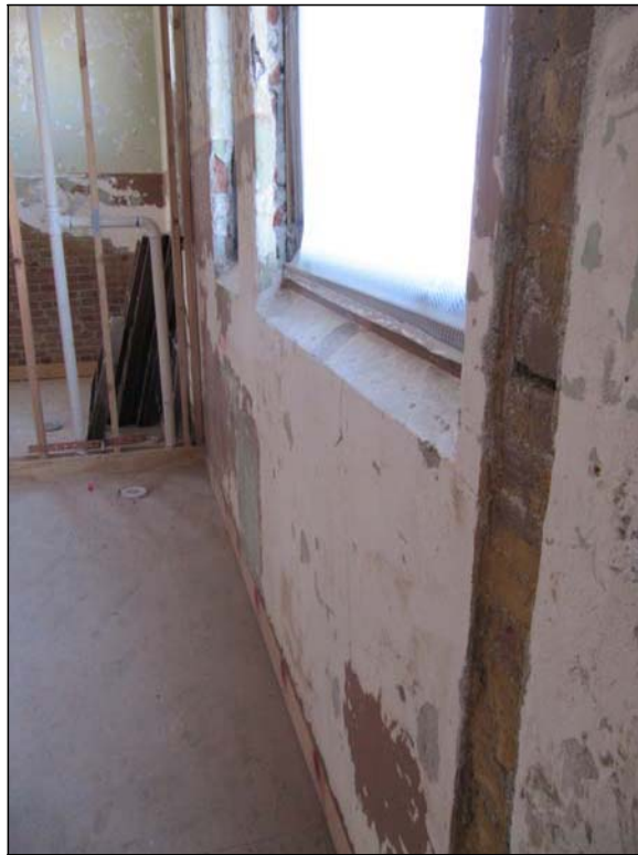
Window sill detail in 2015
