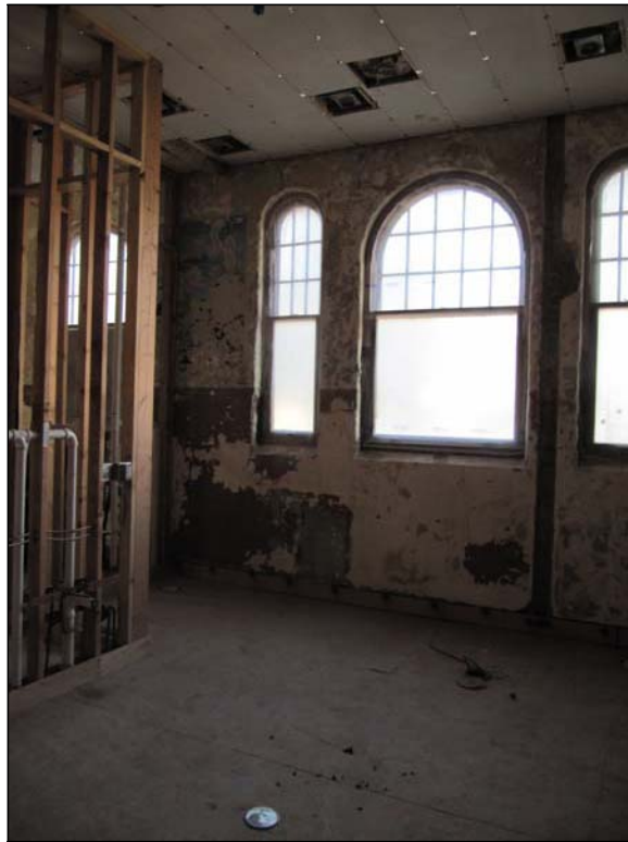
Looking west in southwest room on first floor in 2015
