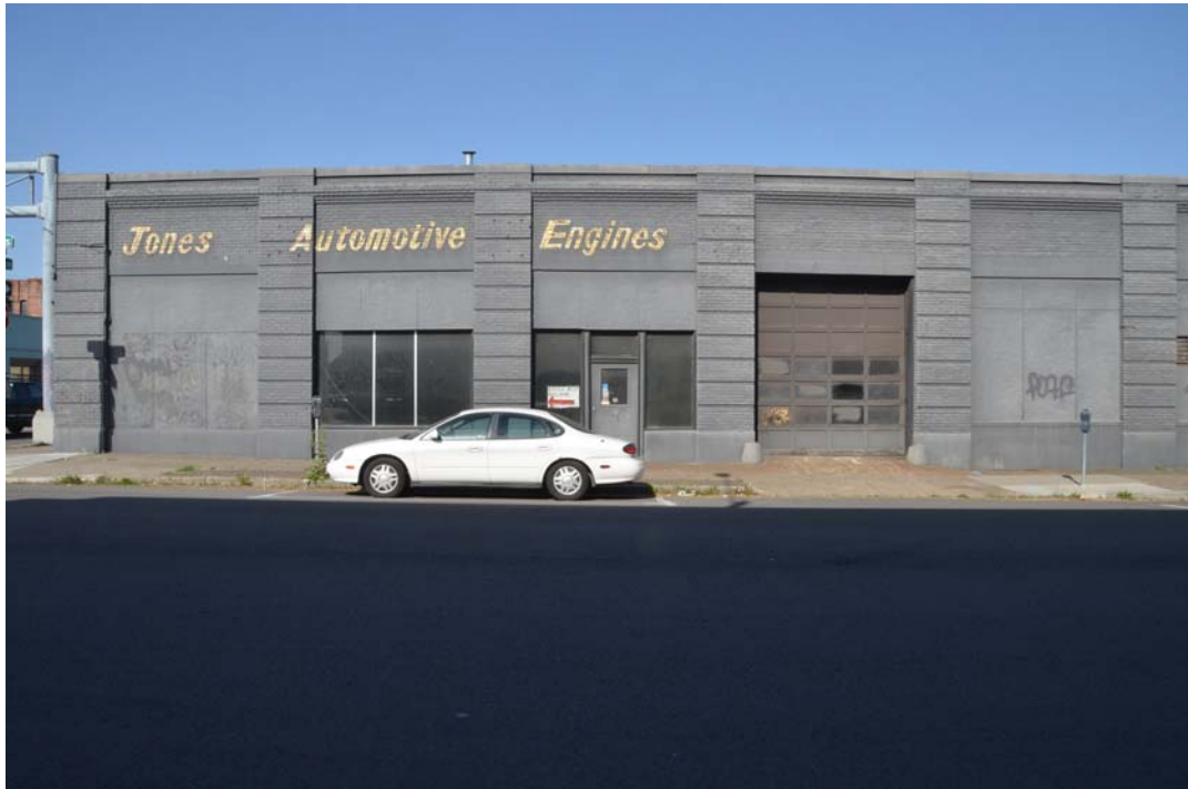
Photo 7 – Looking West Showing East Façade Bays 1 through 5
