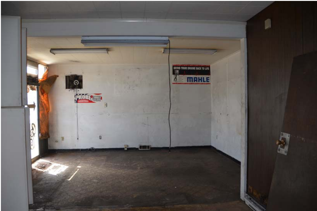
Photo 3 – Looking West Toward Main Entry on Front Facade
