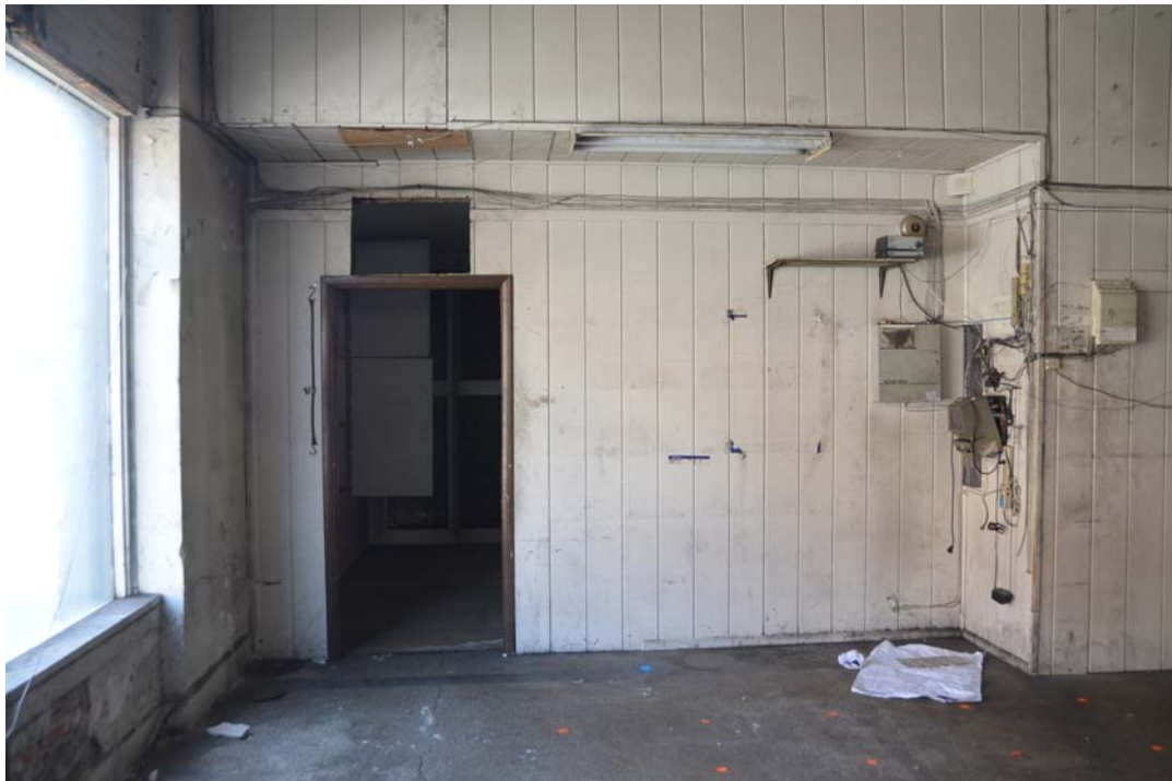
Photo 4 – Looking South Toward Front Office (SE Corner of Building)
