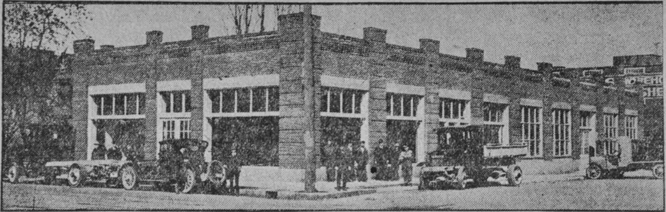
New House for Truck Firm.
