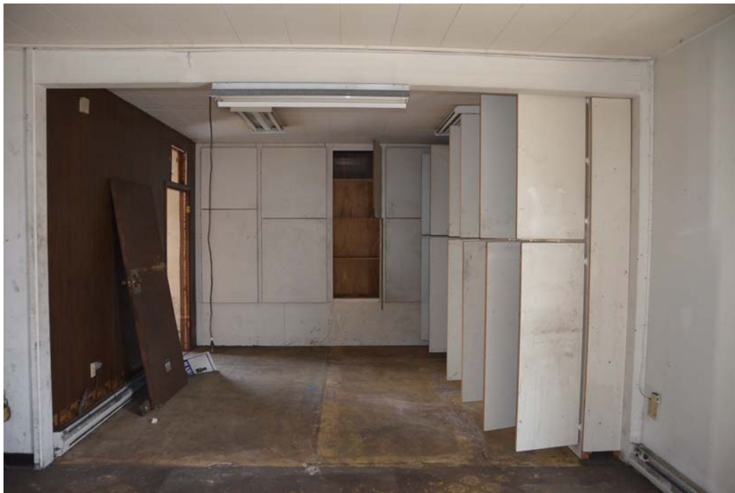
Photo 2 – Looking East Toward Showing Front Office (Bay 1 Covered)
