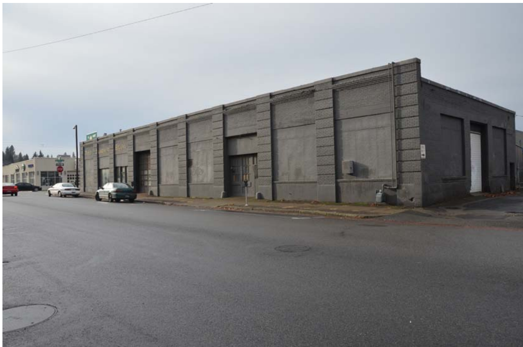
Photo 4 – View to Southwest Showing East Façade, Rear Façade
