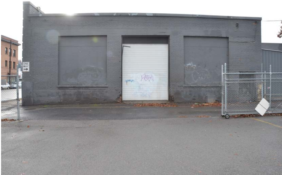
Photo 5 – Looking South at Rear (North Façade)
