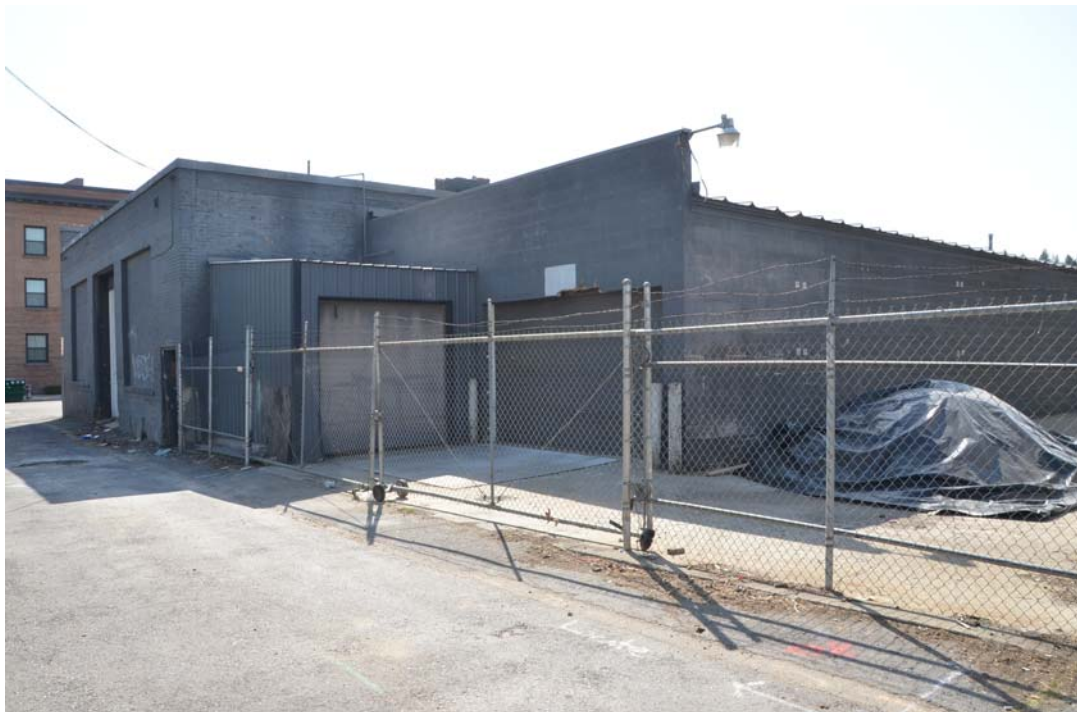
Photo 6 - View to SE Showing Rear Façade (northwest corner) and West Side Addition
