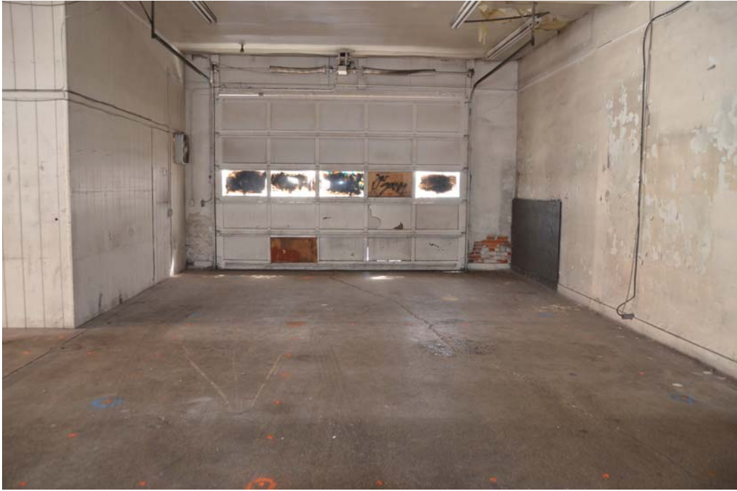
Photo 5 – Looking South Toward Truck Door in Front Façade (SW Corner)
