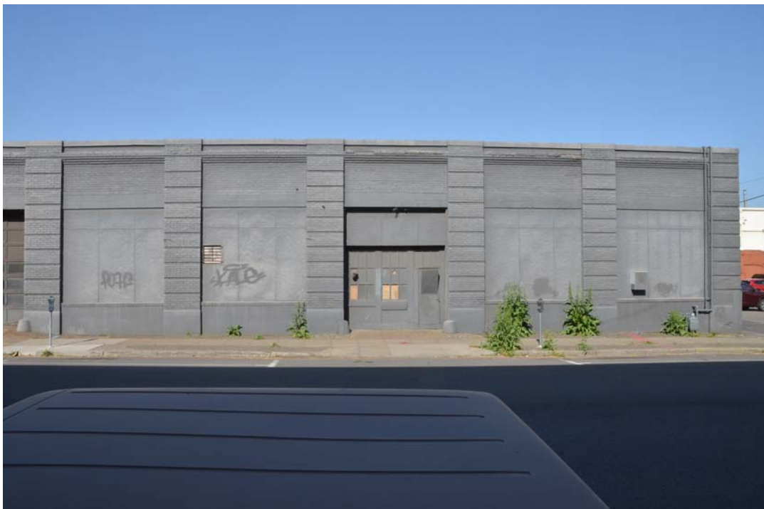
Photo 8 - East Façade, North End Showing Bays 5 through 9
