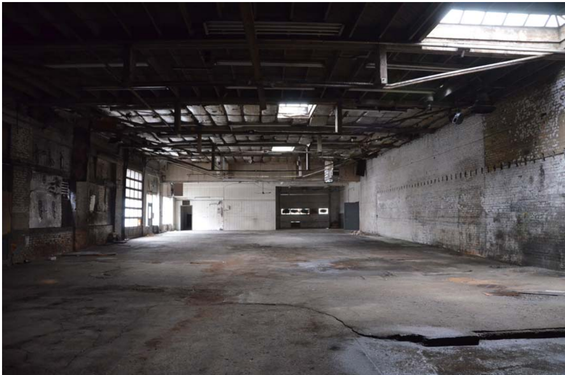
Photo 8 – Looking South Across Shop Floor Toward Front Office
