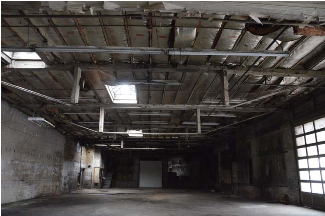
Photo 6 – Looking North Toward Rear of Building Showing Shop Area
