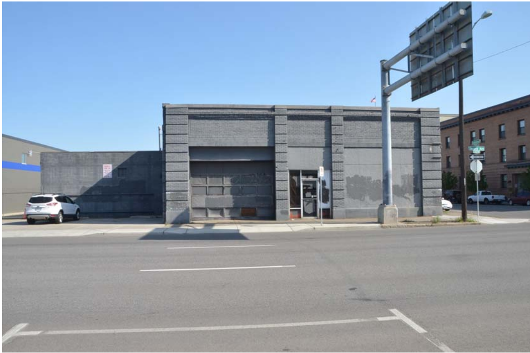
Photo 1 – View to North Showing Front Façade of 1302 West 2 nd Avenue (Building Built ca. 1921; Addition 1980)
