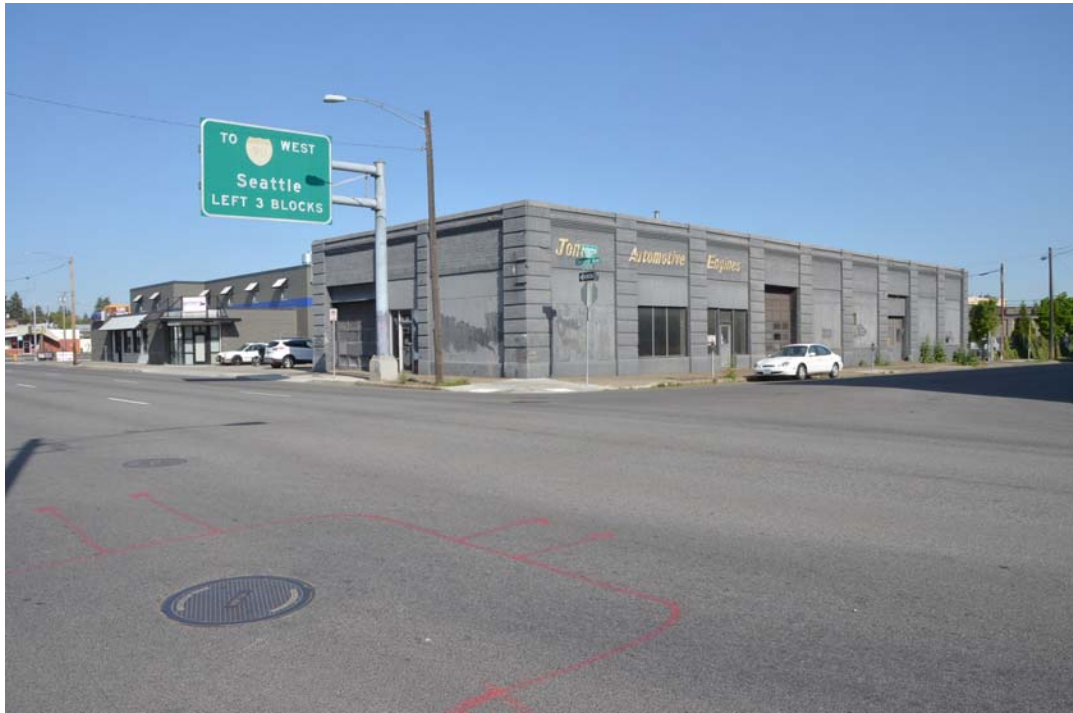
Looking NW at Jones Automotive Context Before Remodel
