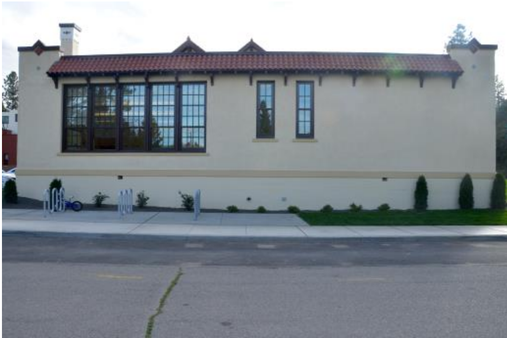
Photo 12 – Looking South at North Façade of 1930-31 Addition
