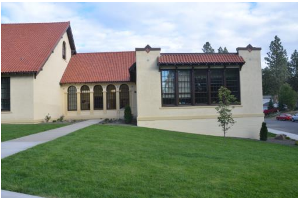
Photo 6 – Looking East at South End Showing 1930-31 Wing
