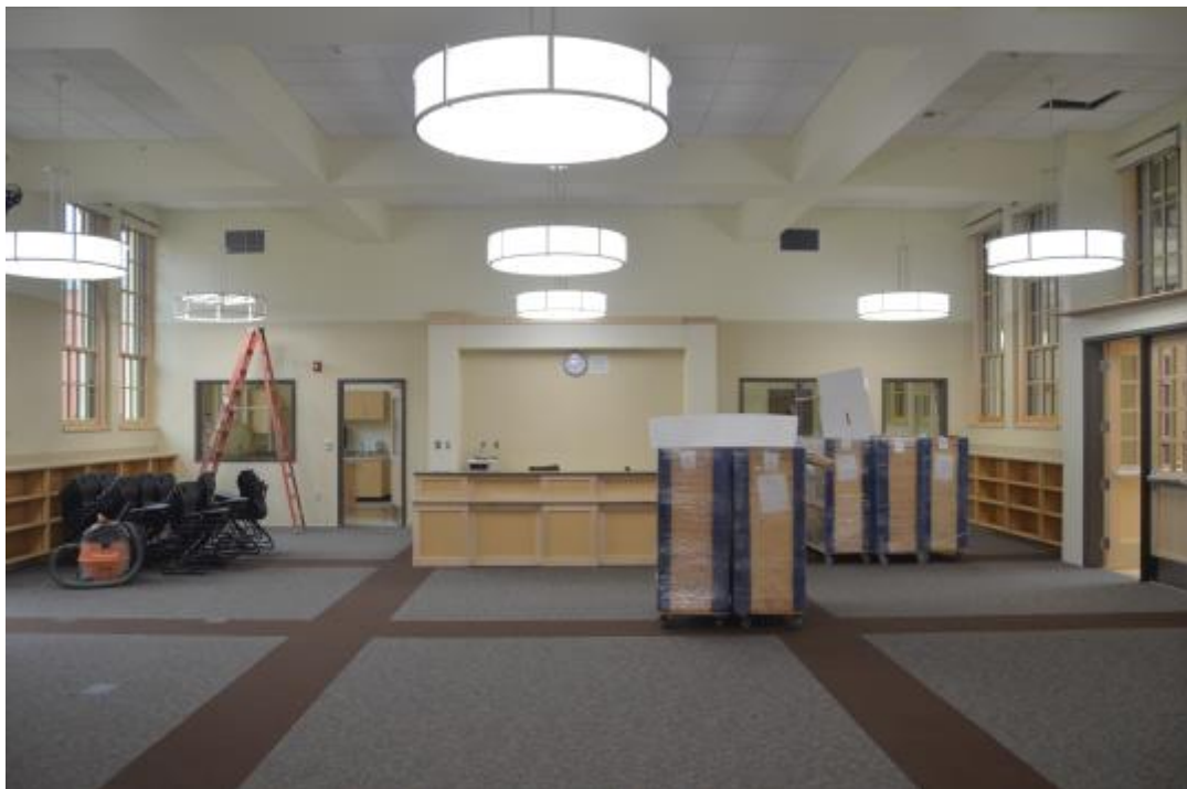
Photo 6 – Looking East at Library Toward Stage (Former Multi-purpose-Gymnasium)
