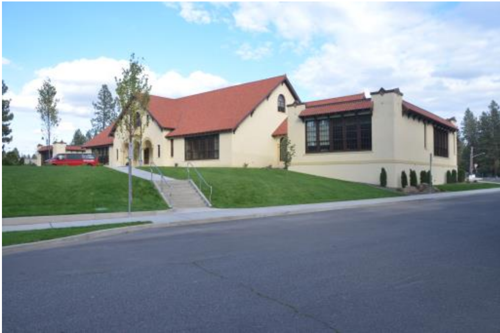
Photo 5 – Looking NE at SW Corner of Building – 1930-31 Wing
