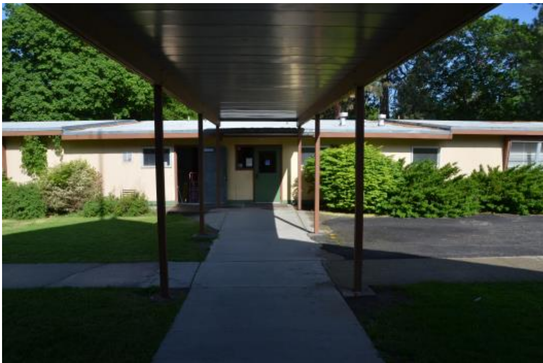
Photo 22 - Looking West at Covered Walkway Connecting 1956 Classroom Unit and 1921 Main Building
