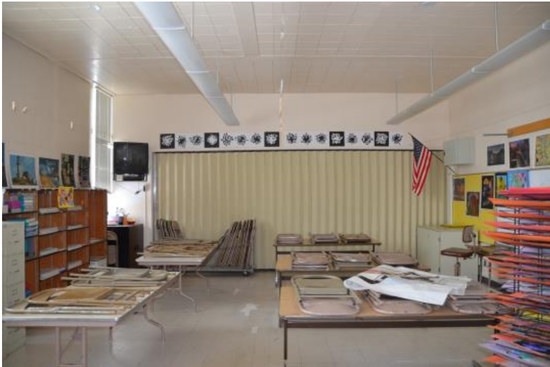
Photo 27 – Looking West Across Classroom 142 in 1949 Wing
