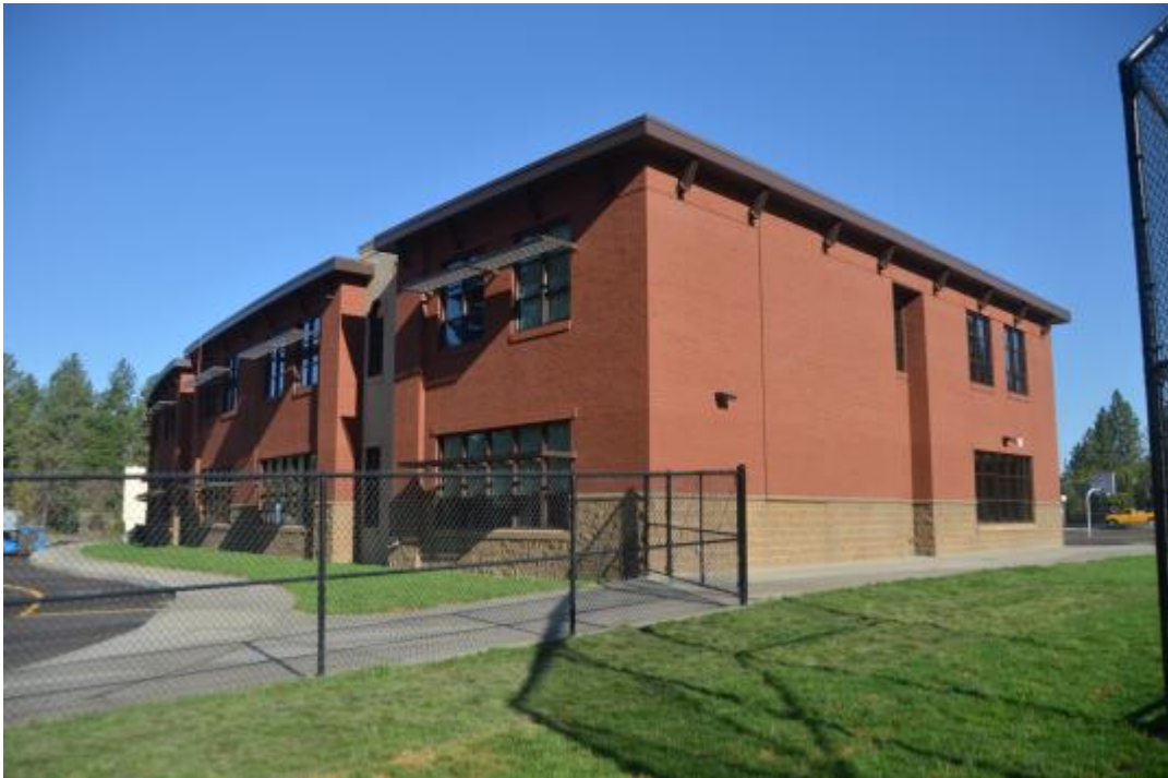
Photo 9 – Looking West at Southeast Corner of 2015 Addition
