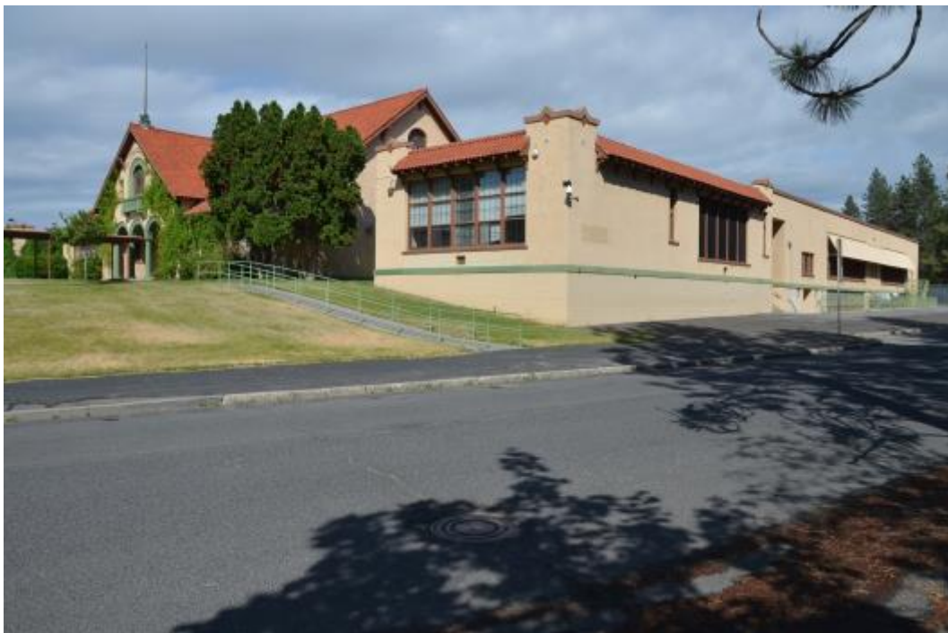
Photo 16 - SW Corner of 1931 Addition, 1949 Addition to East
