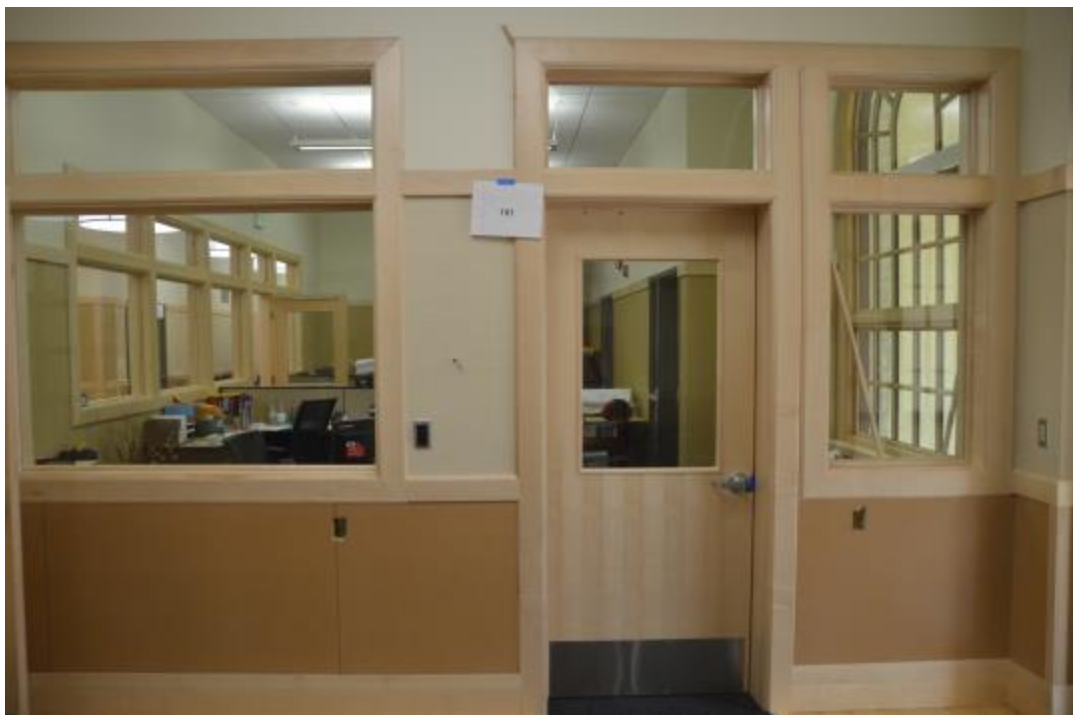
Photo 2 – Looking West Toward Reception-Office From Entry Vestibule
