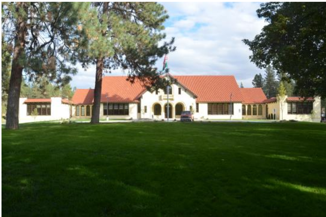
Photo 2 – Looking East at Main Façade-1921 Building & 1930-31 Additions
