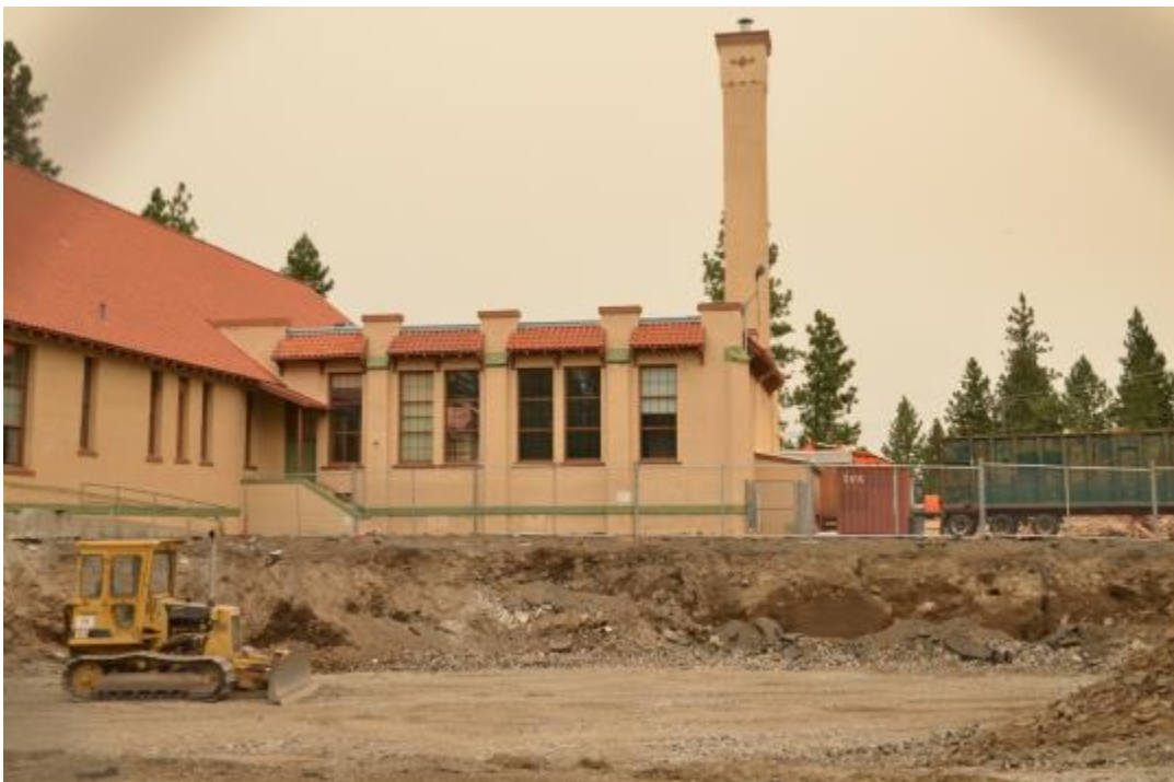
Photo 26 – Looking North at West Side of Gymnasium During Demolition – 7/17/2014
