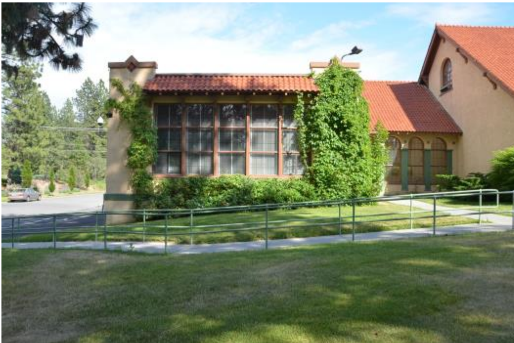
Photo 4 - Looking East at 1930-31 Classroom Wing Addition (NE Corner) of Hutton School
