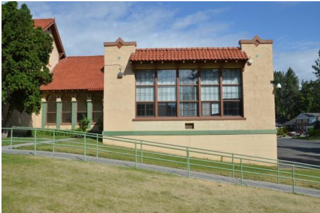
Photo 14 - Looking East at 1931 Classroom Wing (South End)
