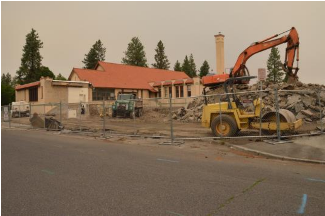
Photo 23 – Looking NW at SE Corner of School During Demolition – 7/17/2014
