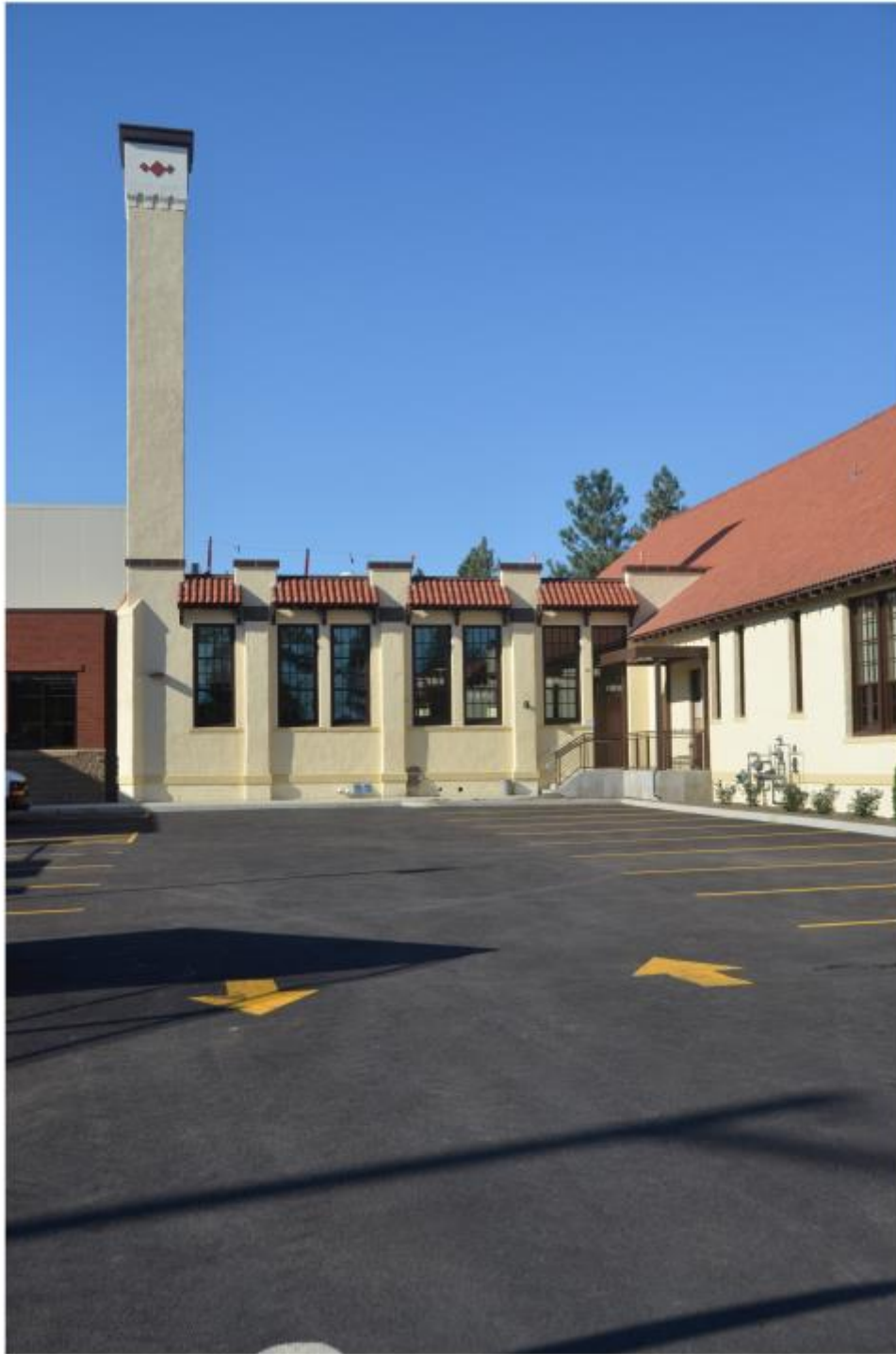
Photo 11 – Looking South at North Façade of 1930-31 Gymnasium/Multipurpose
