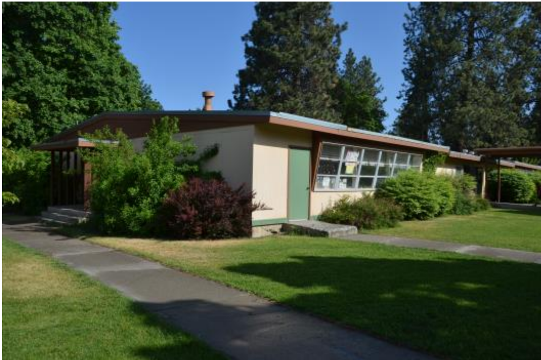
Photo 21 - Looking NE at 1956 Classroom Unit
