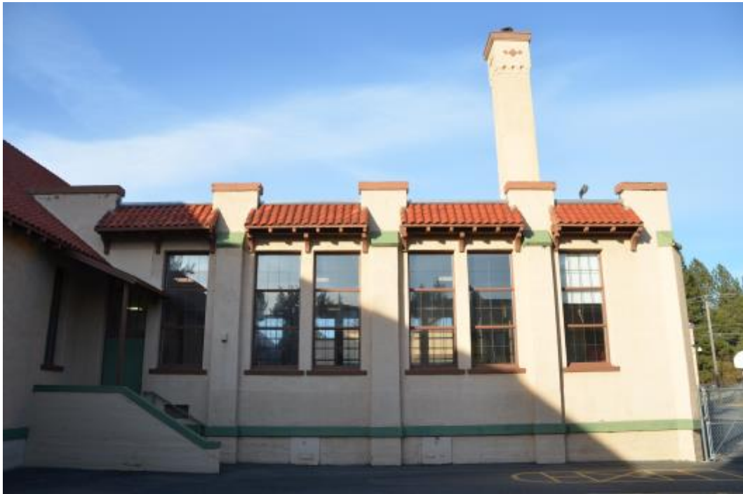
Photo 9 - Looking North at 1931 Gymnasium/Auditorium Addition, West Facade
