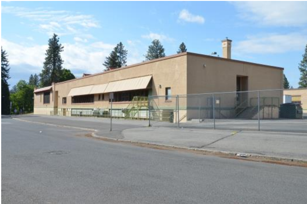
Photo 17 - Looking NW at 1949 Addition SE Corner of South Wing
