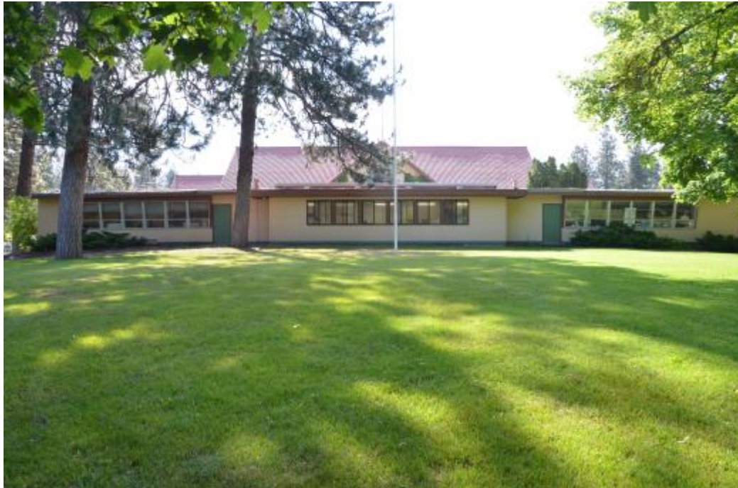
Photo 2 - Looking East at 1956 Classroom Unit in Front of 1921 Wing of Hutton School
