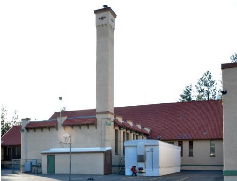
Photo 11 - Looking West at Rear of 1930-31 Gymnasium/Auditorium, NE Corner
