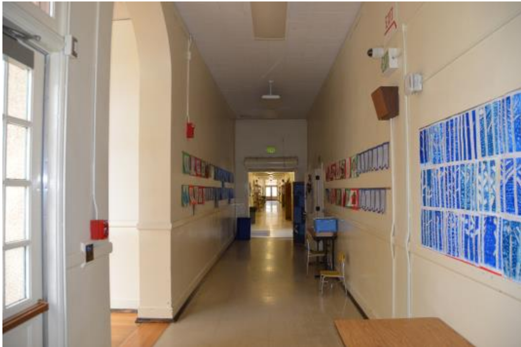
Photo 23 – Looking East Along 1930-31 South Hallway Toward 1949 Wing
