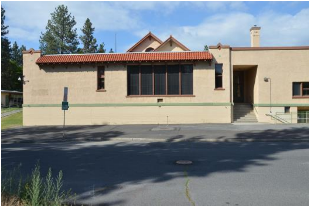
Photo 15 - Looking North at SW Corner, South Façade of 1930-31 Addition (At Juncture with 1949 Addition)
