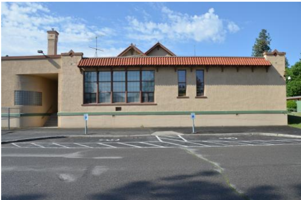
Photo 6 - North Façade of 1931 Addition, Juncture with 1949 Addition to East
