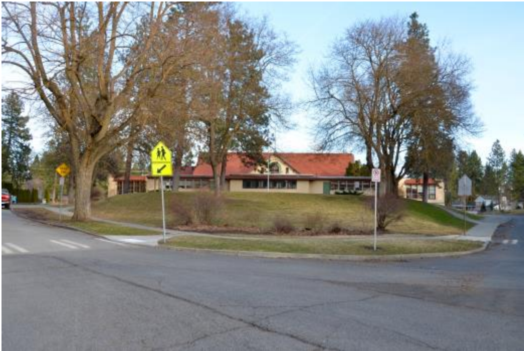
Photo 1 - West End of Hutton School Site at East 24 th Avenue & Plateau Road
