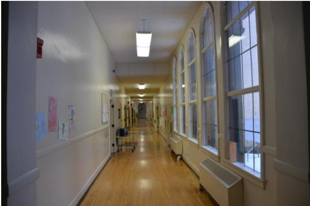
Photo 9 – Looking South Along Main Hallway From North End
