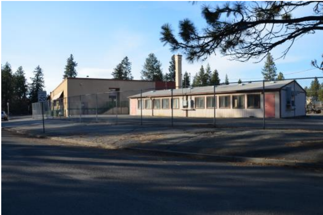
Photo 19 - Looking West at Portable Unit near East End of 1949 South Wing
