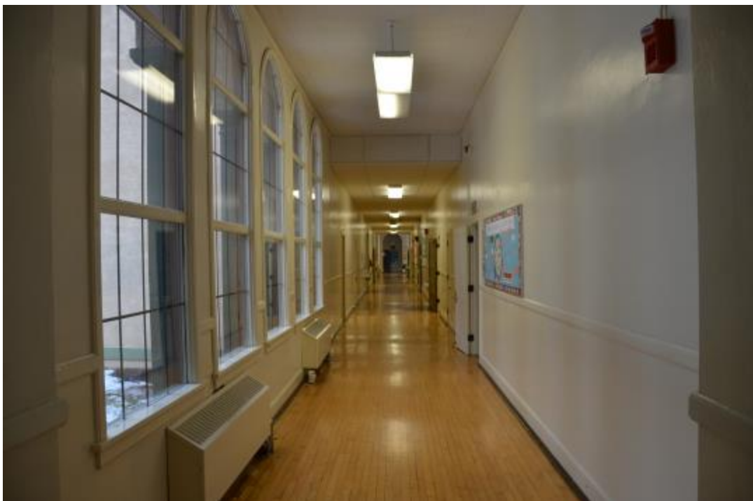
Photo 10 – Looking North Along Main Hallway From South End
