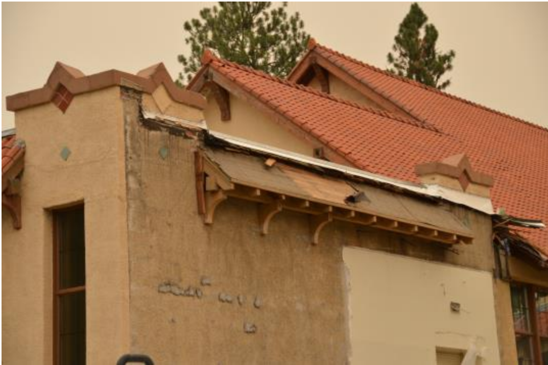
Photo 25 – Looking NW at SE Corner of 1930-31 Wing During Demolition – 7/17/2014
