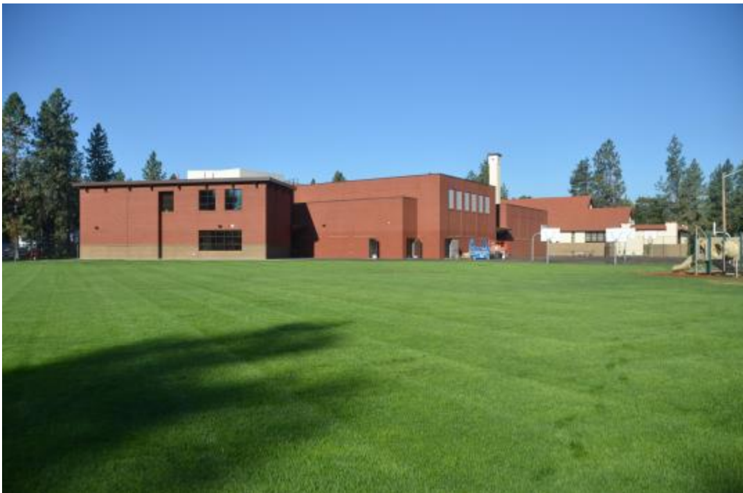
Photo 10 – Looking West at Rear of 2015 Addition and Historic Hutton School
