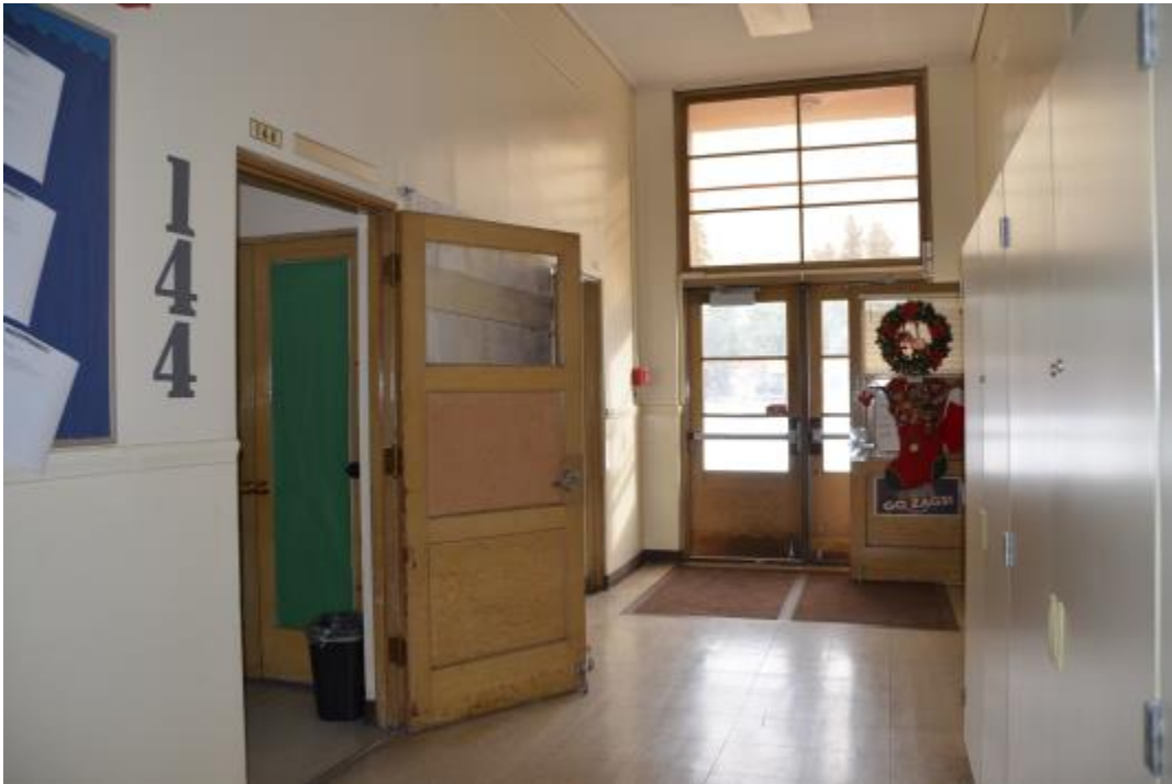
Photo 25 – Looking East Along Hallway in 1949 Wing to Room 144
