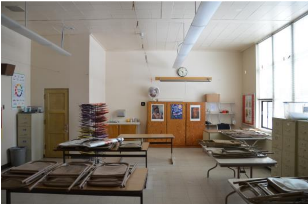
Photo 28 – Looking East Across Classroom 142 in 1949 Wing
