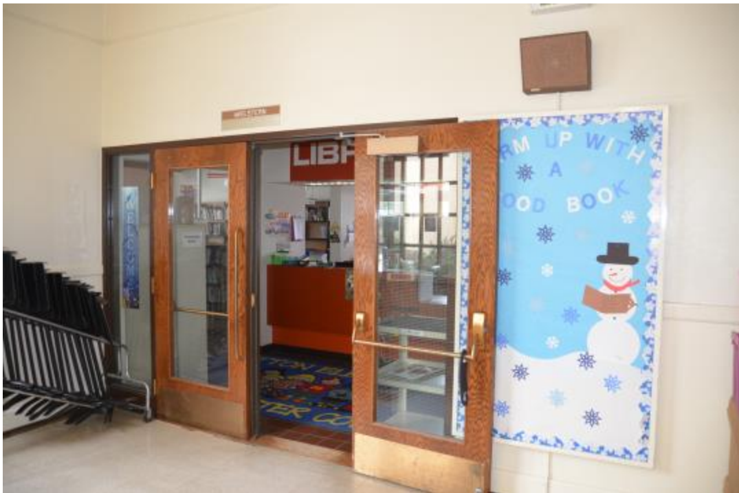
Photo 20 – Looking Northwest at Doors to Library in North End, 1930-31 Addition
