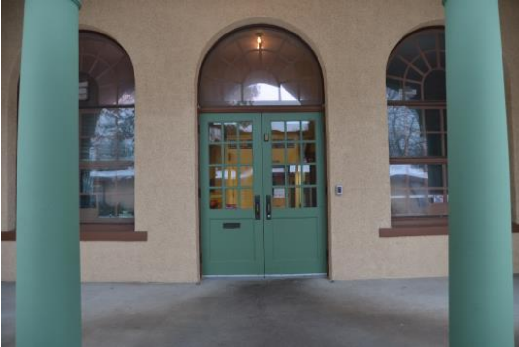
Photo 1 – Looking East at Front Entry of 1921 Building
