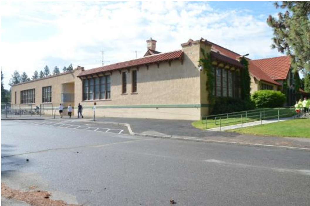
Photo 5 - Looking SW at NE Corner of Hutton School (1930-31 and 1949 Additions)
