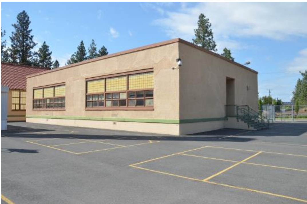
Photo 8 - Looking NE at 1949 North Wing Addition, West Facade
