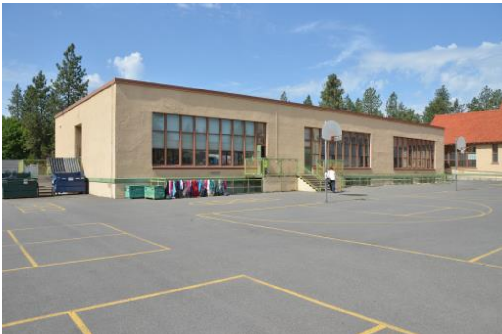
Photo 18 - Looking SW at 1949 Addition, North Façade of South Wing
