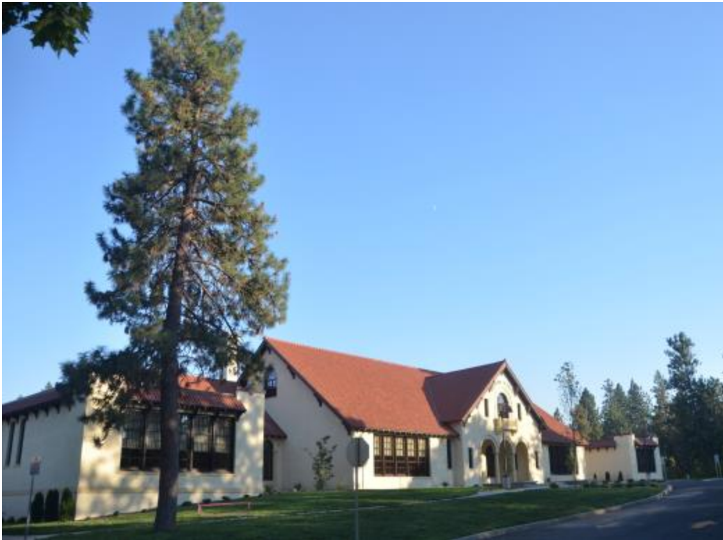
Photo 3 – Looking SW at NE Corner of Hutton School
