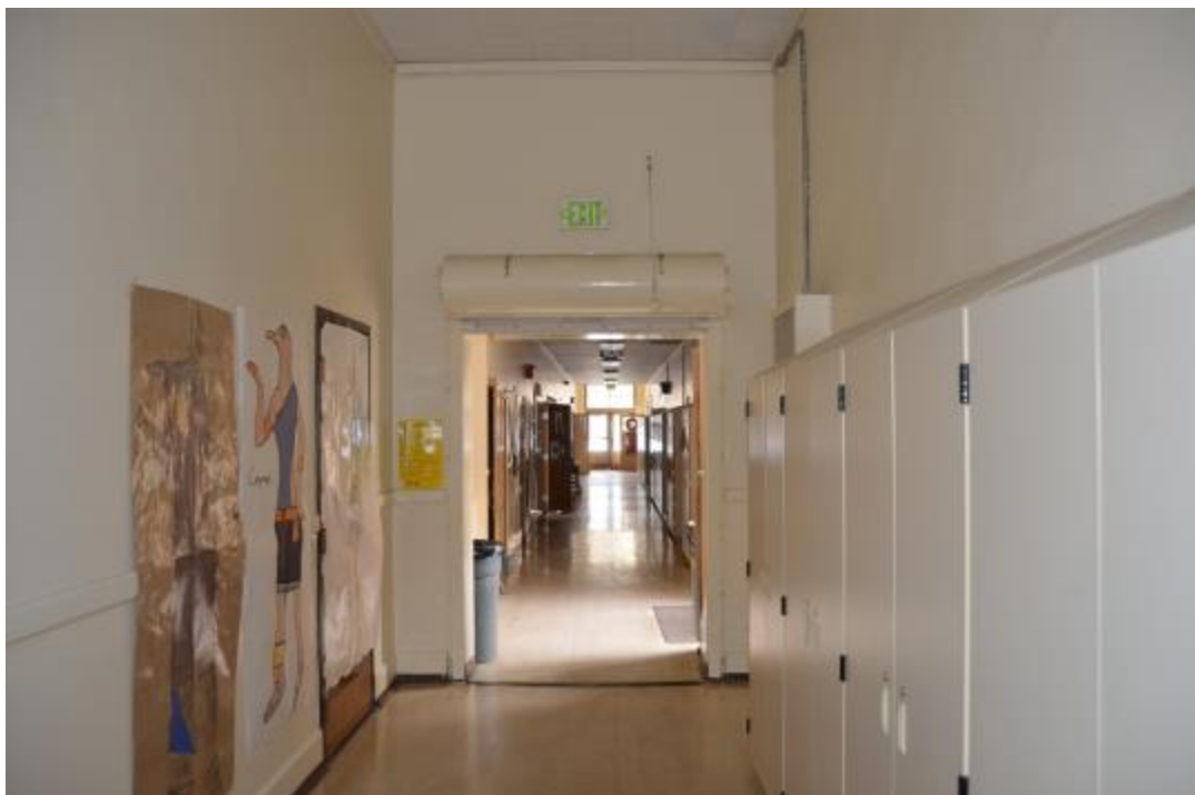
Photo 24 – Looking East Along 1930-31 North Hallway Toward 1949 Wing
