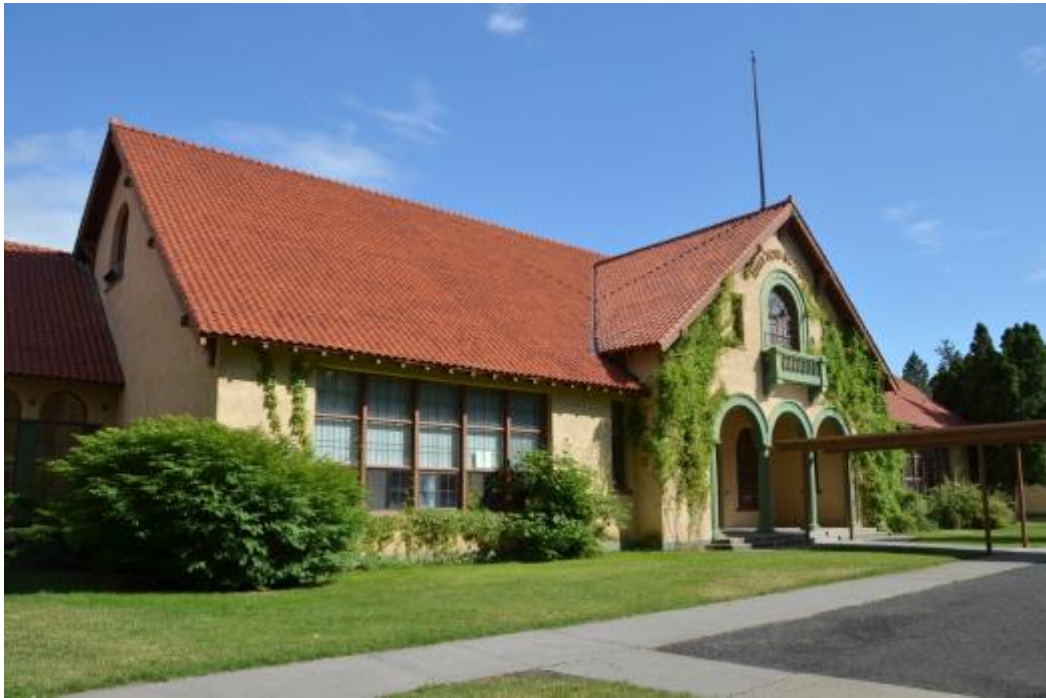
Photo 3 - Looking SE at Front (West Façade) of 1921 Wing of Hutton School
