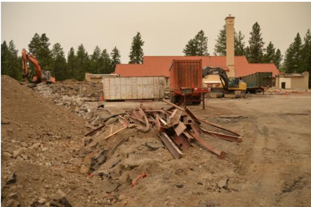
Photo 24 – Looking West at Rear of School During Demolition – 7/17/2014
