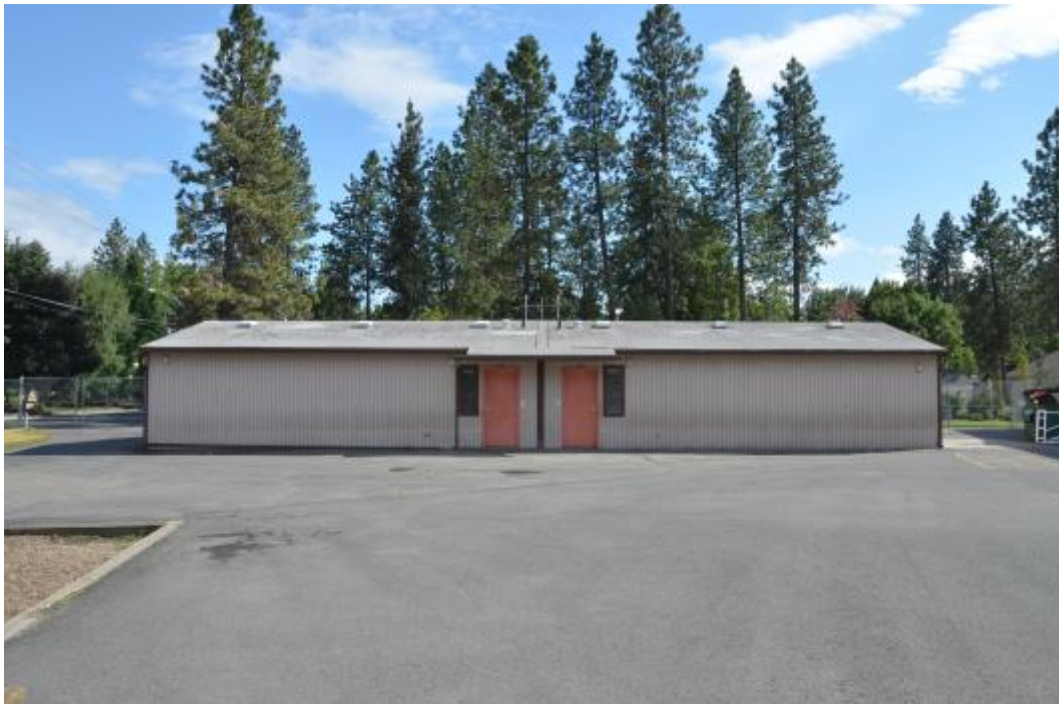
Photo 20 - Looking North at Portable Unit East of 1949 South Wing
