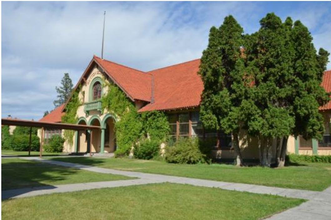
Photo 13 - Looking NE at 1921 Classroom Building-Covered Walkway to 1956 Unit
