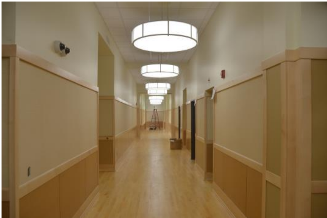
Photo 3 – Looking North Along Central Hallway of Original 1921 Building
