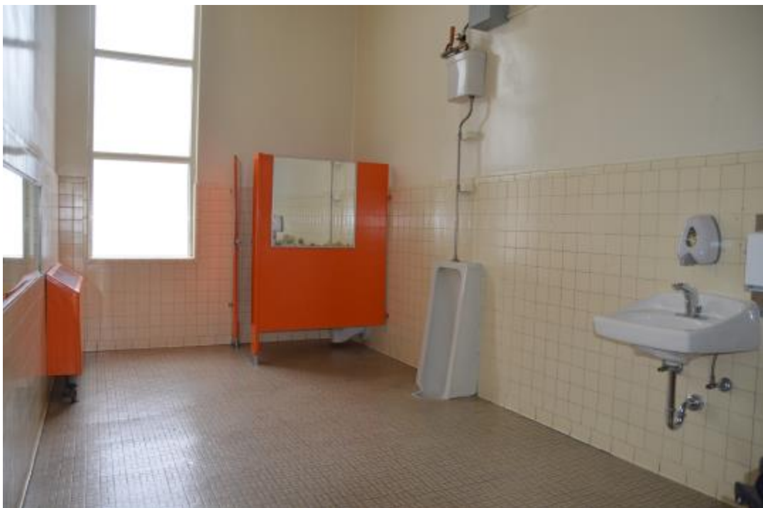
Photo 30 – Looking at Boys Restroom in 1949 Wing
