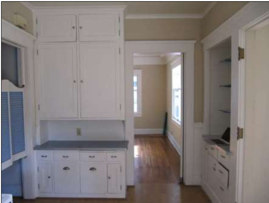
Kitchen in 2015, looking south into dining room
