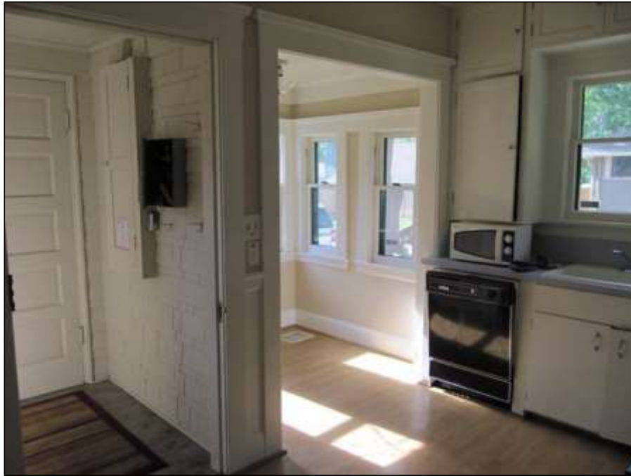
Kitchen in 2015, looking northwest into backyard
