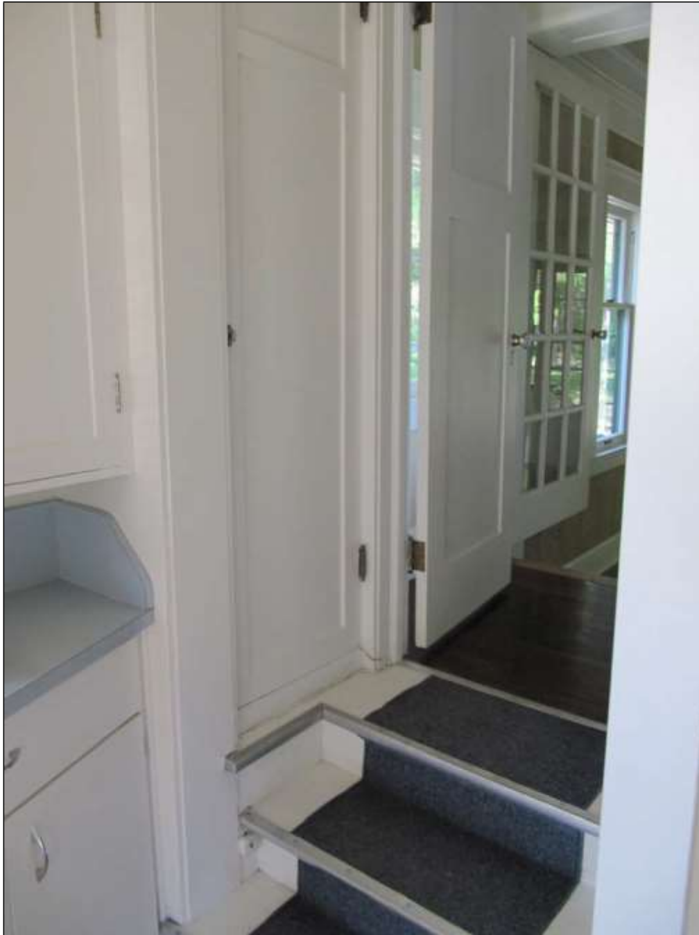
Stairs from kitchen to landing in 2015, looking northeast into living room
