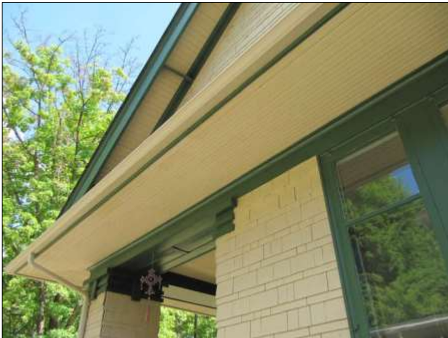
Northeast corner at roof in 2015
