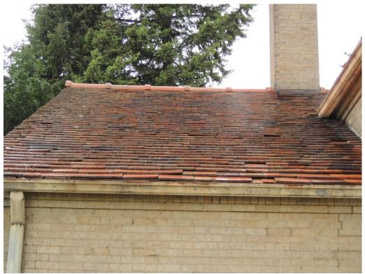
Photo 7: Red glazed barrel-shaped ceramic tiling of the roof (June 3, 2015)
