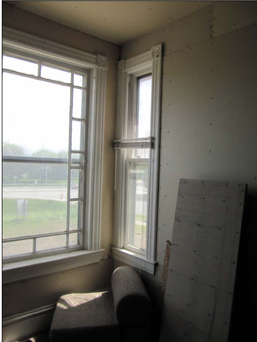
Southeast corner bedroom window on second floor in 2015.
