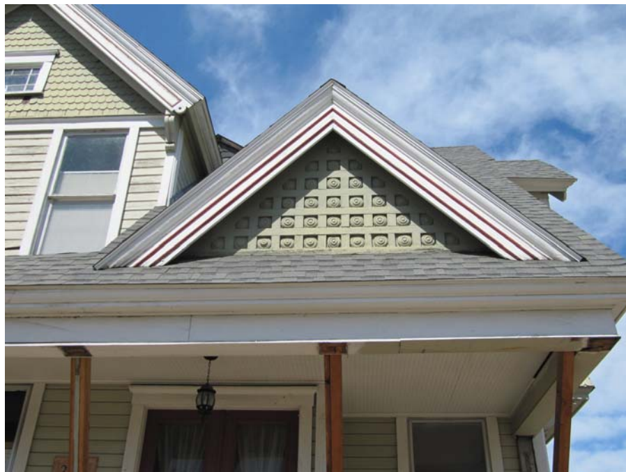
South façade porch gable peak in 2015
