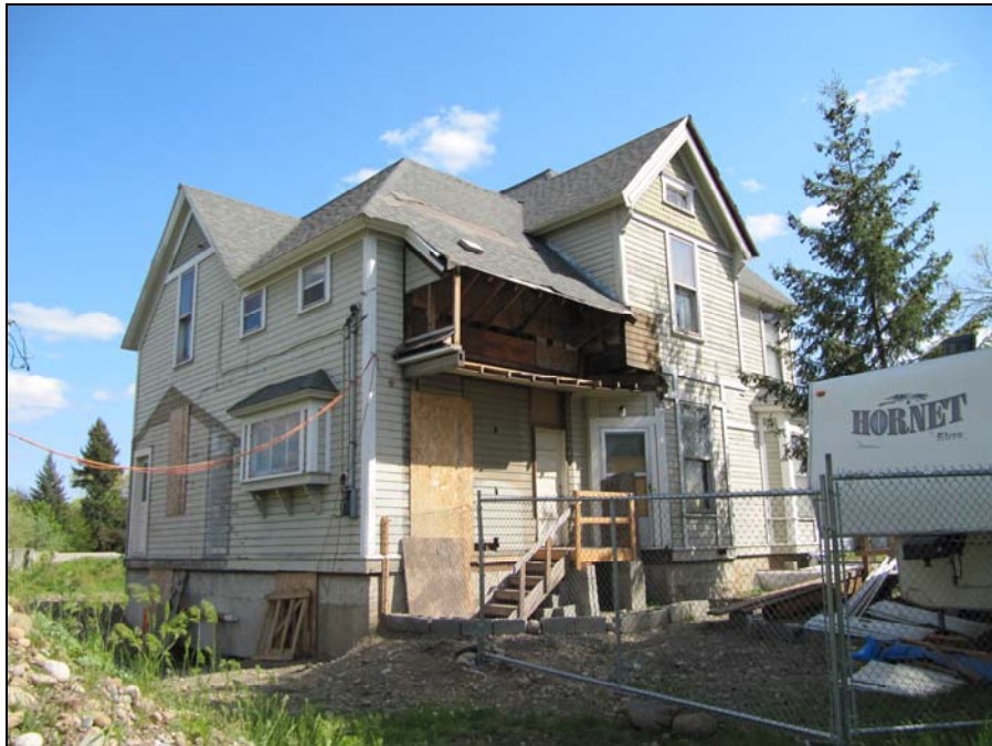
North rear and west elevations in 2015
