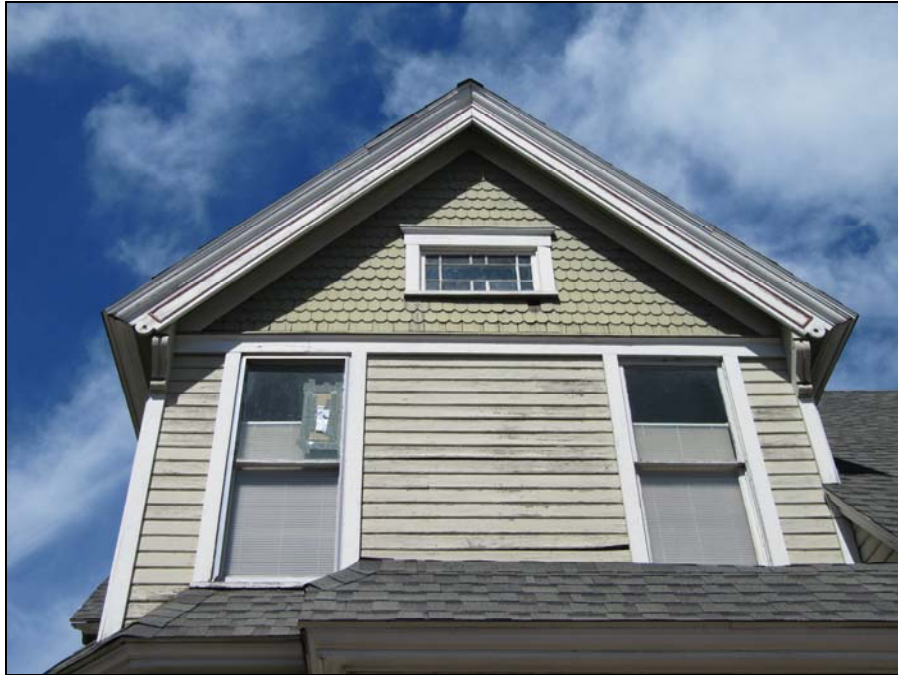
South façade gable peak in 2015
