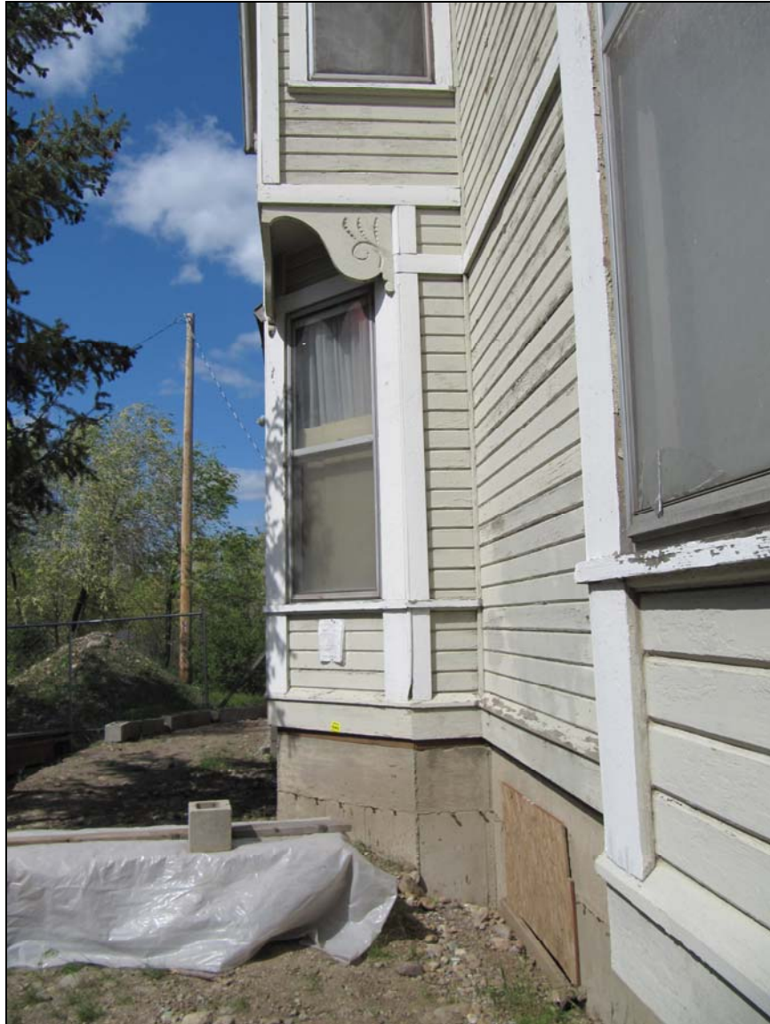
Cut-away window and decorative scroll-sawn brackets on west elevation in 2015.
