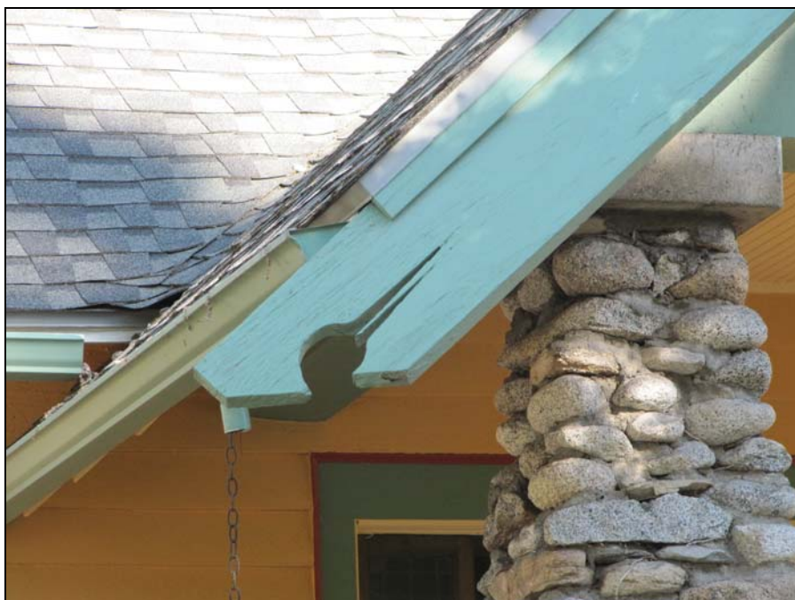
Front porch bargeboard in 2015
