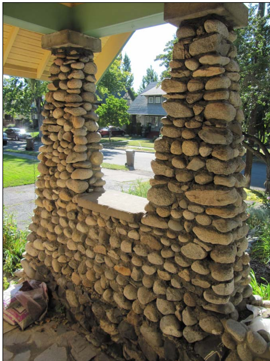
Cobblestone front porch pillar in 2015, looking west
