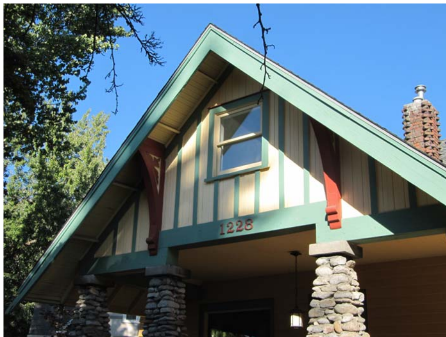
Front porch gable roof in 2015
