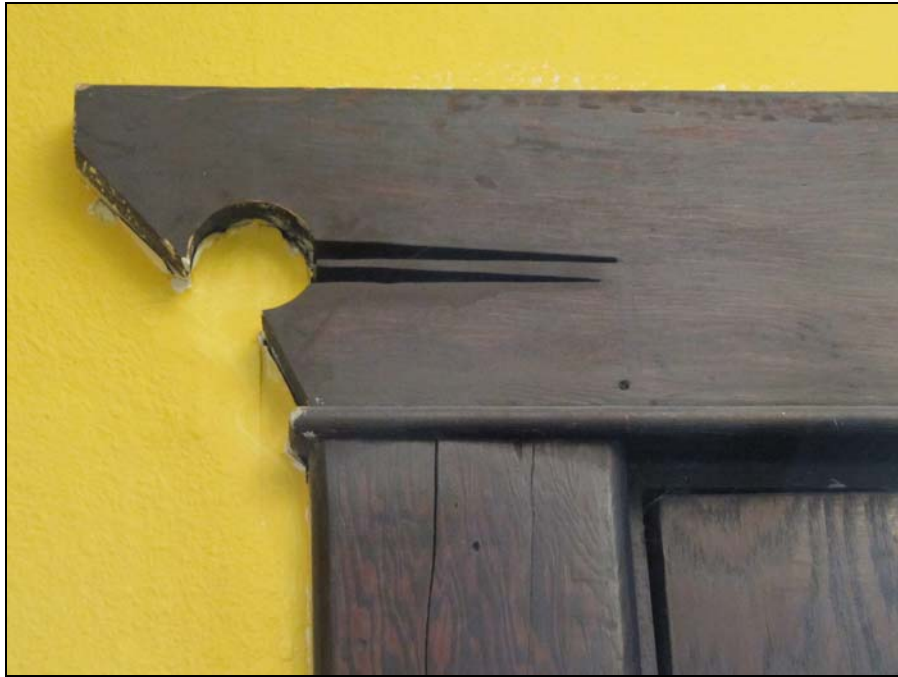
Interior door lintel in 2015
