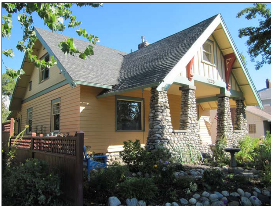
West façade in 2015
