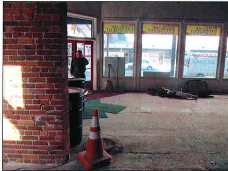
Bennett Block interior at 530 W. Main Avenue, looking west
