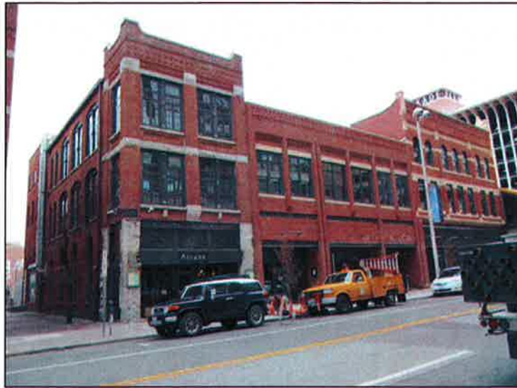
2014 Bennett Block west façade Lockhardt Building, Star Hotel, Bennett Building
