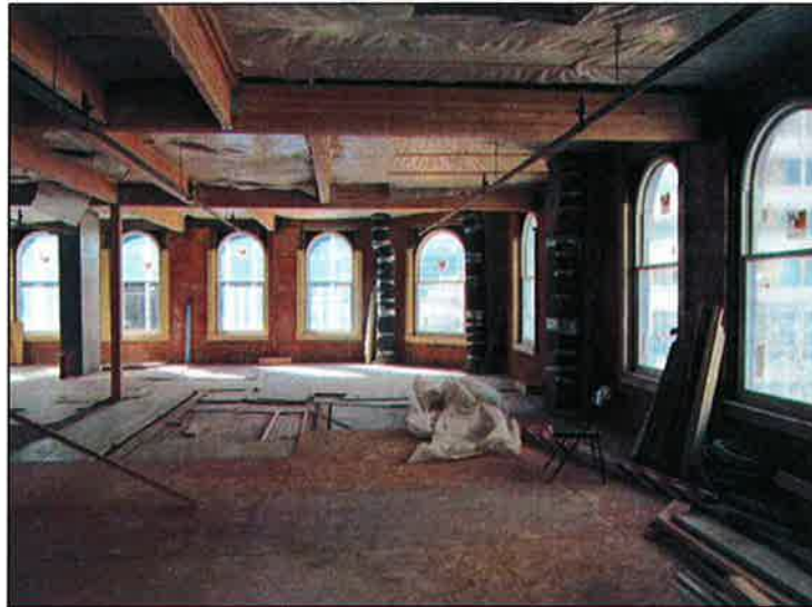
Bennett Block 3 rd floor, looking south in 2014
