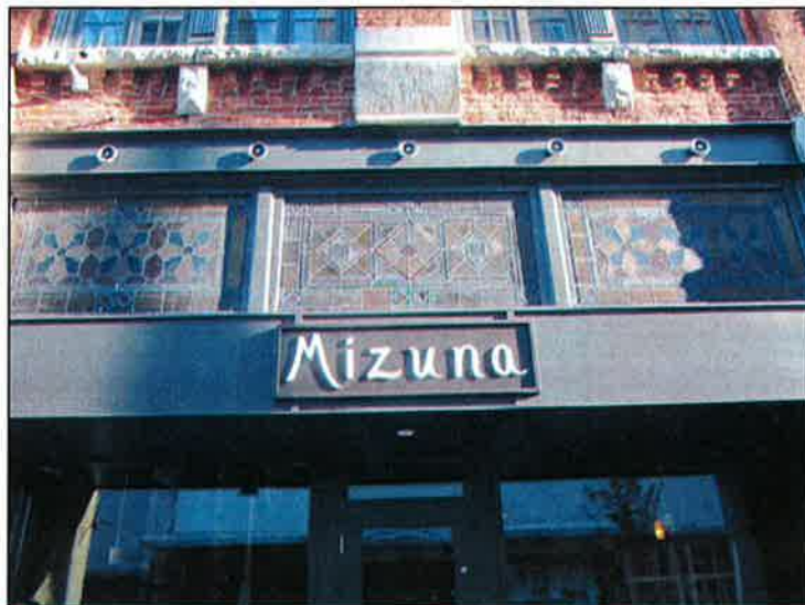
Lockhardt Building transom windows built in 1890
