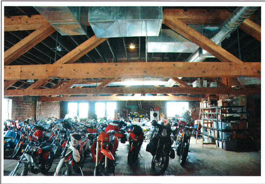
Photo 7 – Mezzanine Floor Looking North Toward Freight Elevator and Rear
