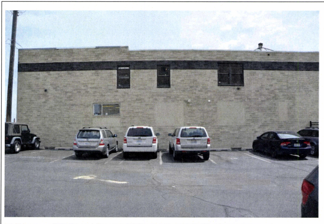
Photo 8 – View to East Showing West Side Facade
