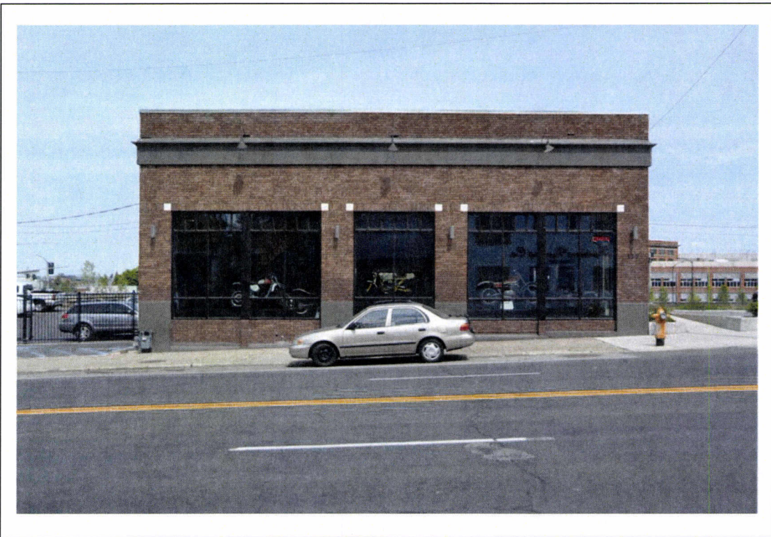
Photo 4 – View to North Showing Front Façade
