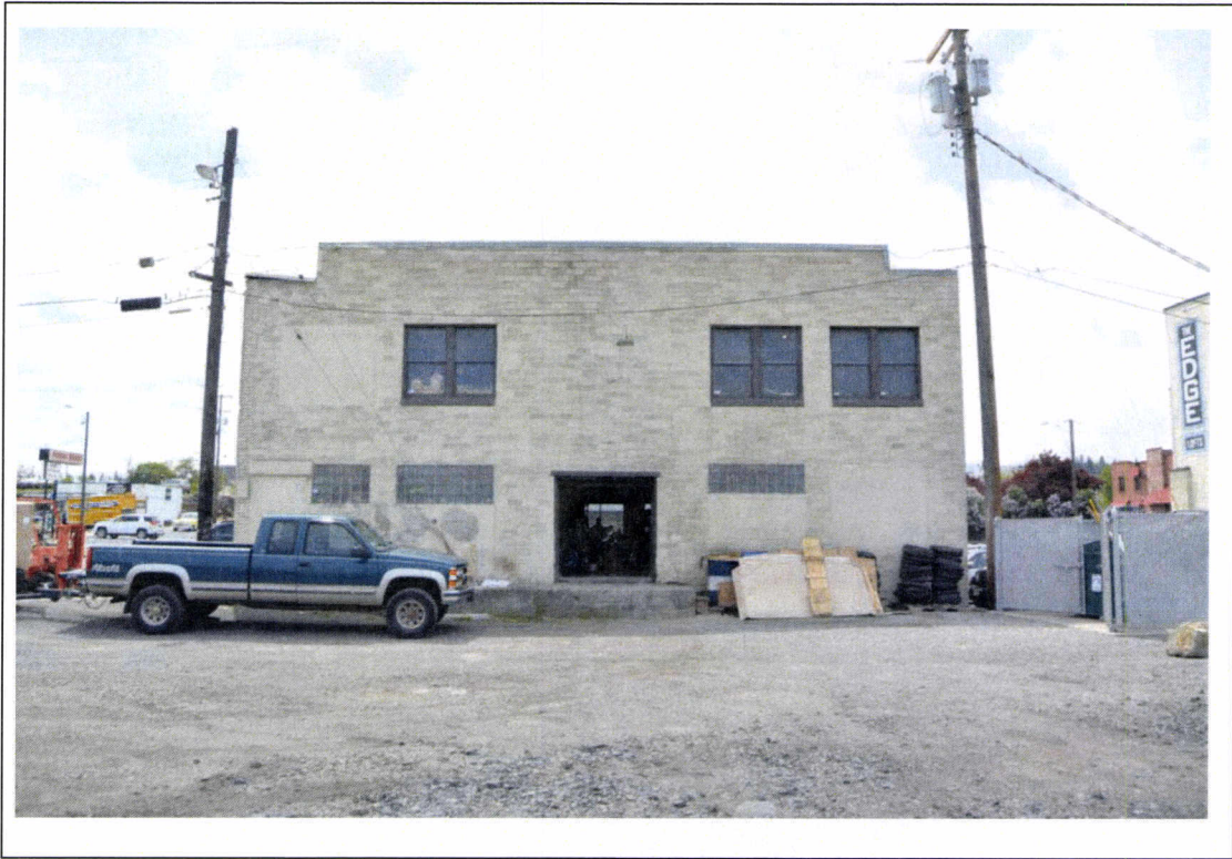
Photo 7 – View to South Showing Rear Facade
