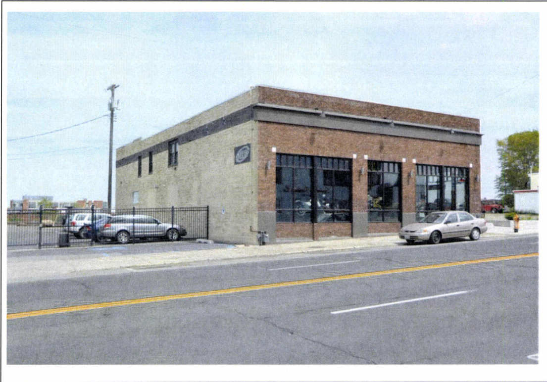
Photo 3 – View to Northeast Showing West and South Facades
