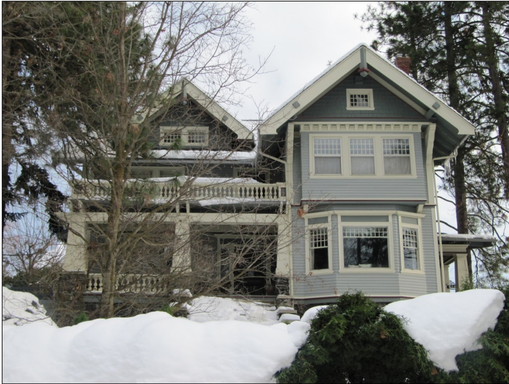
The historic Kroll House at 1249 S. Wall Street, Spokane, WA in 2011
