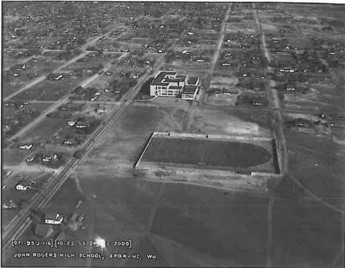
Bird's Eye view of John Rogers High School shortly after construction, October 1933.
