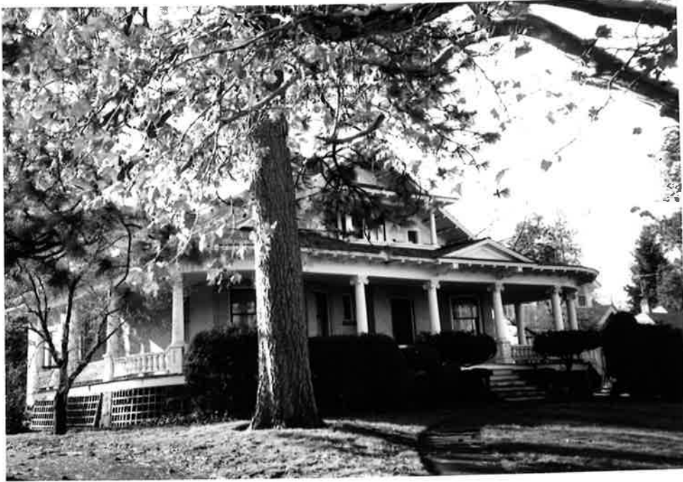
Photos 7 and 8 North facade elevation of Strack House in 2003.
