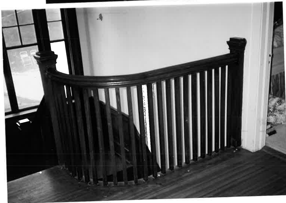
A. L. PORTER HOUSE Photos 13 and 14: Second-floor landing looking south down stairwell--1998 photos.
