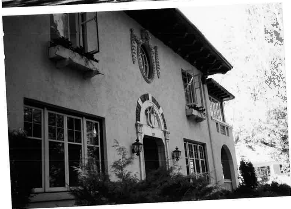
A. L. PORTER HOUSE Photos 1 and 2: North facade of house--photos taken in 1998.
