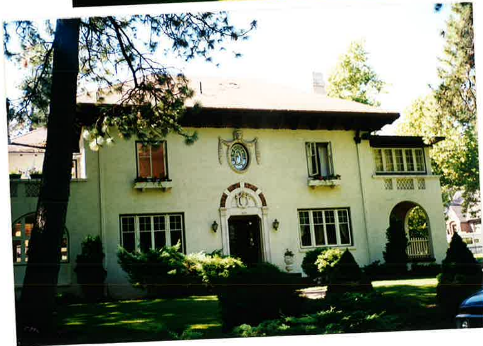
A. L. PORTER HOUSE Photos 2 and 3: North facade of house--photos taken in 1998.
