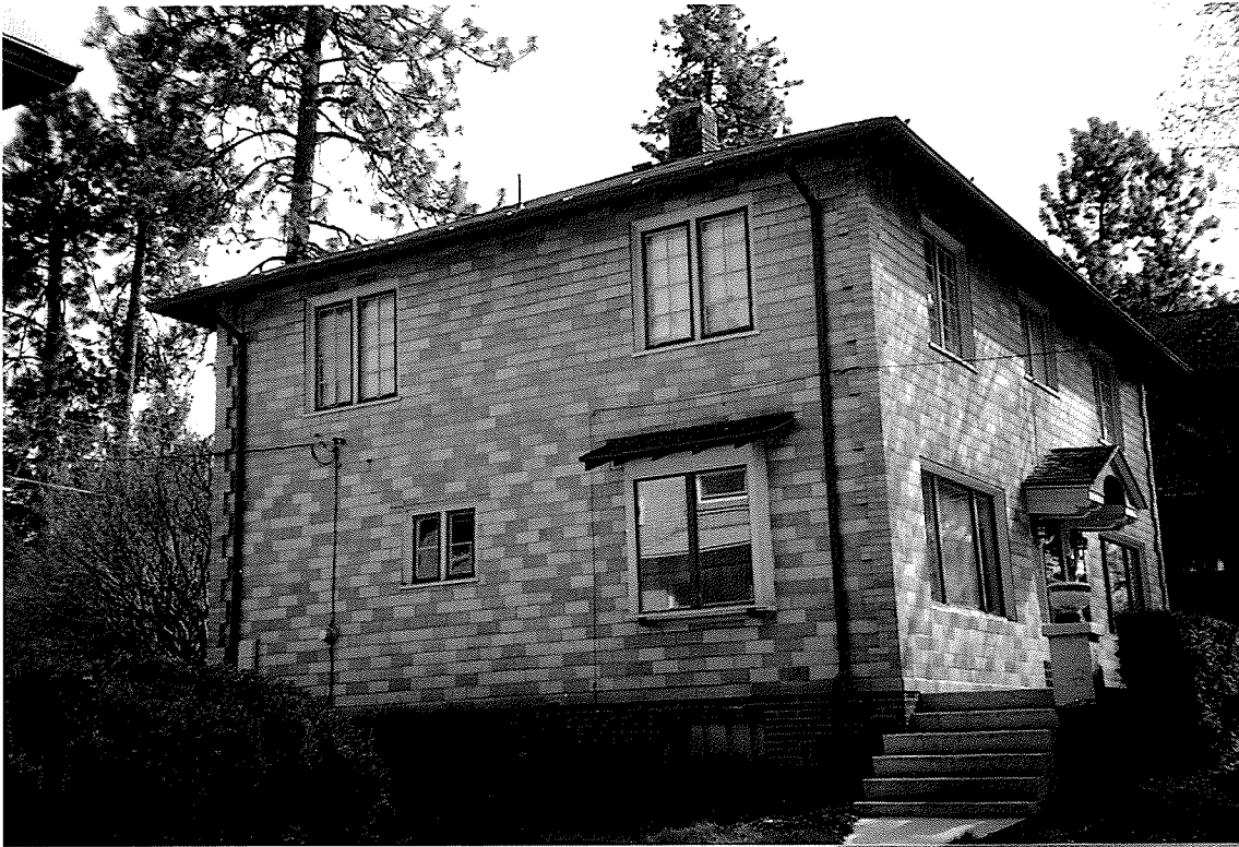
Photos 5 and 6 West elevation of house in 2008; detail of tile cladding and basement foundation.
