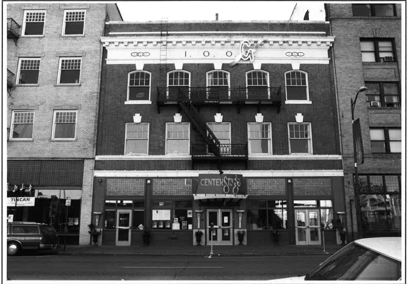
View to South of Front Facade
