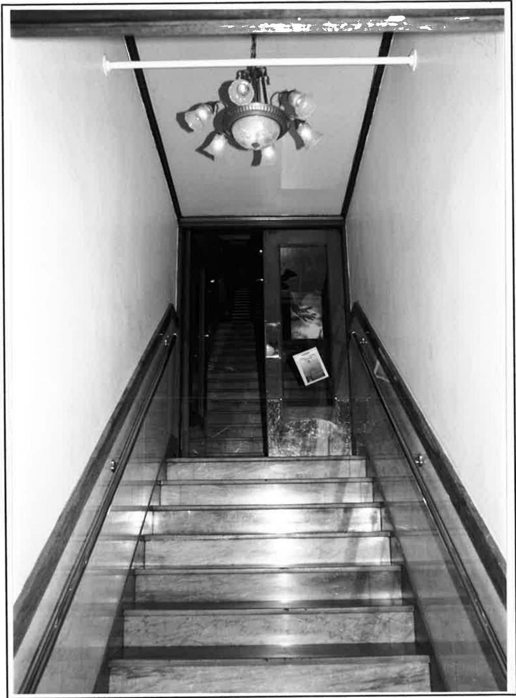
View to South Up Main Stairs to Second Floor
