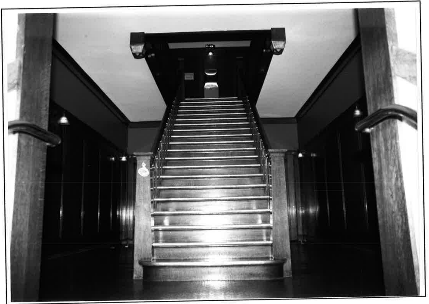
View to South - Second Floor Stair Landing Vestibule & Stairs to Third Floor
