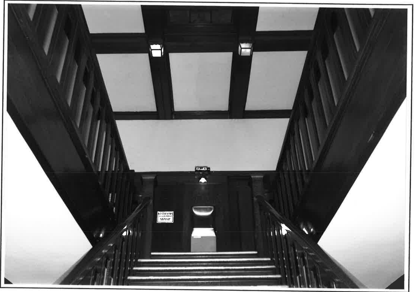
View to South - Approaching Thrd Floor Landing
