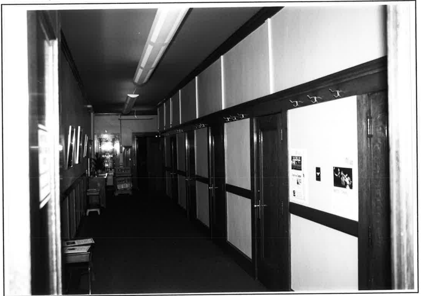
View to South- Second Floor Hallway to Lodge Hall (Offices and Storage Rooms and West Side)
