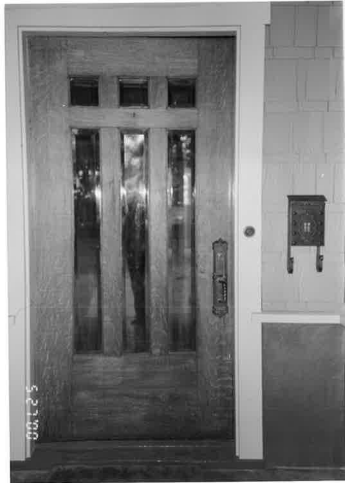
Front door from inside house, facing north.
