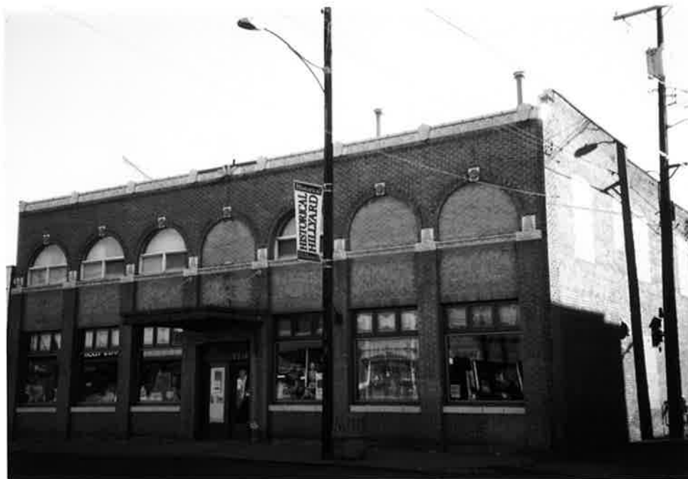
Photos 13 and 14 United Hillyard Bank Building; west façade.
