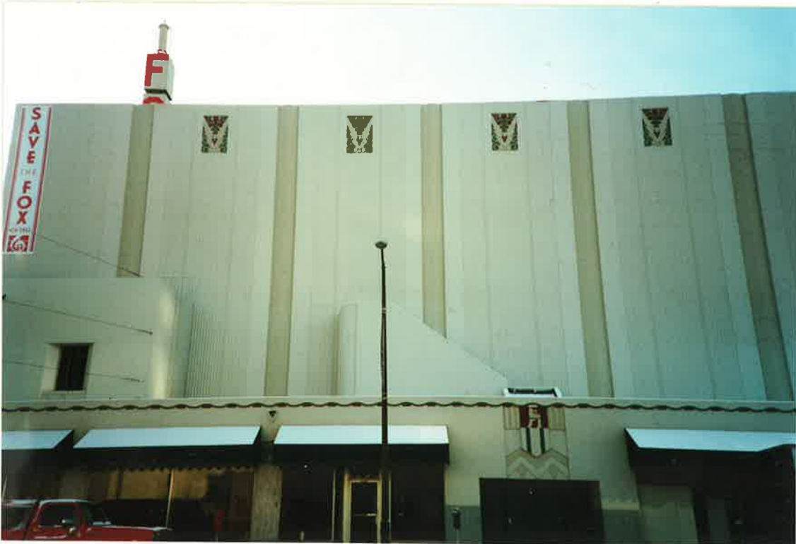
FOX THEATRE West Sprague facade
