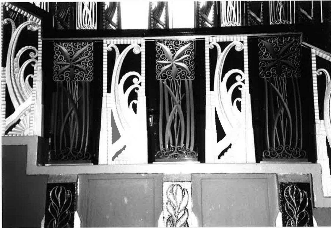
FOX THEATRE Aluminum and glass balusters Grand staircase
