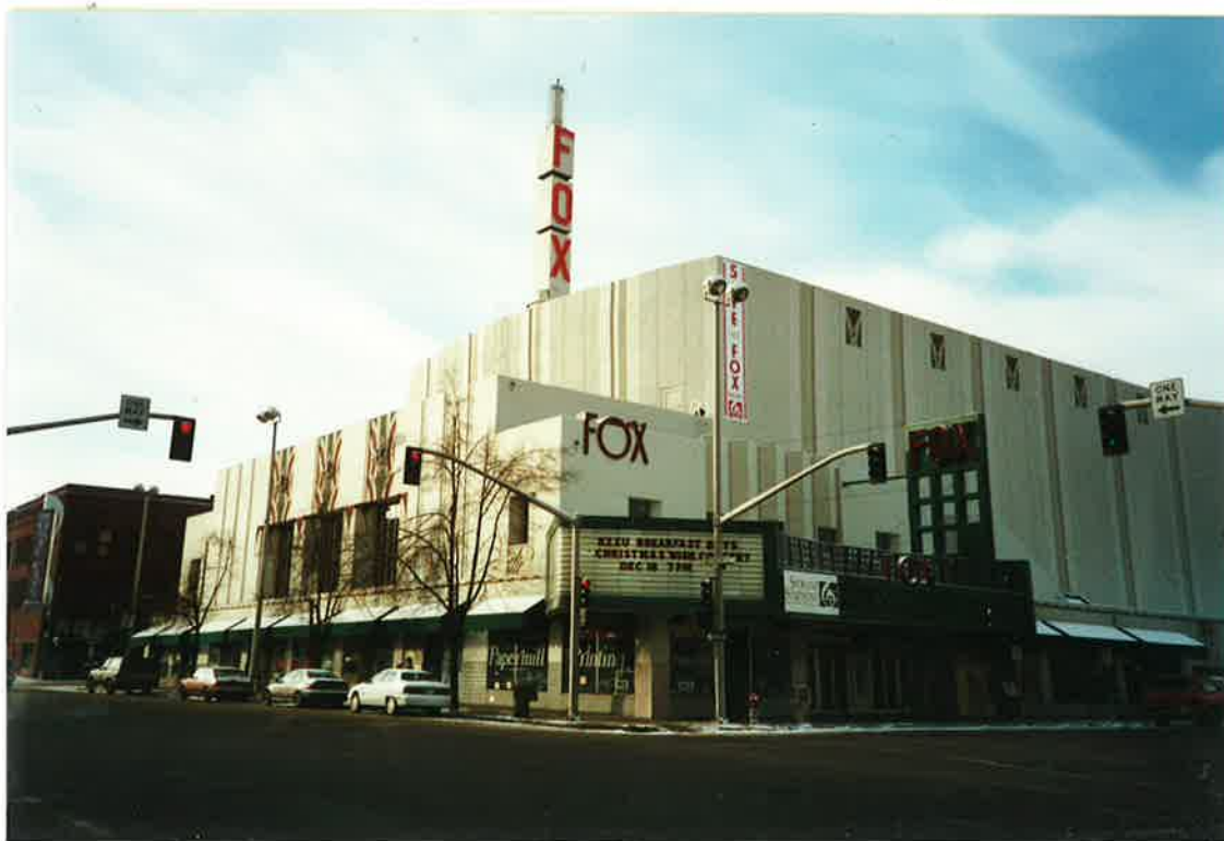
FOX THEATRE West Sprague Avenue (North elevation)
