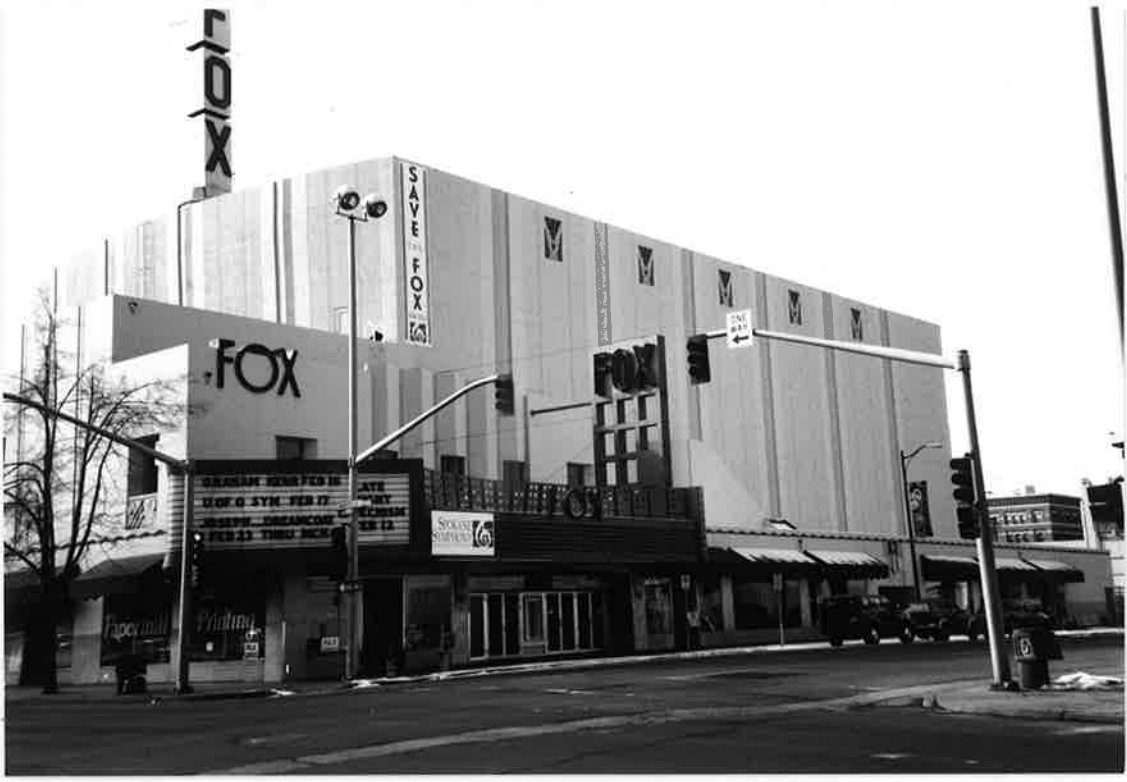
FOX THEATRE West Sprague Avenue North elevation
