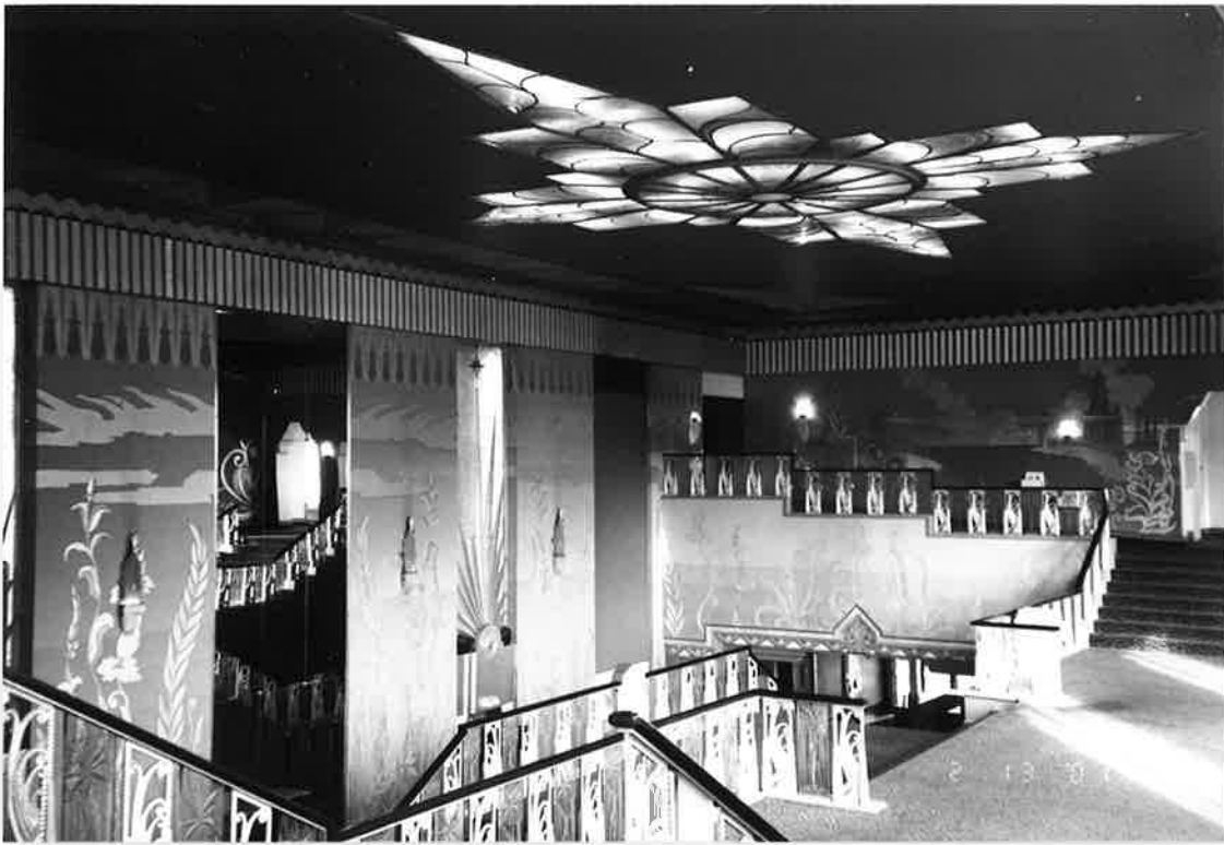
FOX THEATRE Lobby and mezzanine View to northwest
