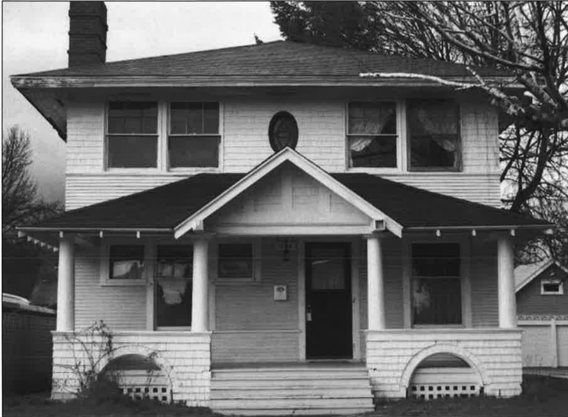
Front (south) façade
