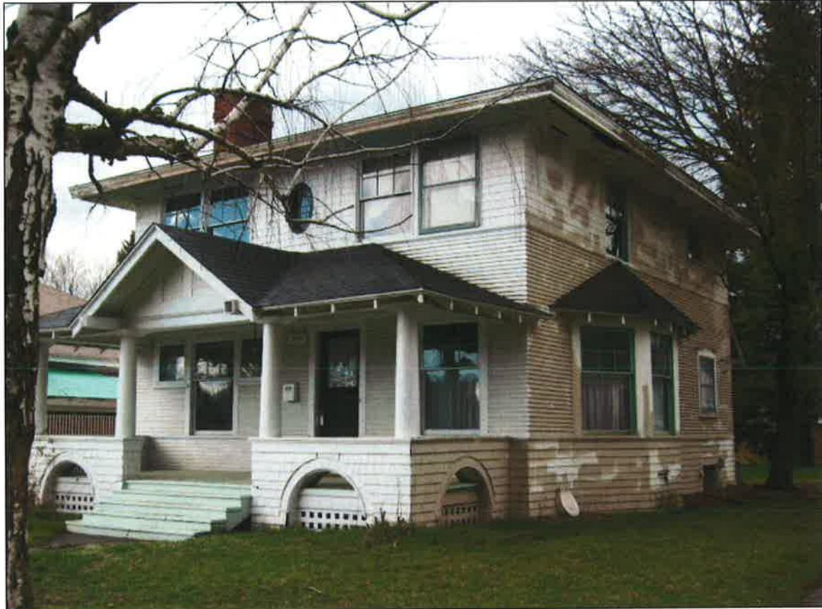
Front (south) and side (east) façade
