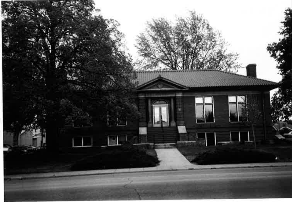
Photos 3 and 4 West façade of building, photos taken in 2004.
