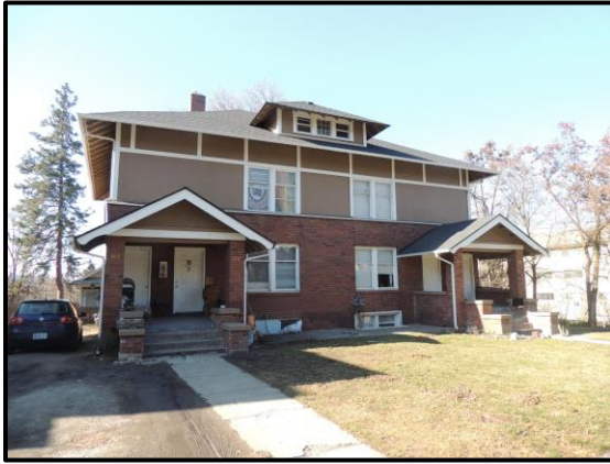
3. Double house converted to apartments at 606 South Cedar Street.
